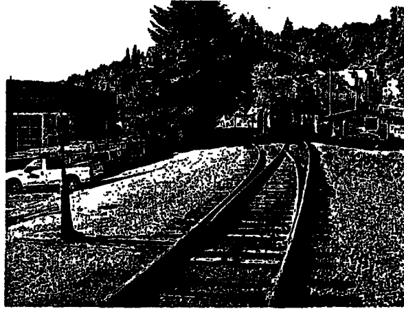
001 Issaquah(Redmond) Spur - Woodinville Junction Switch
