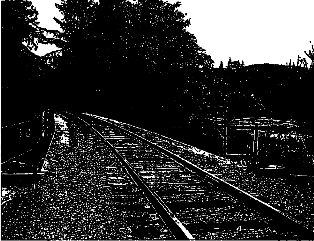
1. Looking Toward Increasing Milepost
