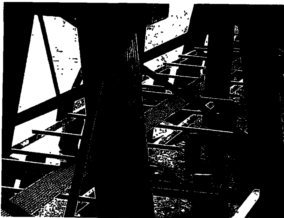
7. Walkway Under Bridge
