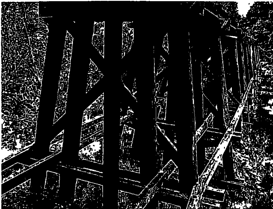
7. Looking Ahead From Under Bridge
