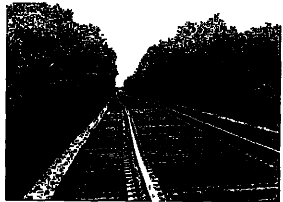
Bridge 29 2 Photo 4 Note lateral shift in track structure due to bridge shifting.
