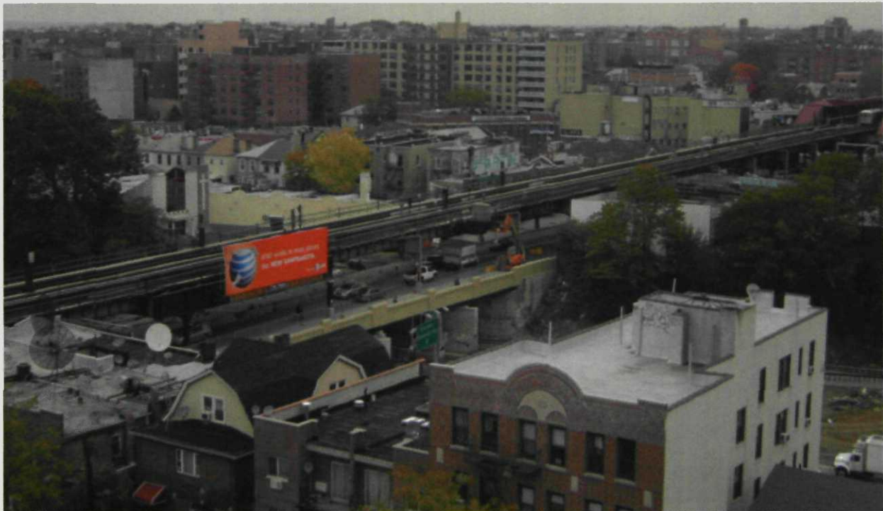
Photo # 2 Rooftop Photo of Roosevelt Avenue Overpass from Vitale-Owned Apartment Building Note Bridge Opening in Center of Photo (looking east)
