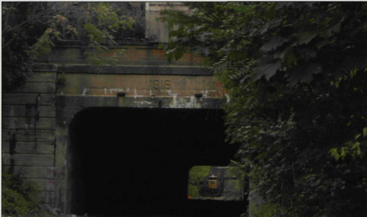
Photo # 4 Metropolitan Avenue Overpass (approximately 500 Feet Long) (looking north)
