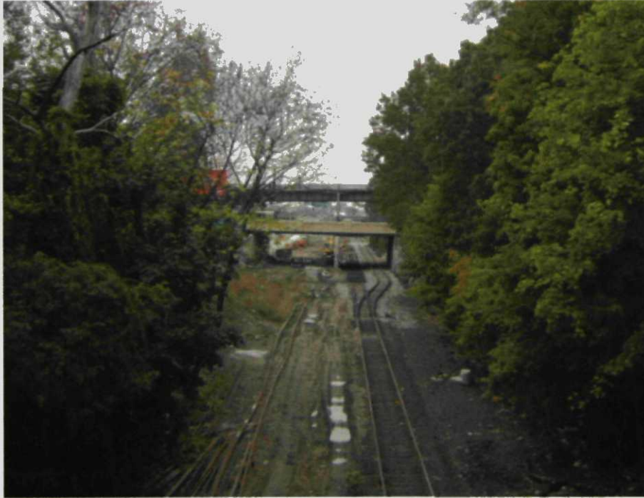
Photo # 1 Roosevelt Avenue Overpass from 41 st Street Overpass Note Temporary Track (Shoofly) to the East of Main Track (looking north)
