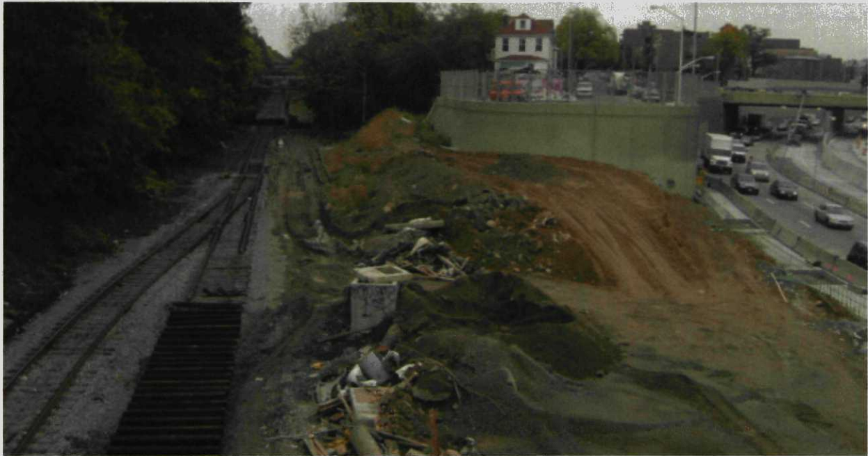
Photo # 3 Brooklyn-Queens Expressway Construction Note Temporary Track (Shoofly) to the East of Main Track (look south)
