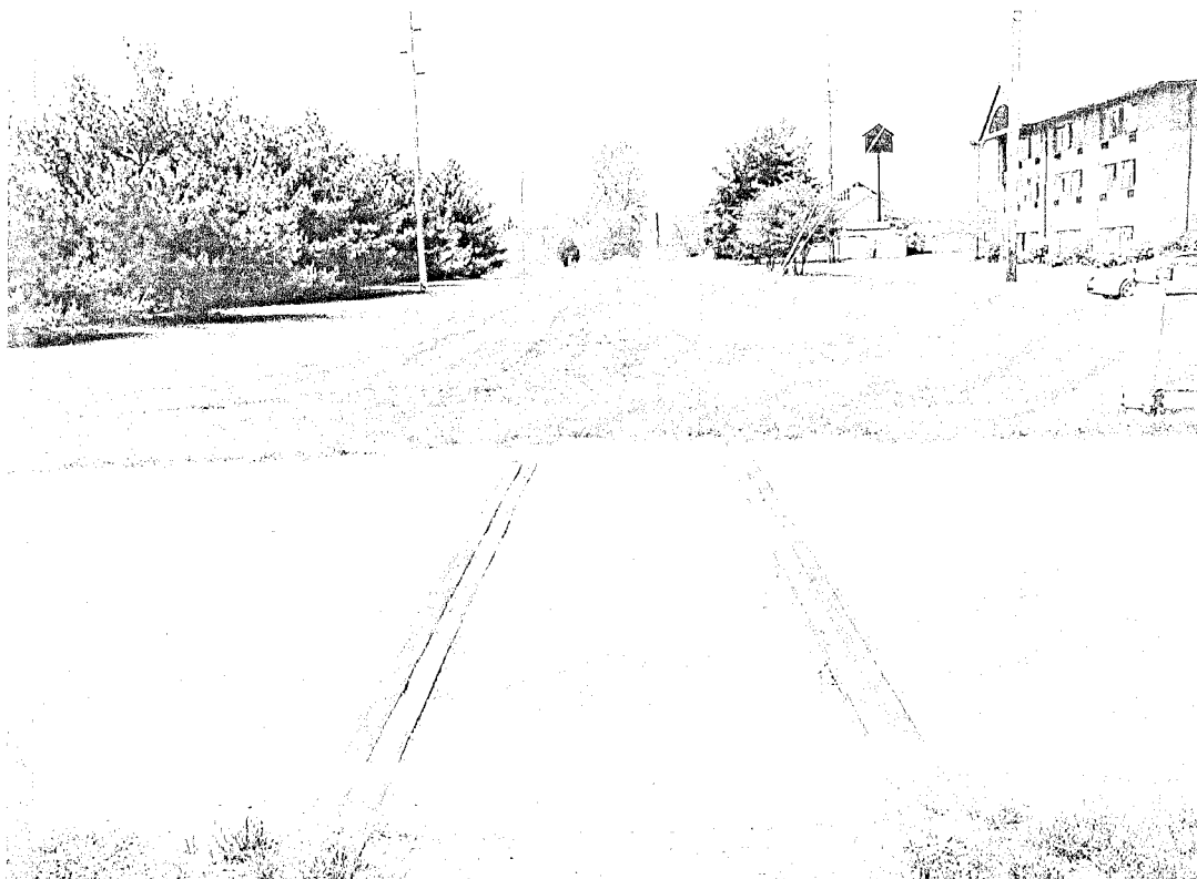
Figure 1 Douglas Rd. extension looking north to Toll Road, note rails still in crossing
