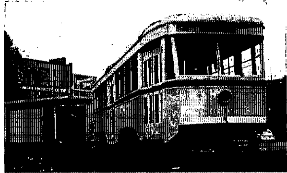
No. 6119 arrives at its new home, the just-completed BSM carhouse.
