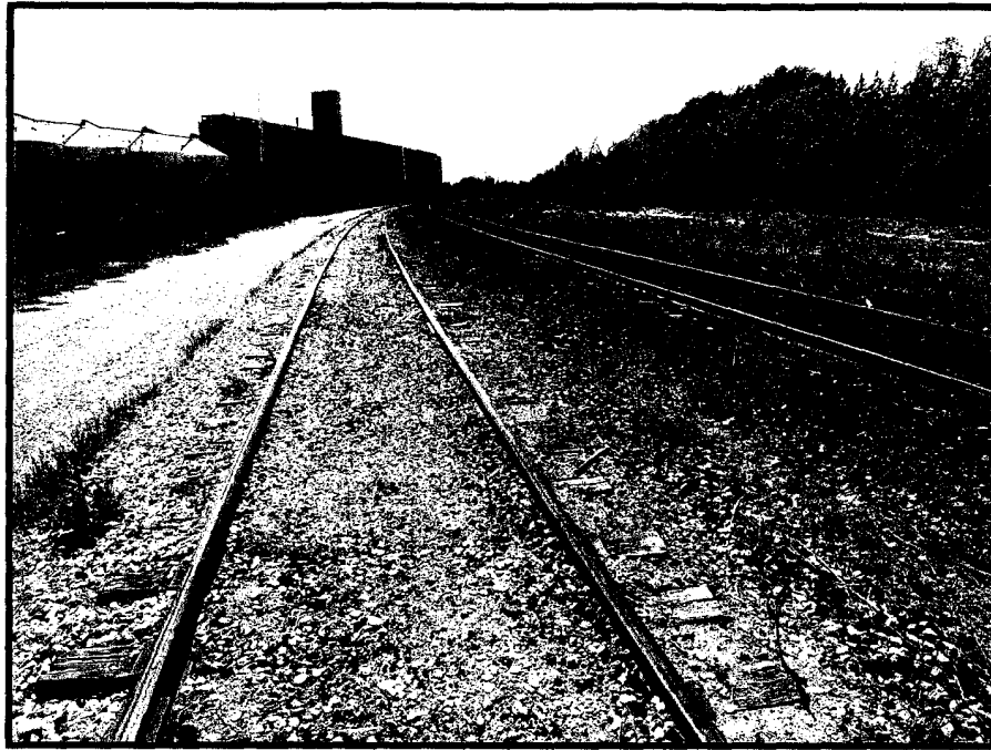
This section of the trackage is referred to as Track 9200 just north of 37 th Street west of Guava Avenue.
