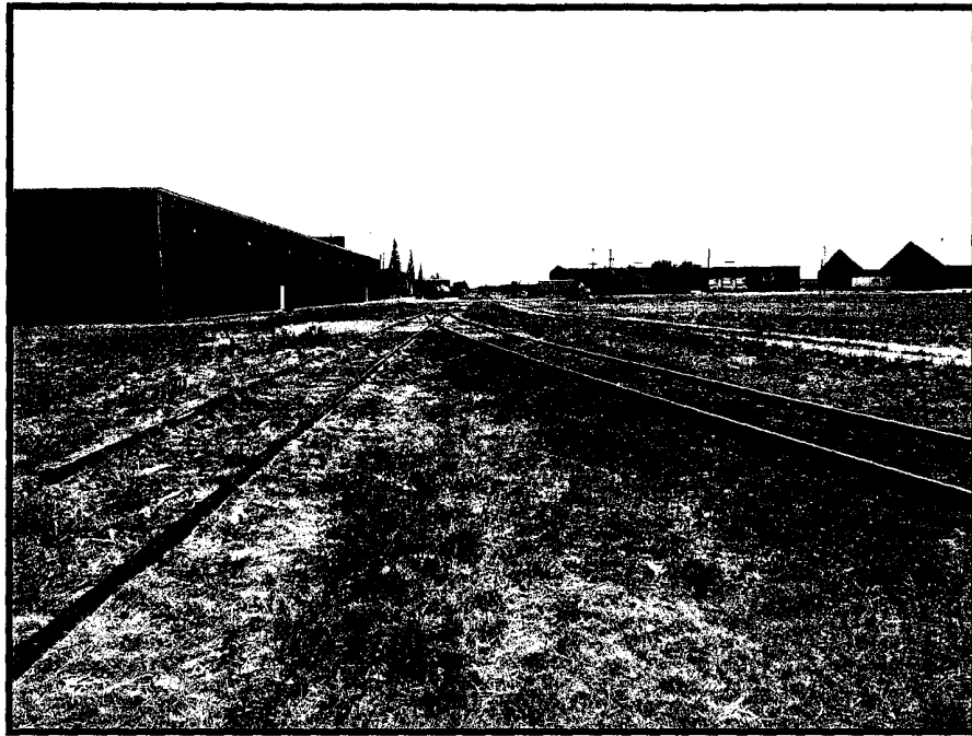
This rail track spur is in the Burlington Industrial District area as we look south from 40 th Street just west of Locust Avenue.
