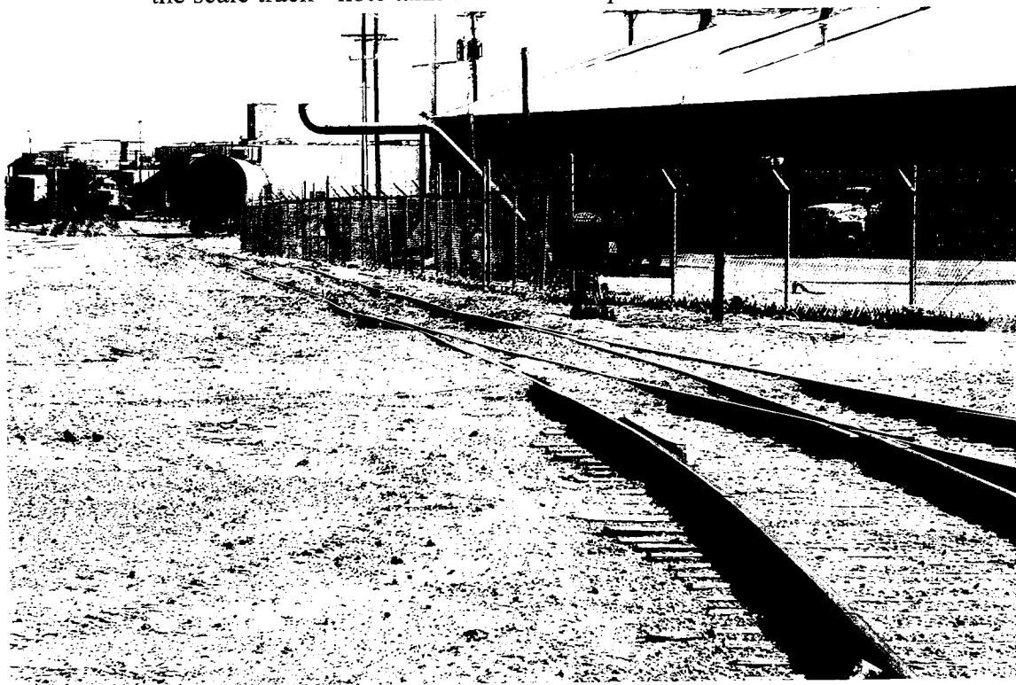
Photograph 6 - termination of the shop track on right side of photo - shop track accommodates 13 standard-length cars.
