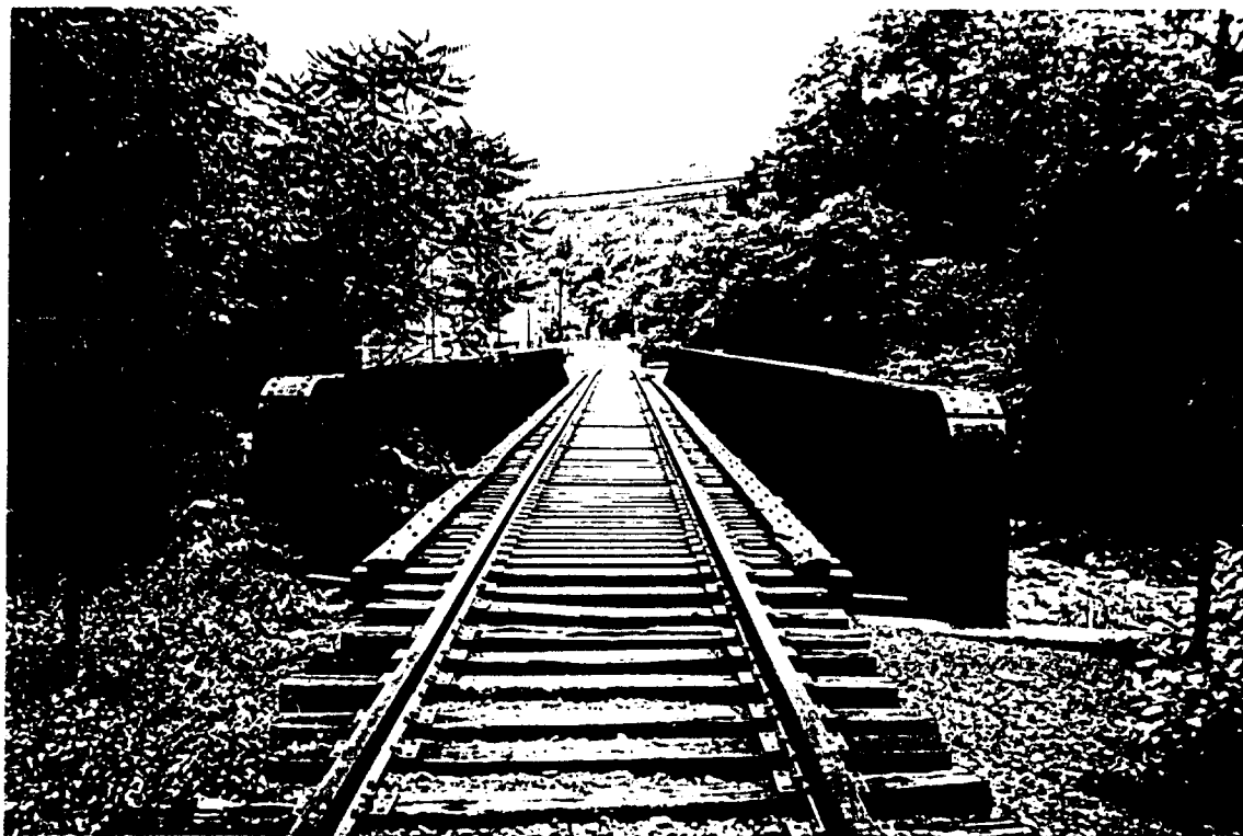
Bridge 2540 Looking East
