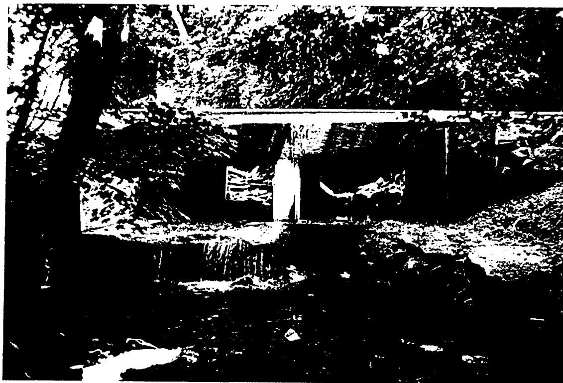
Bridge 2310 South Face
