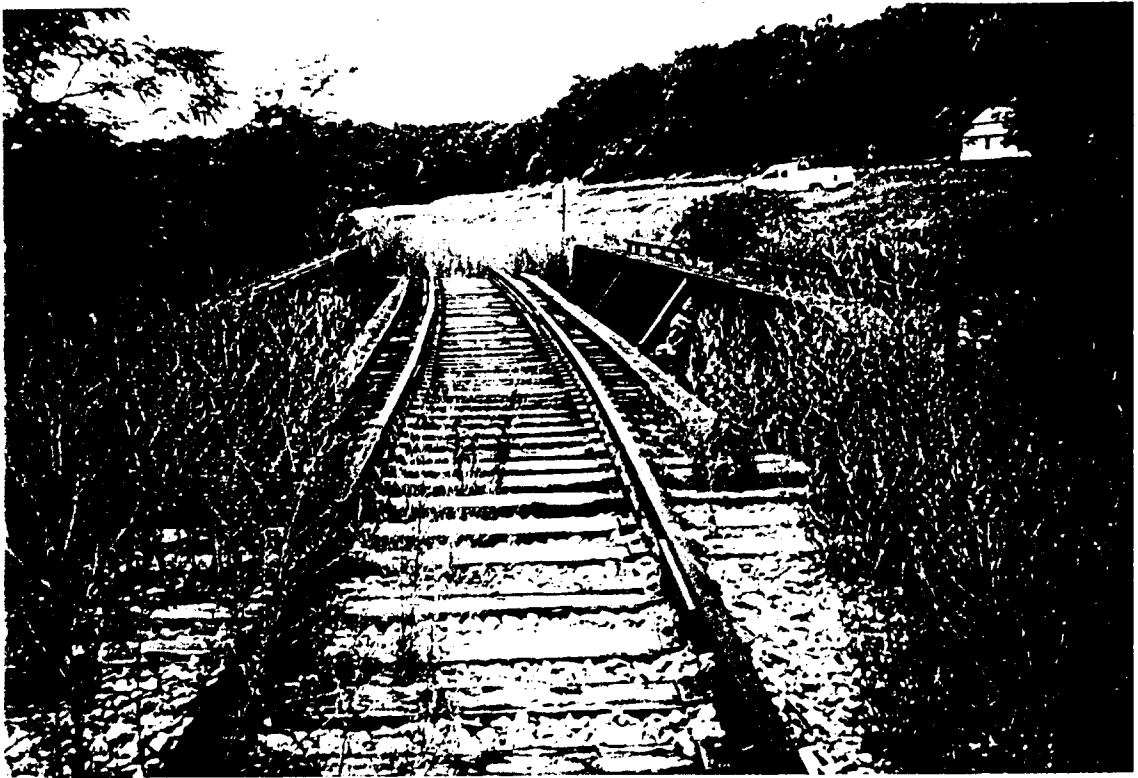
Bridge 2019 Looking West
