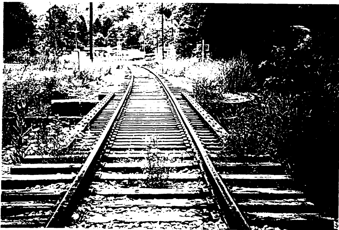
Bridge 2261 Looking East
