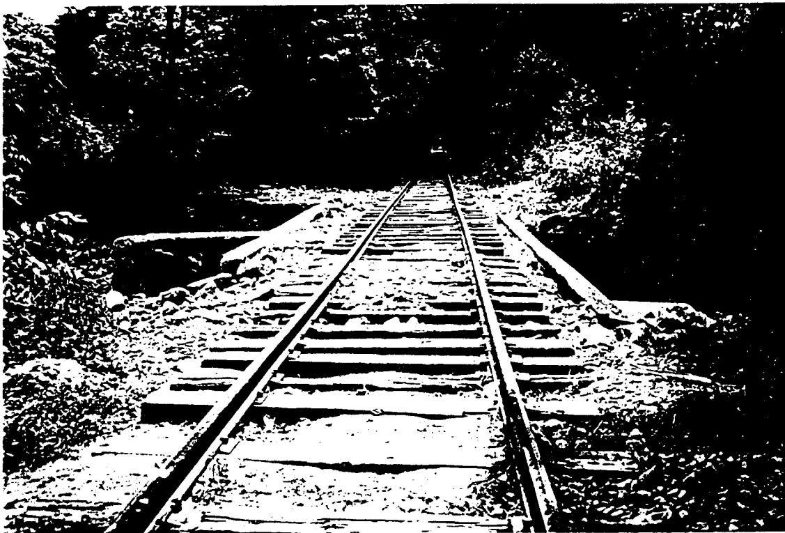
Bridge 2130 Looking East
