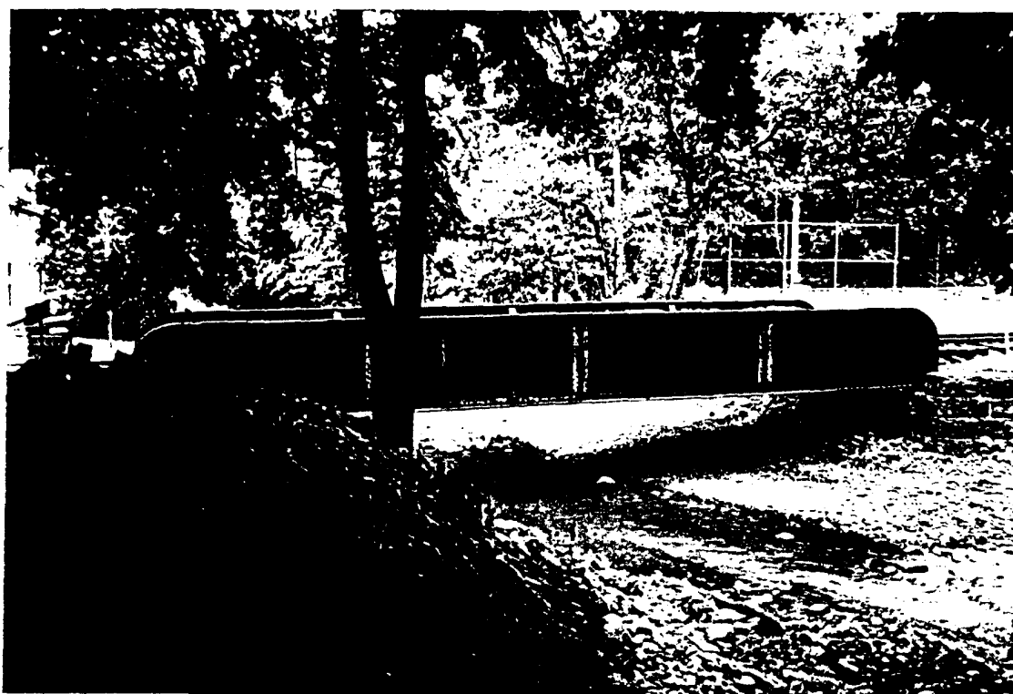
Bridge 2064 North Face
