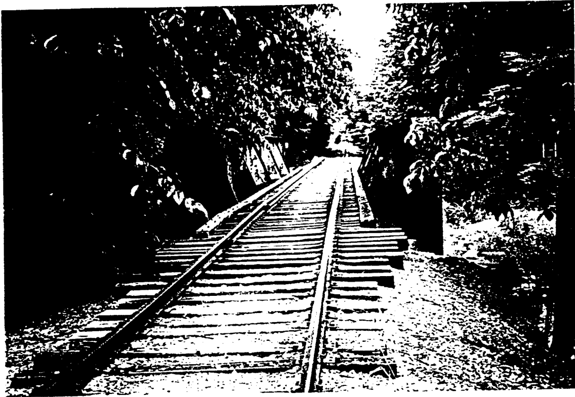
Bridge 2158 Looking West
