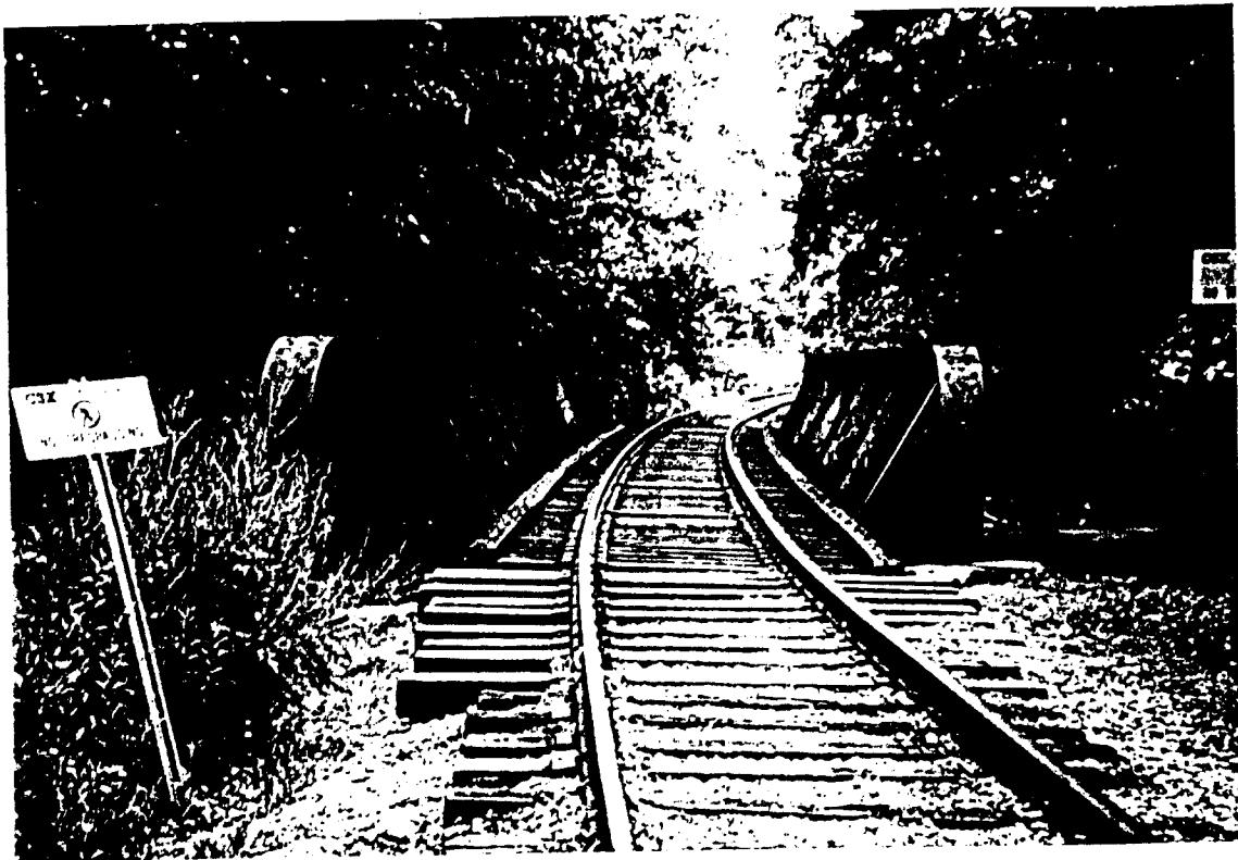
Bridge 2246 Looking West
