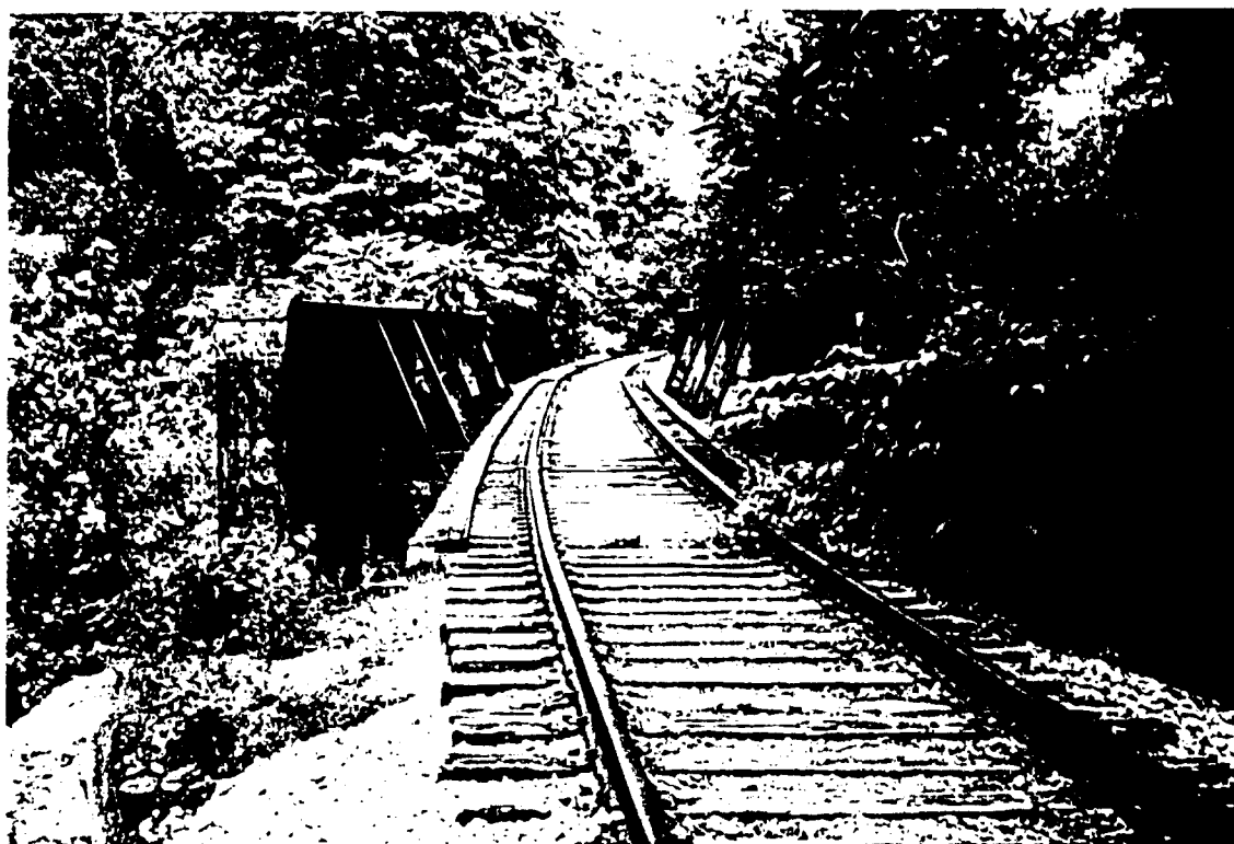
Bridge 2675 Looking West
