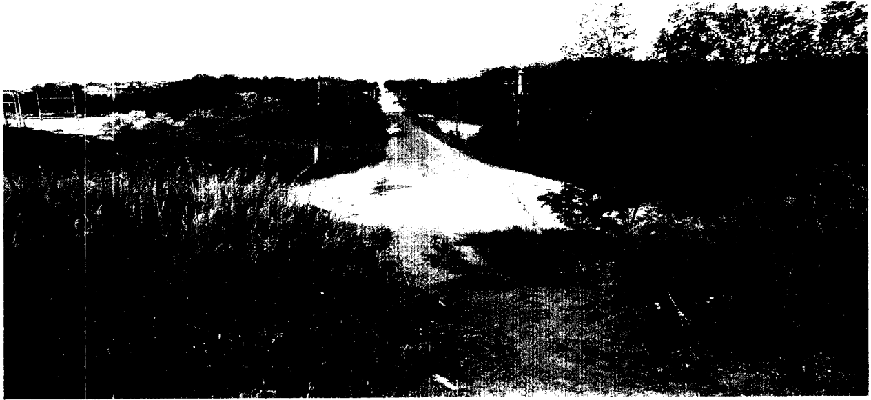
View from top of bridge looking west
