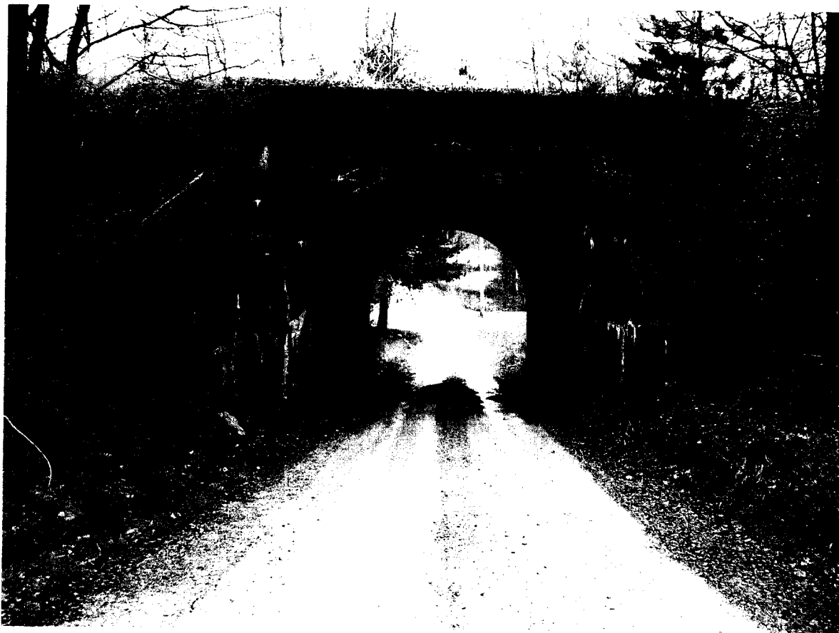
Arch 15' MP 29.51 East
