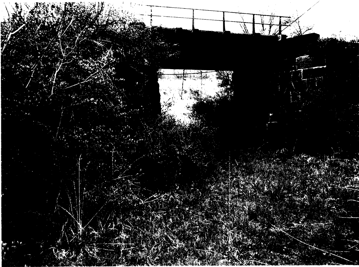
Bridge No. 41.27 East
