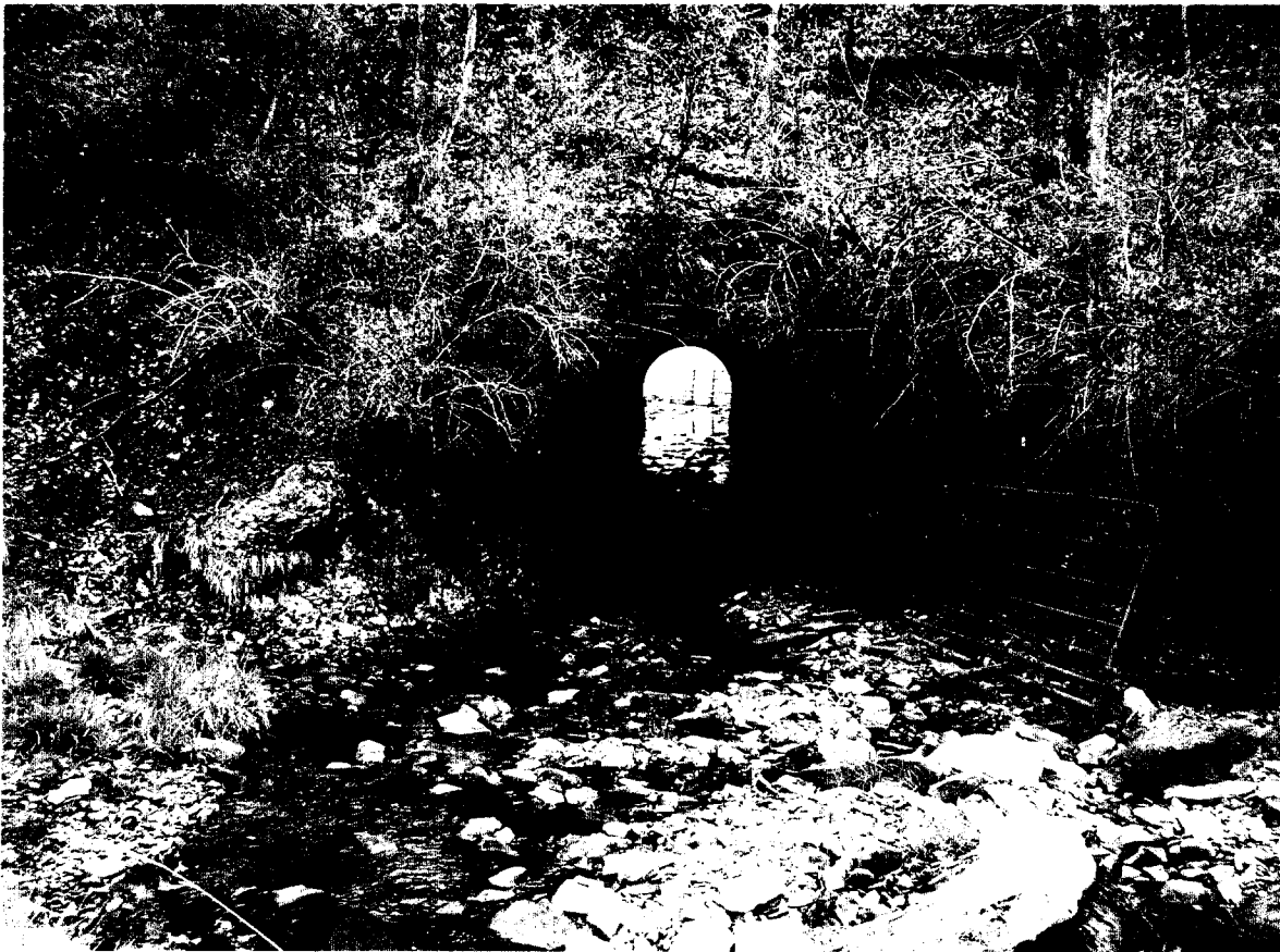
Arch 8' MP 43.16 West
