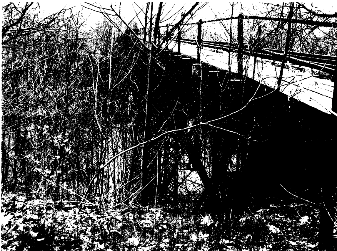
Bridge No. MP 55.43 South End West Side looking North
