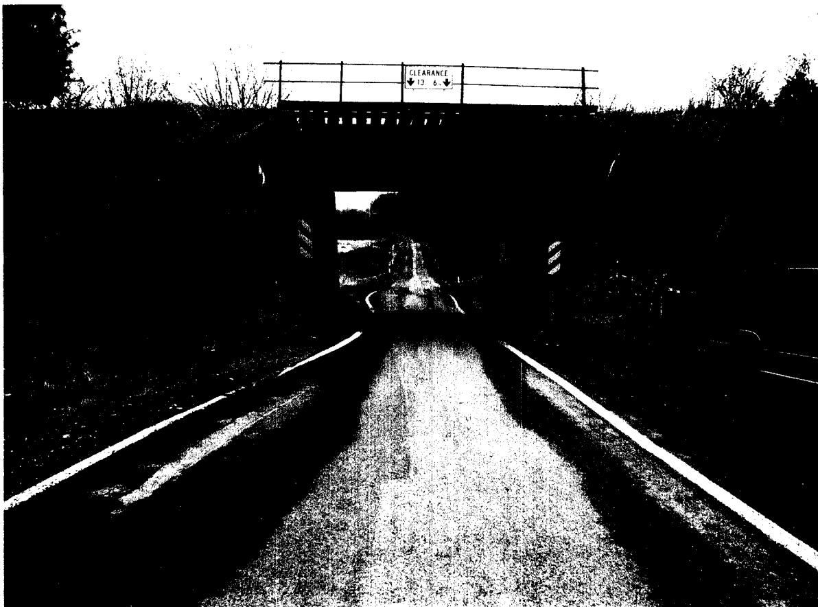
Bridge No. 42.34 East
