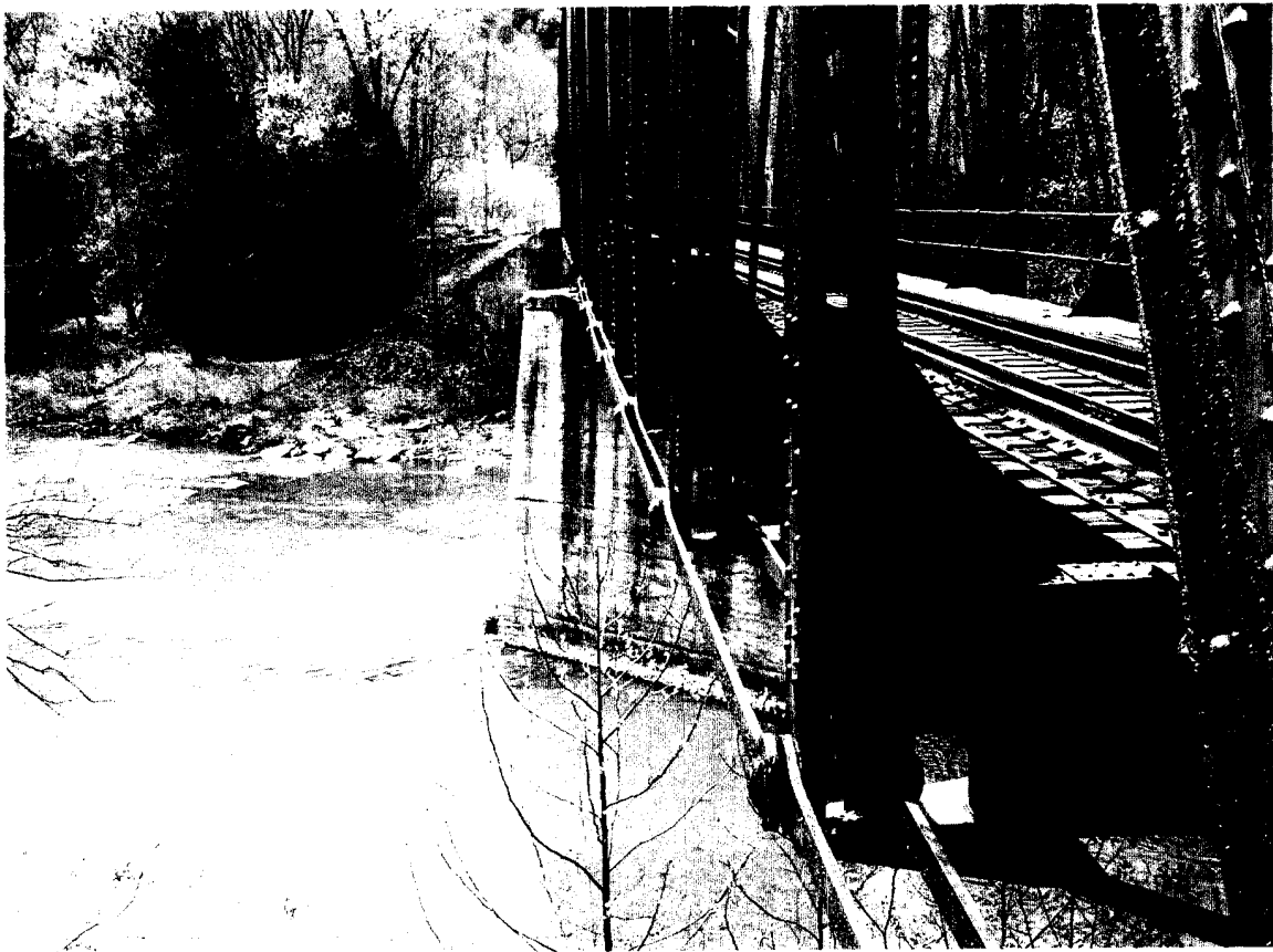
Bridge No. MP 57.81 East
