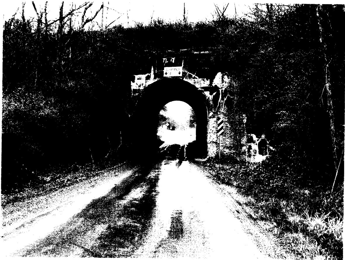
Arch 16' MP 28.02 East
