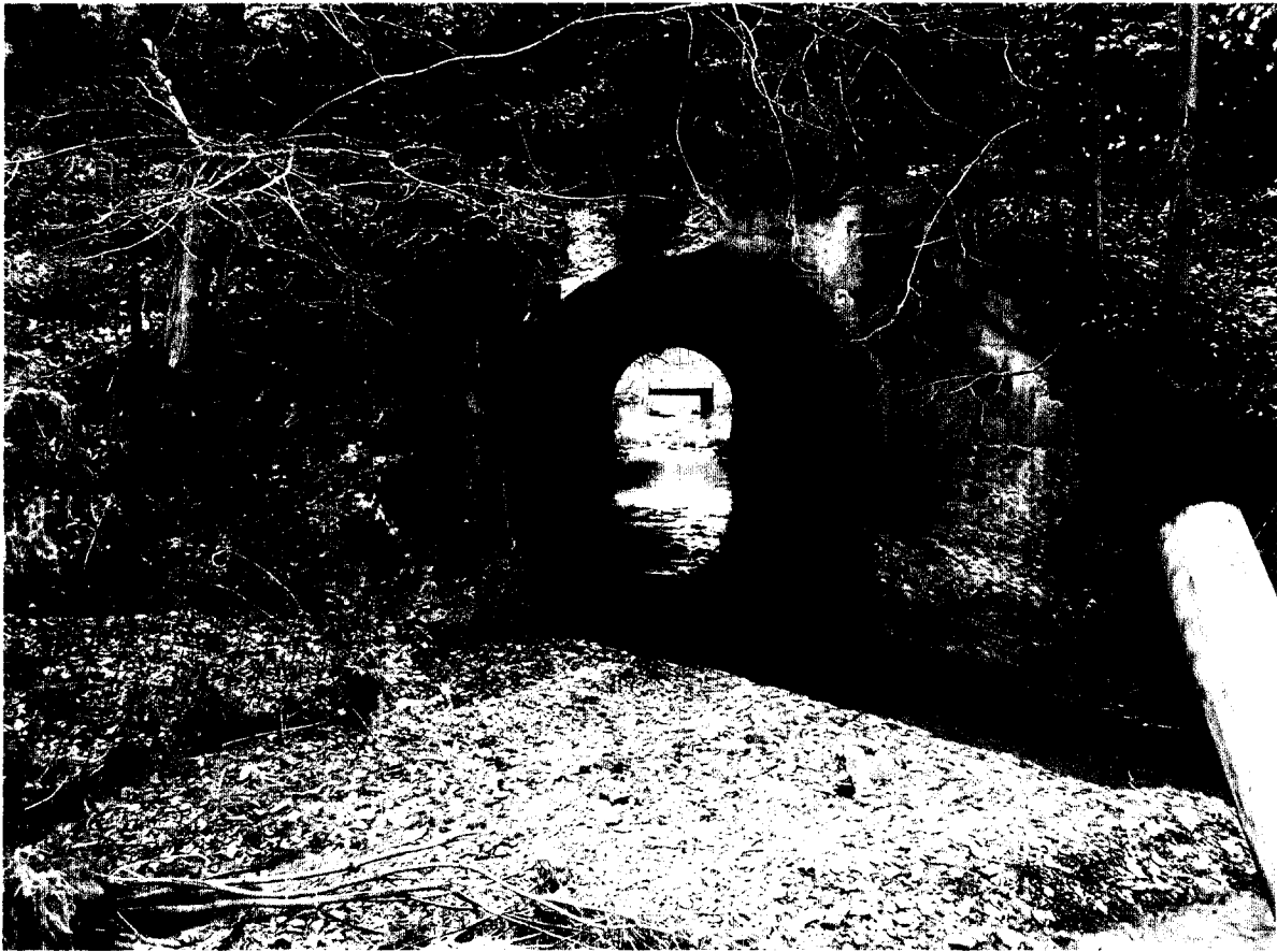
Arch 12' MP 42.86 West
