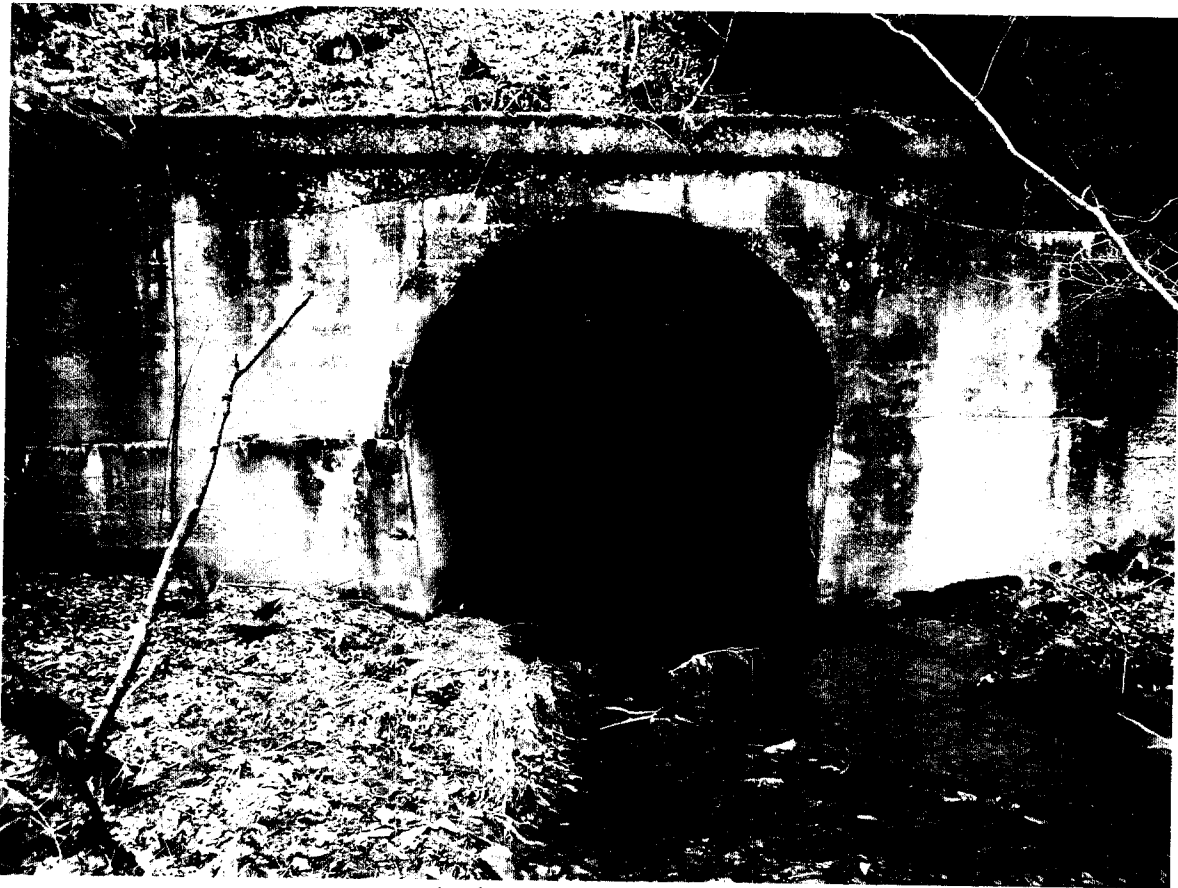
Arch 10' MP 47.92 East
