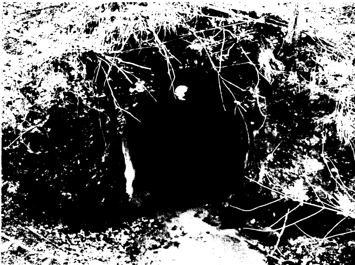
Arch 16' MP 42.39 West
