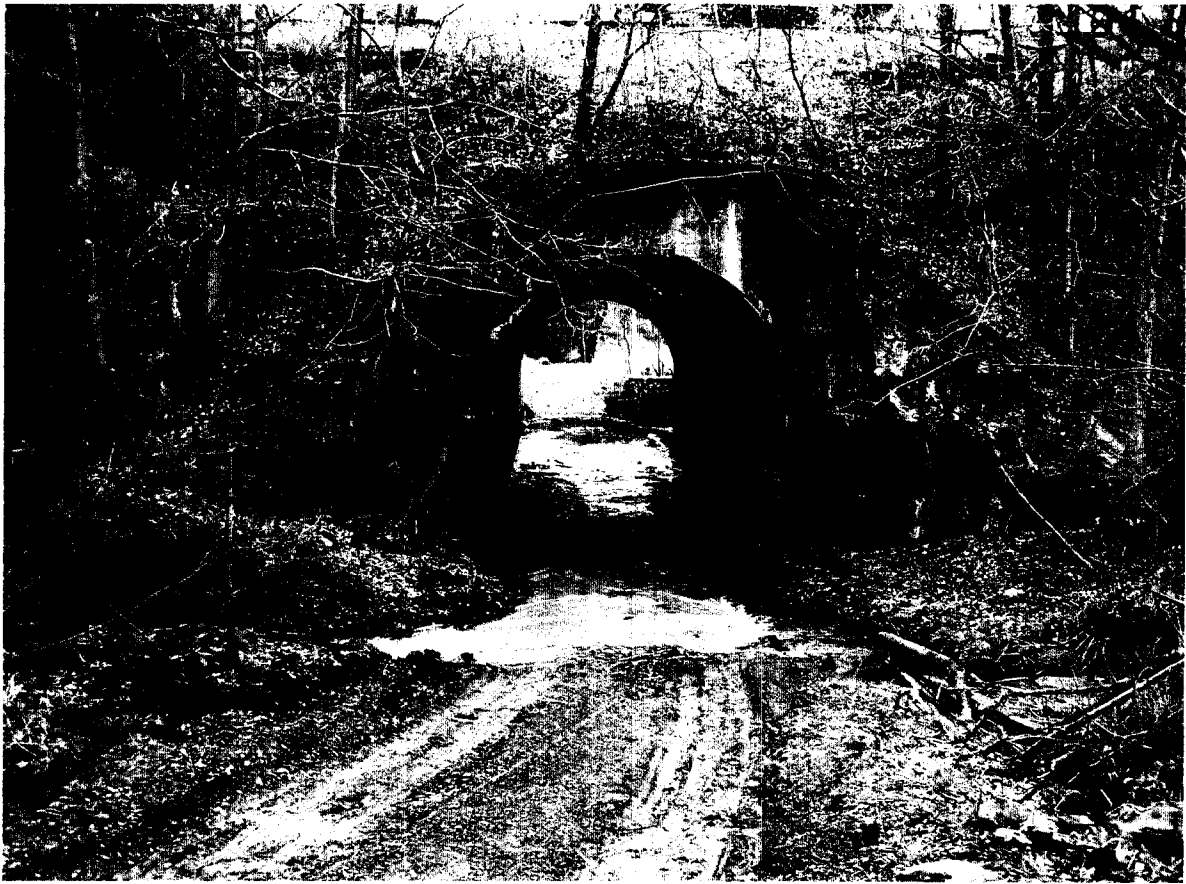
Arch 15' MP 43.59 West
