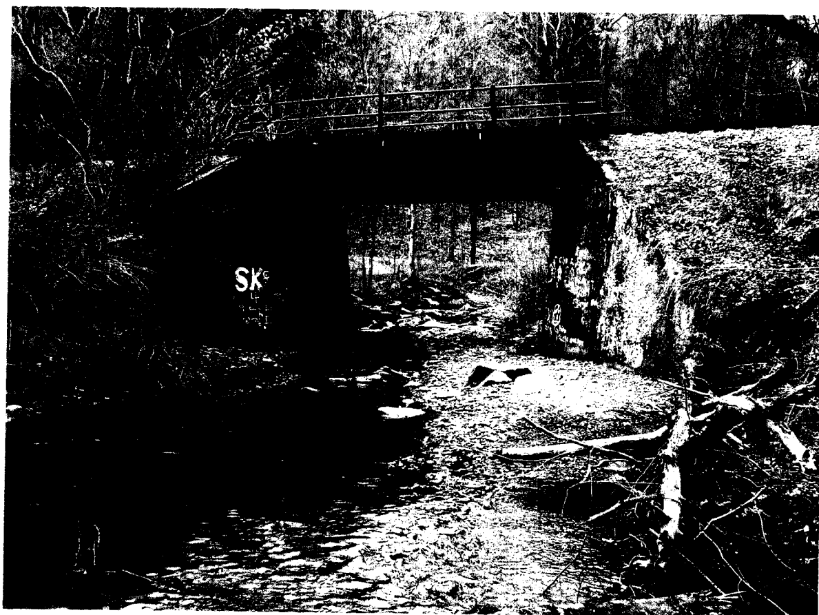
Bridge No. MP 59.21 East
