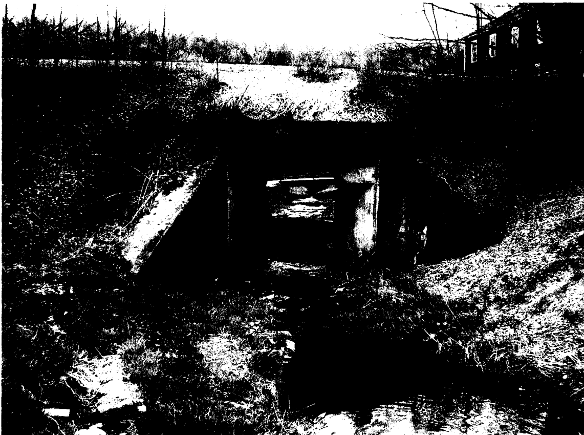
Arch 15' MP 44.57 West
