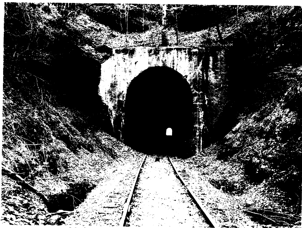
Mack Tunnel MP 56.73 South End looking North
