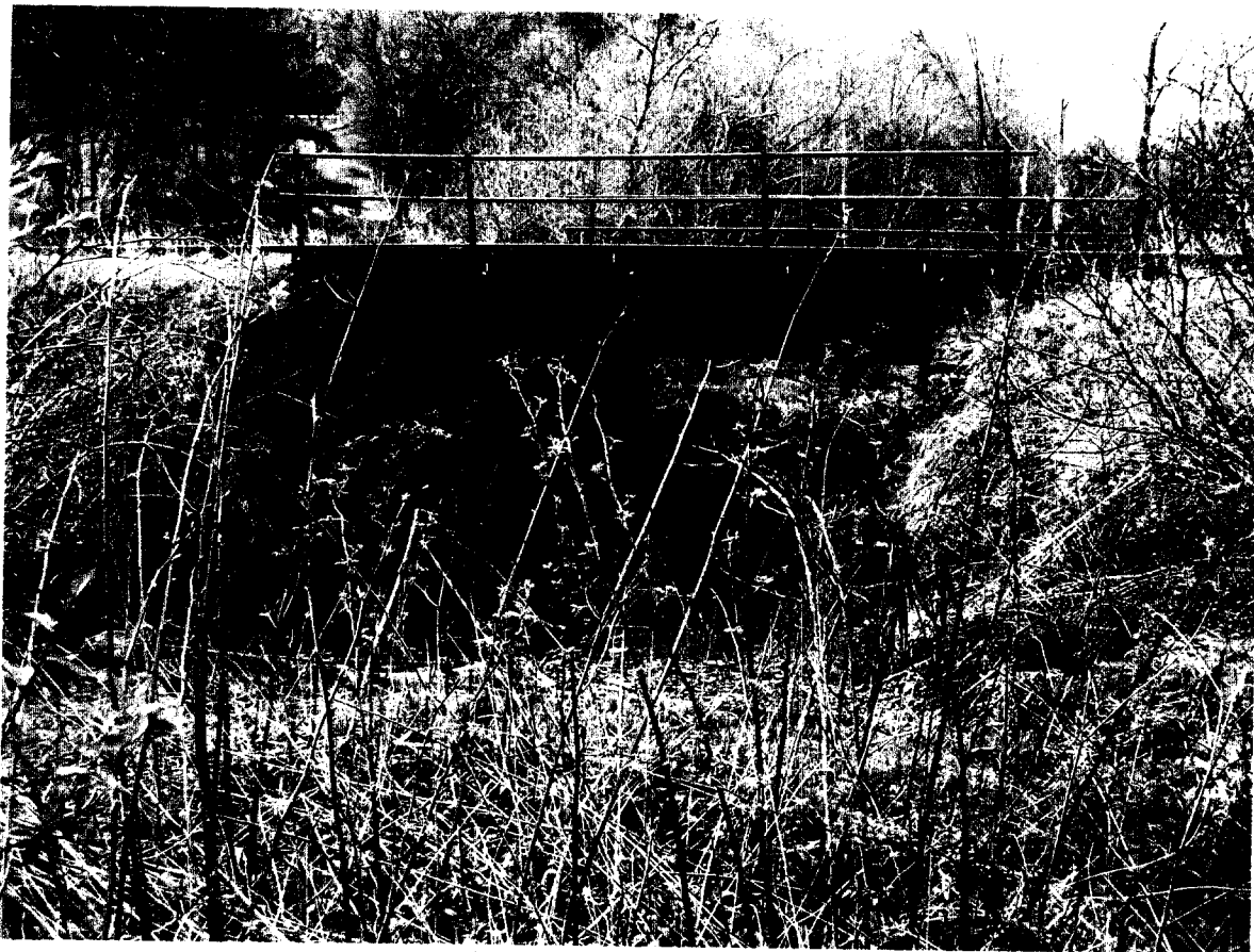
Bridge No. MP 45.95 West
