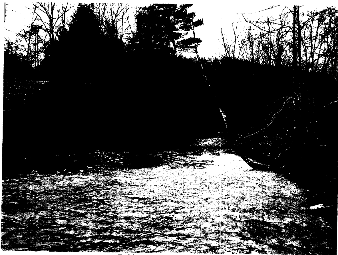
Bridge No. MP 46.32 West
