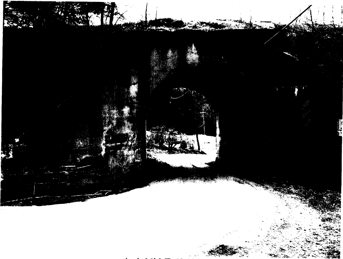
Arch 16' MP 48.92 West
