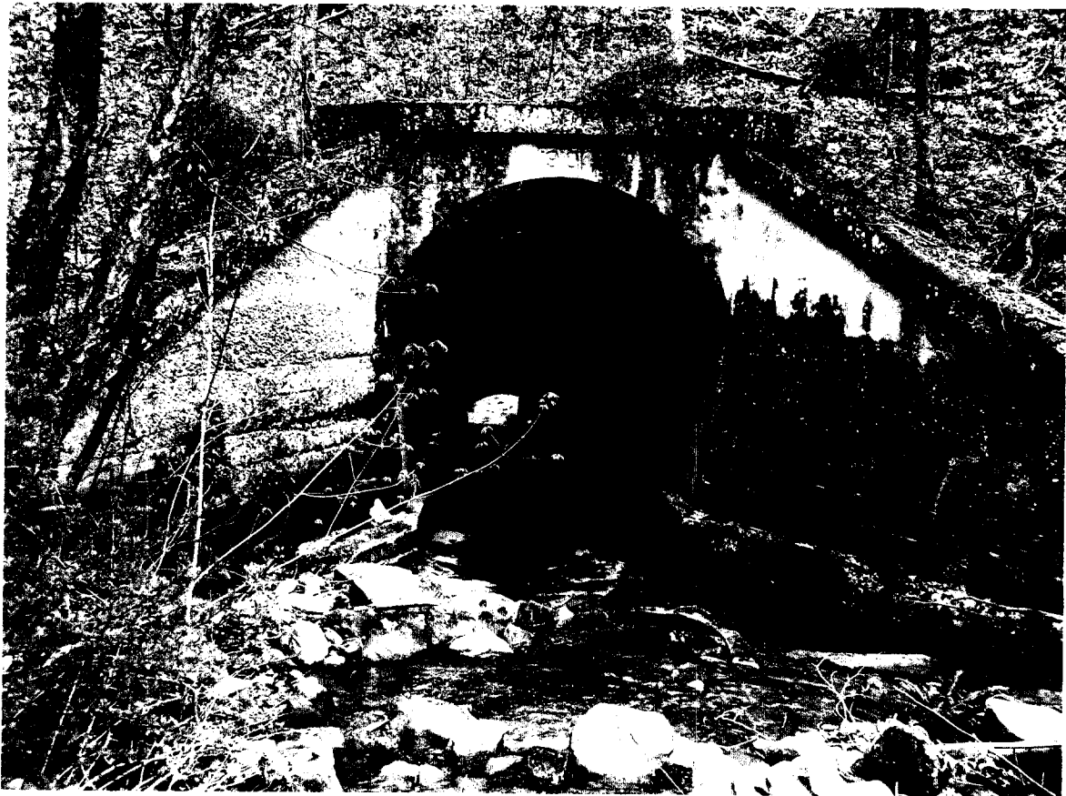
Arch 10' MP 52.69 West
