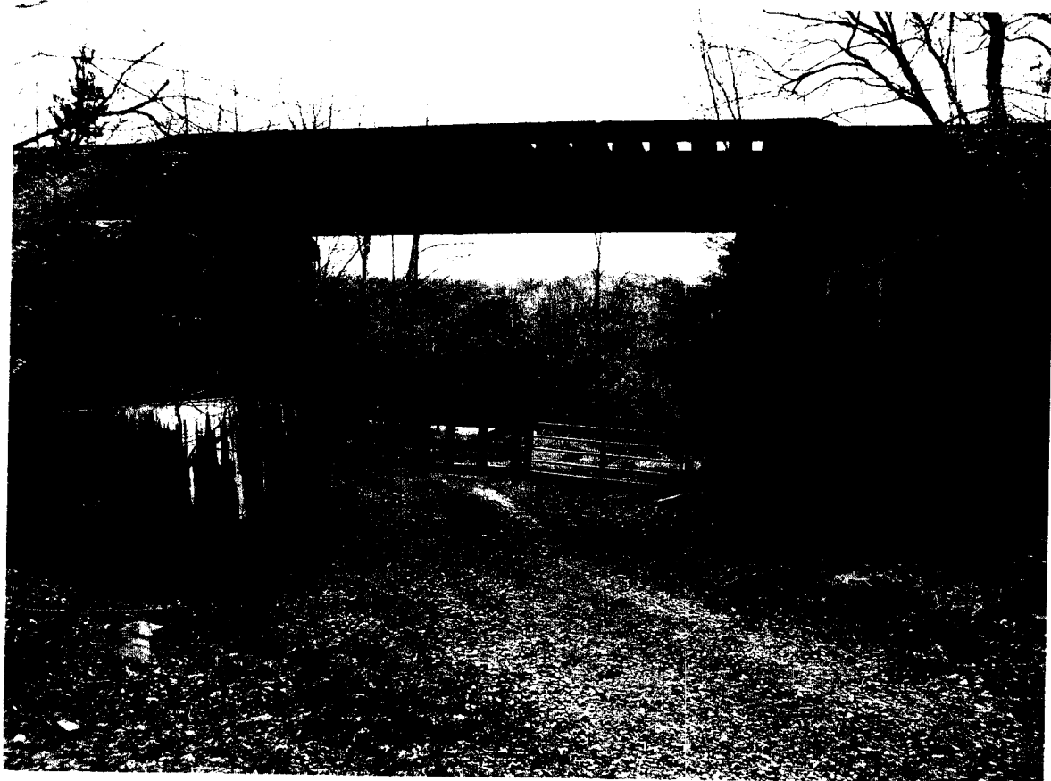
Bridge No. MP 49.06 West
