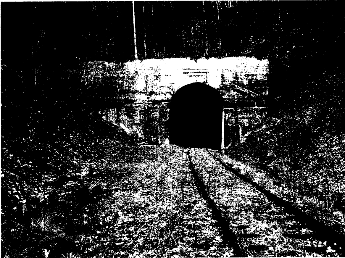
Coulter Tunnel South End looking North 35.73
