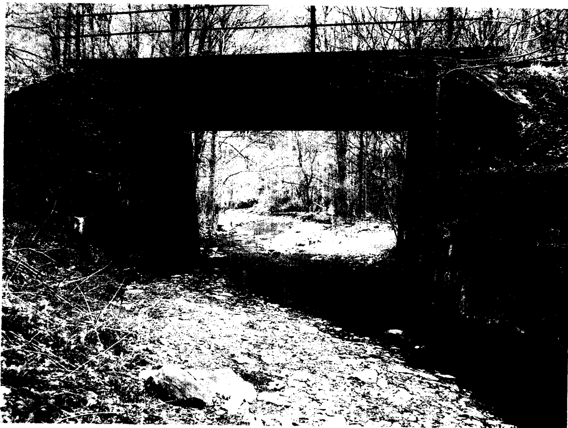
Bridge No. MP 58.46 West
