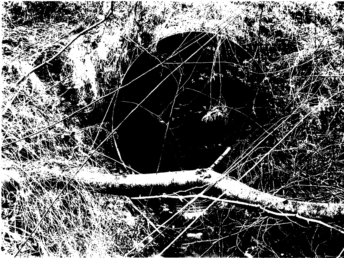
Arch 16' MP 42.39 East
