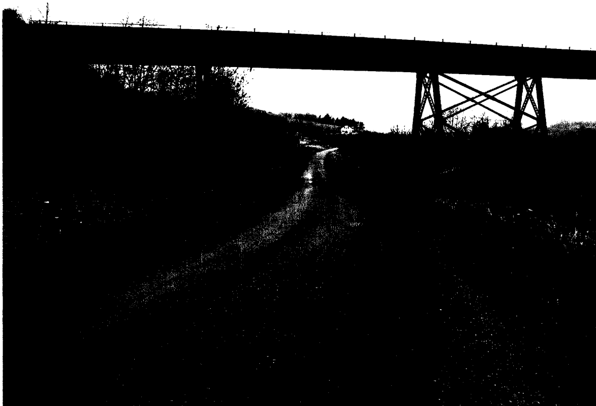
Bridge No. 38.4 East Side of South End
