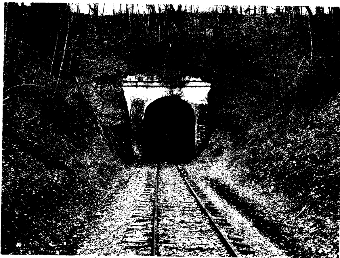
Mack Tunnel MP 56.73 North End looking South
