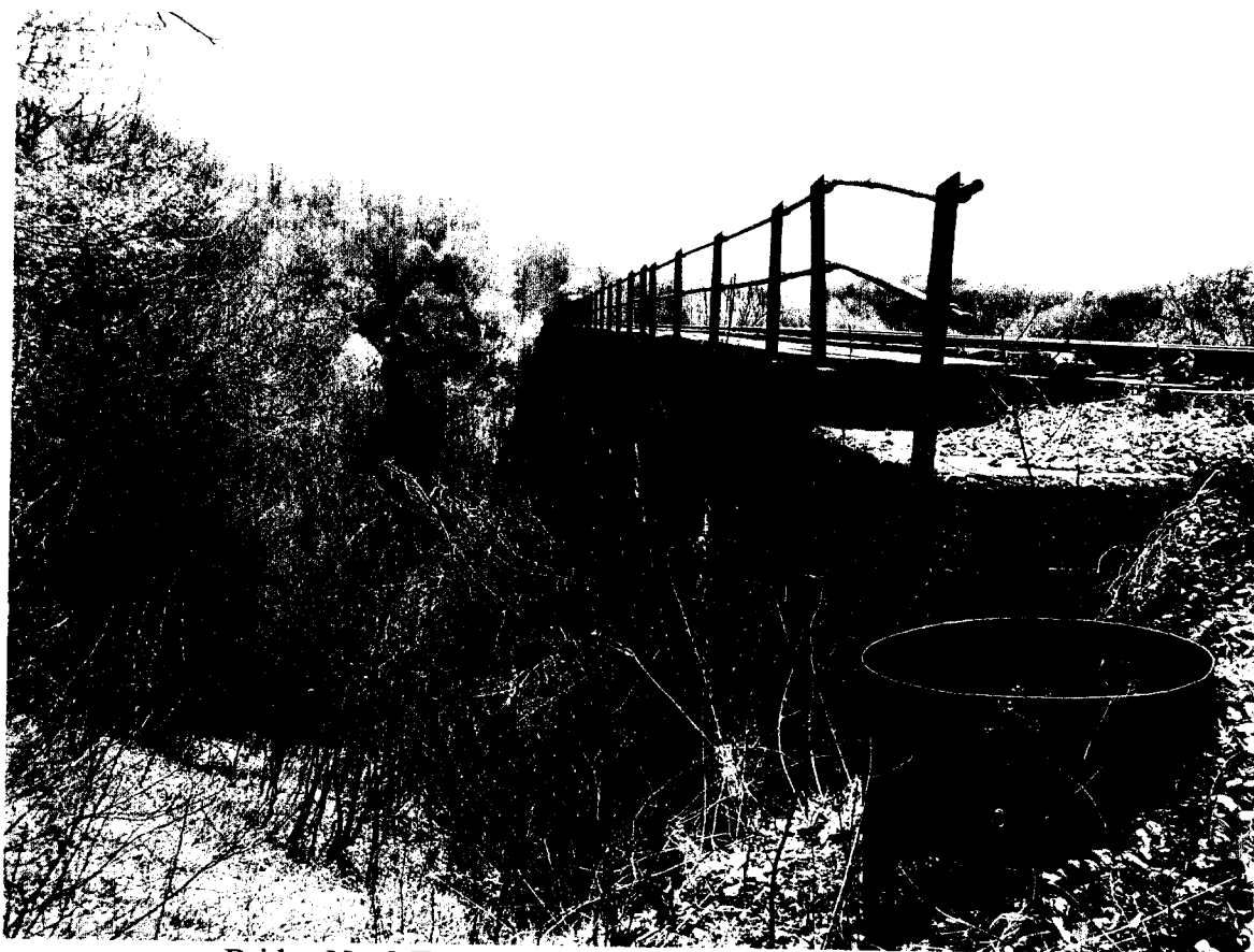
Bridge No. MP 51.23 South End West Side looking North
