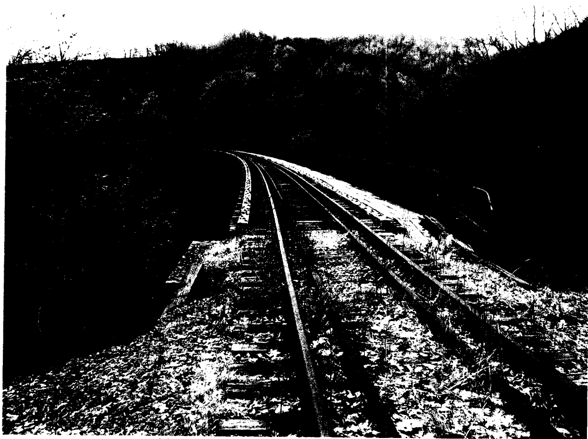
Bridge No. MP 51.86 North End looking South
