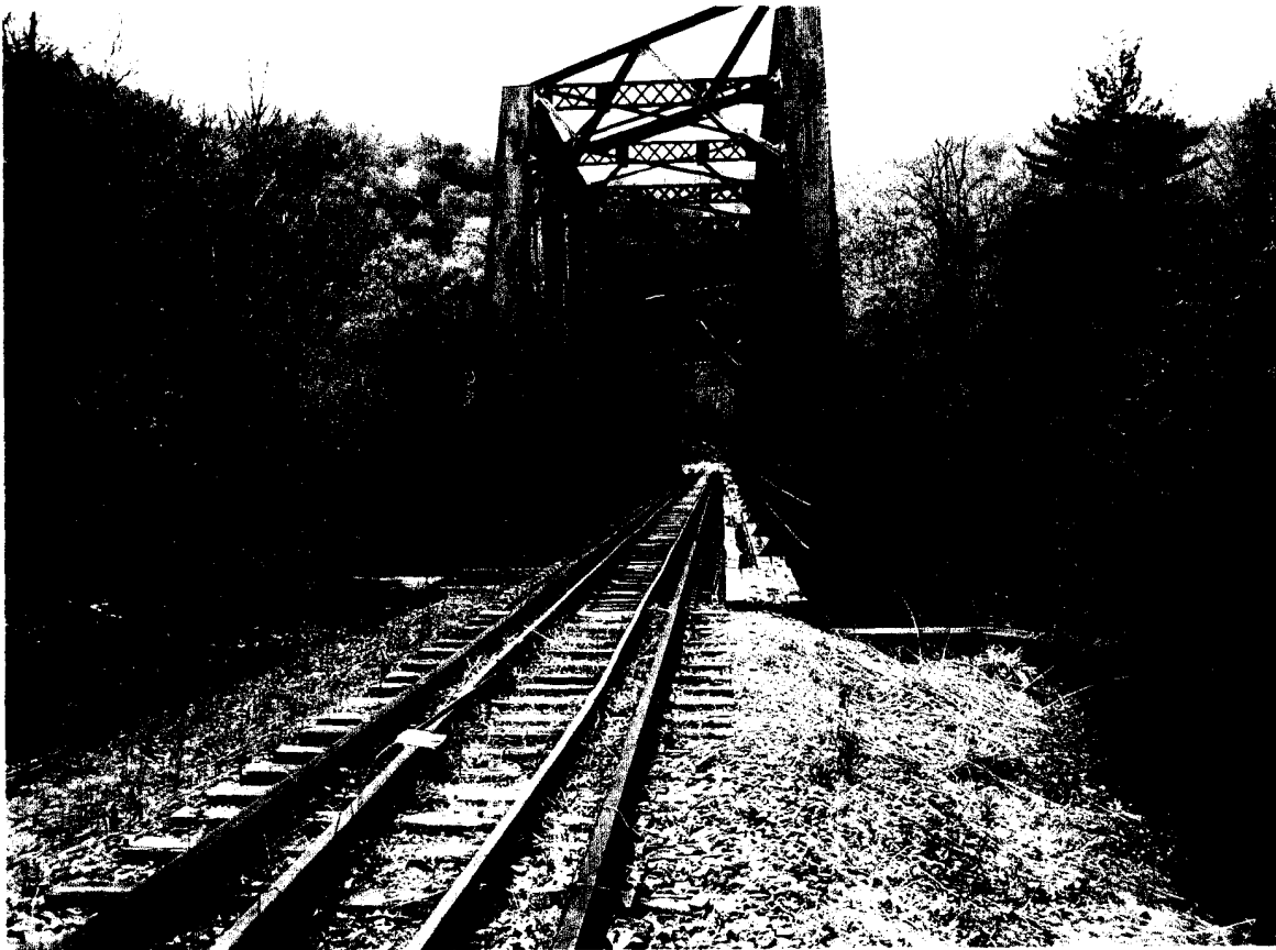
Bridge No. MP 57.81 South
