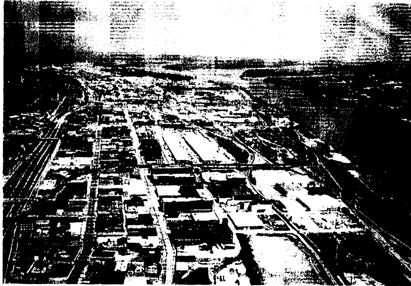
RSM overhead I-70 overpass to NS interchange
