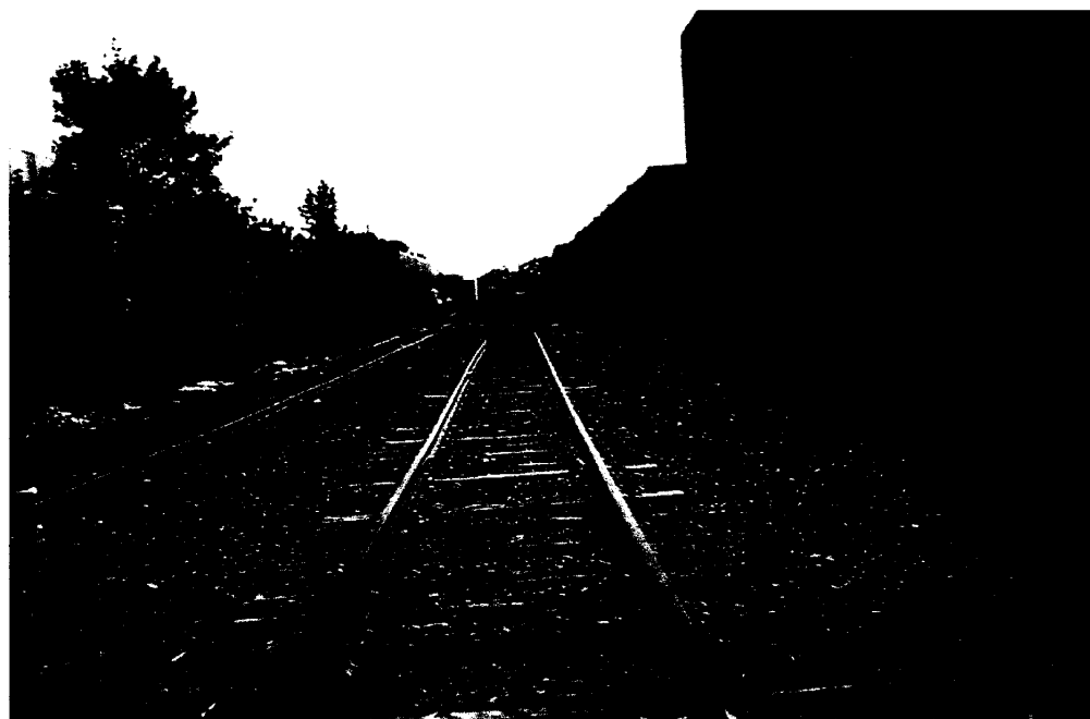
Sidings at 20 Executive Ave. before switch intallation Heller Park 8-15-04
