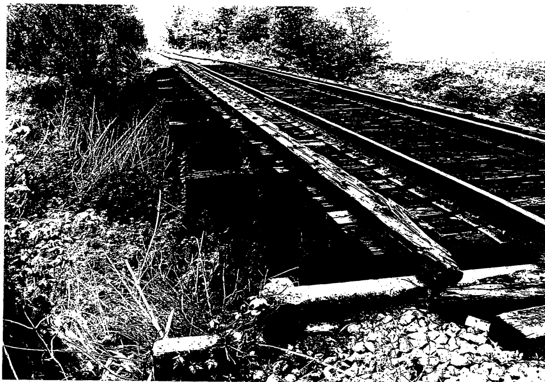
Trestle at MP 447.7 second view
