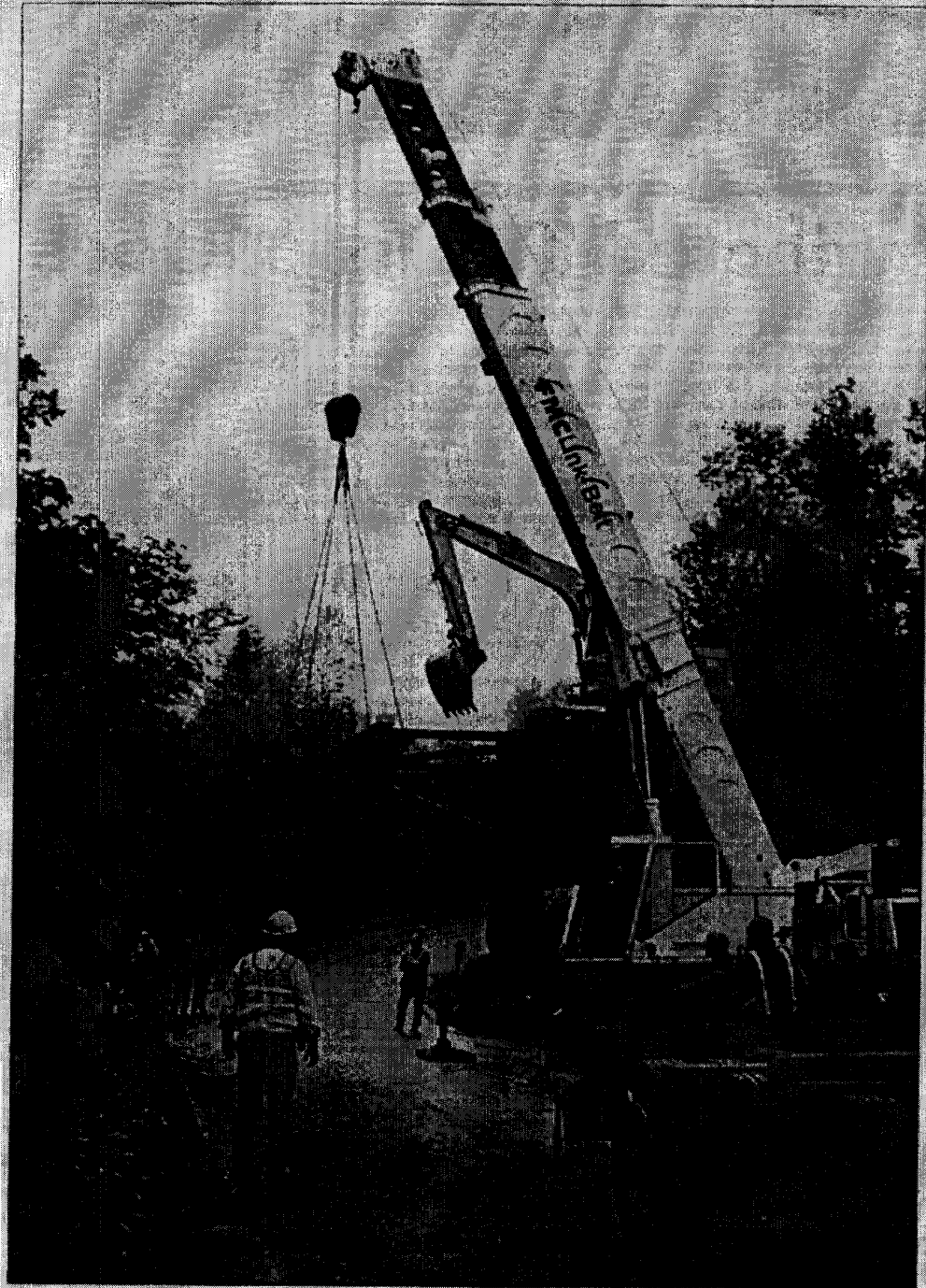
Horses and trains built the Walden overpass 82 years ago, but it took a crane to remove the railroad bridge last week. Construction to widen the overpass and improve visibility continues this week with removal of the concrete abutments and making a wider road. Transportation officials expect the work to be completed by the end of the month. (photo by Kristine Mercier)
