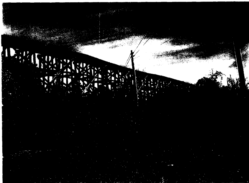
Wood trestle east of Ill Rte 3
