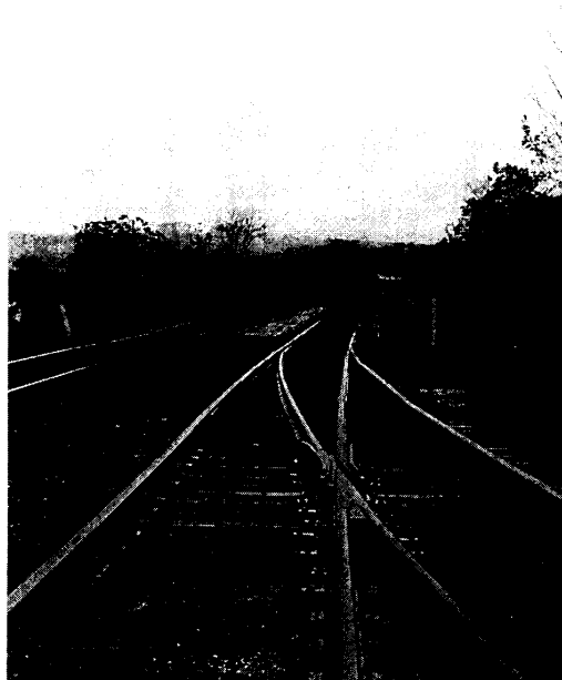
Track north from CSXT exchange
