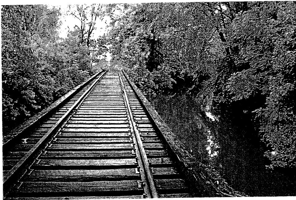
Photo E: Bridge over River Raisin (approx. MP 46.1) looking SW.
