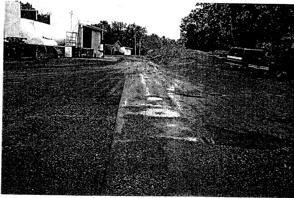
Photo A: College Ave. and TBCR ROW (approx. MP 46.3) looking SSW from Cutler Dickinson Co. parking lot.
