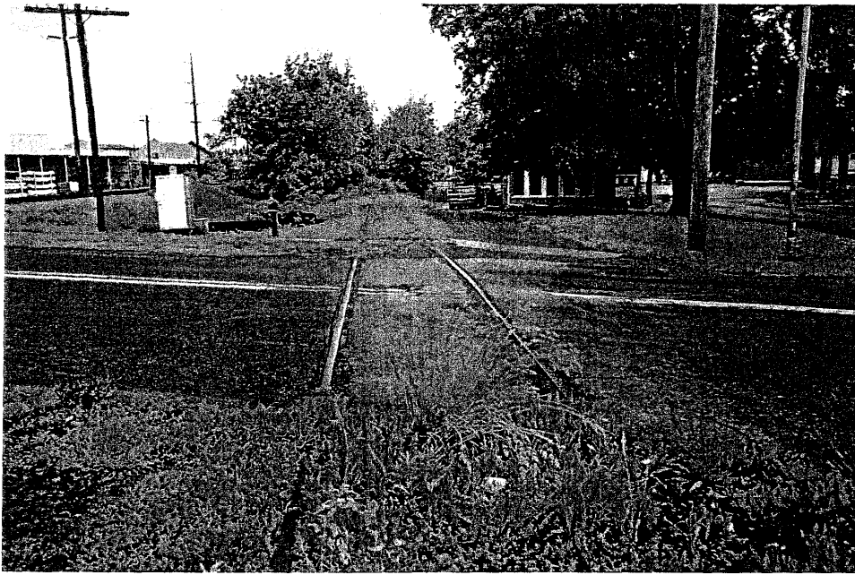
Photo K: Winter St. and TBCR ROW (approx. MP 45.8) looking WSW.
