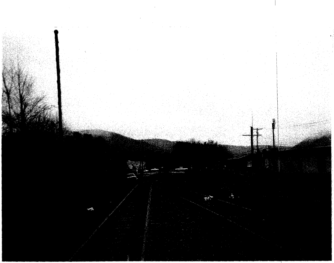
Picture 27: M.P. 149.6 - East End/Customer Siding
