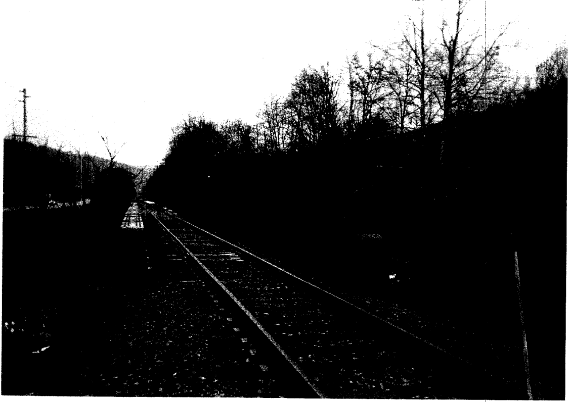
Picture 21: M.P. 147.82 - Ballast Deck Bridge/Top-Side View
