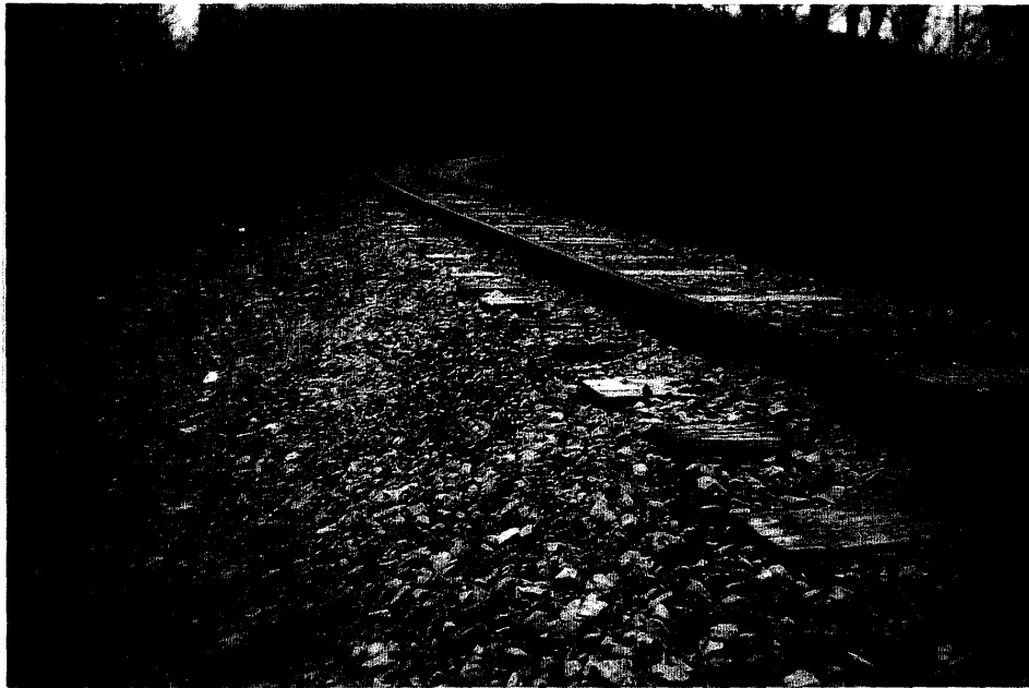
Picture 5: M.P. 134.5 - Continuous Welded Railway
