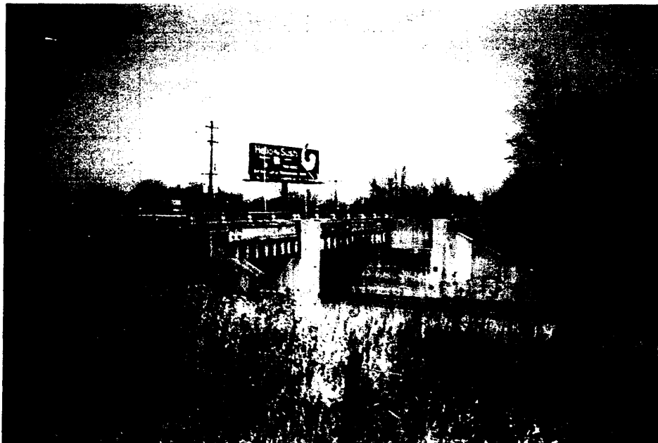
Bridge - Looking East
