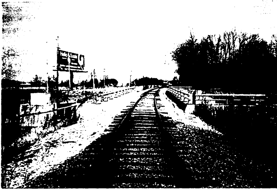
Bridge - Looking East
