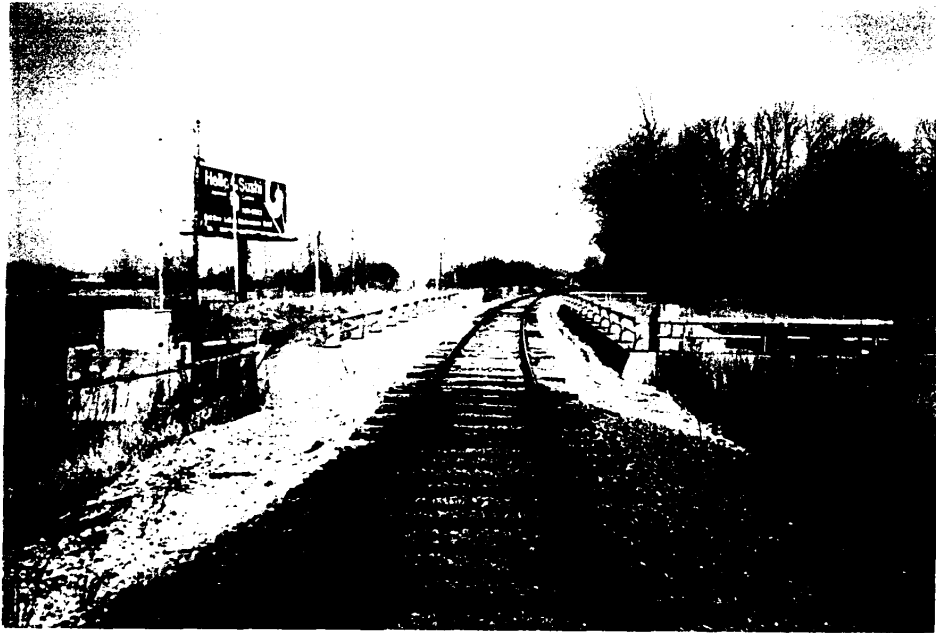
Bridge - Looking East
