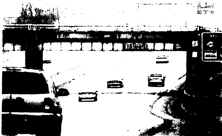
Bridge Viewed From I-75 - Looking South
