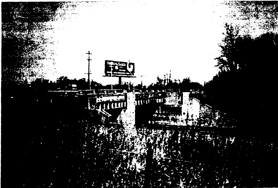
Bridge - Looking East
