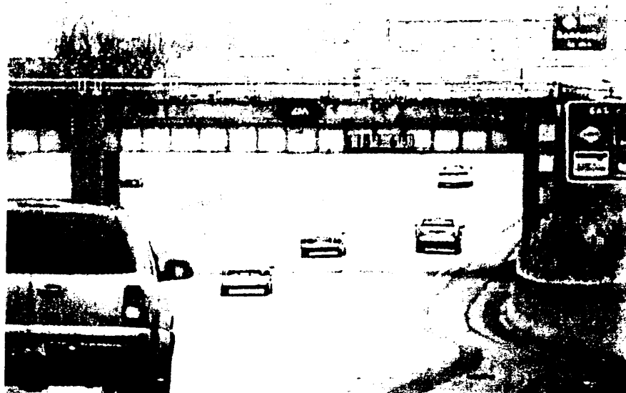
Bridge Viewed From I-75 - Looking South
