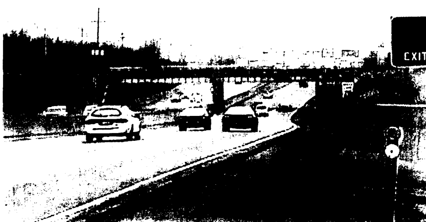
Bridge Viewed From I-75 - Looking South
