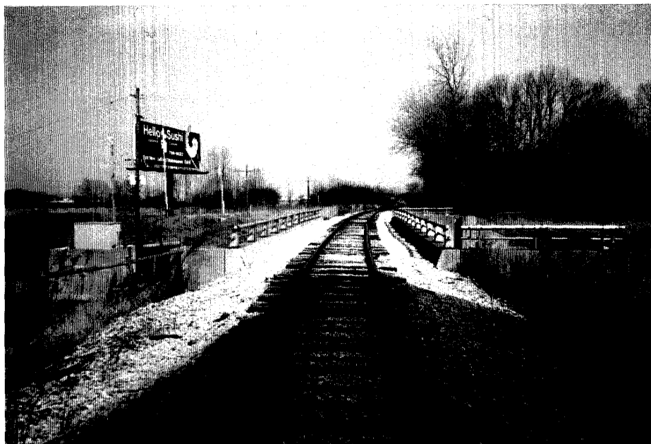
Bridge - Looking East
