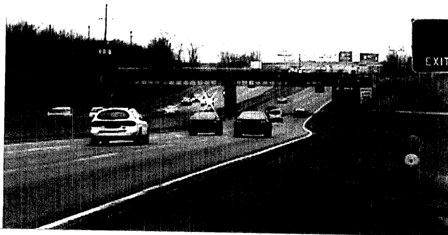
Bridge Viewed From I-75 - Looking South
