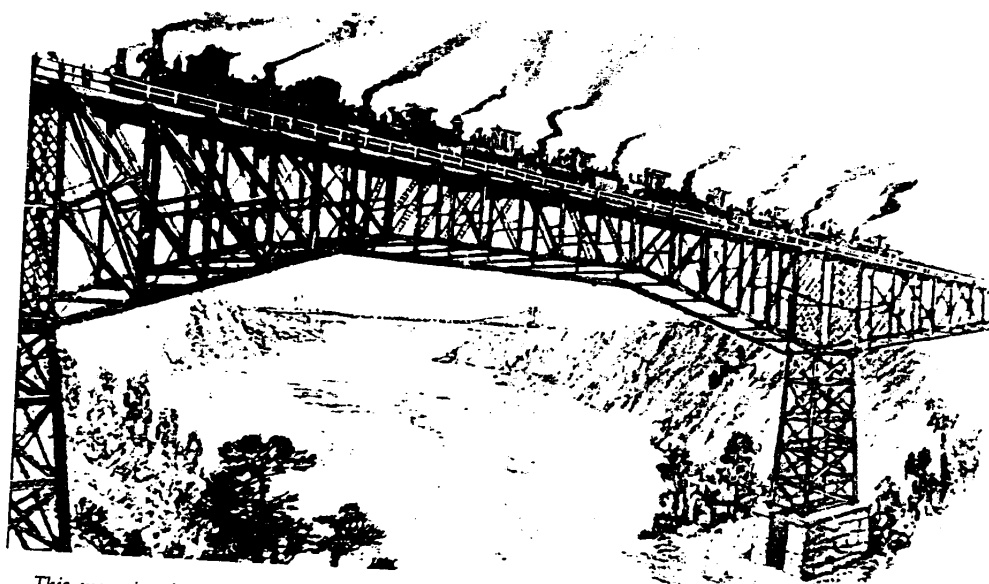
This engraving depicts the testing of the Niagara Cantilever Bridge with ten heavy locomotives.
