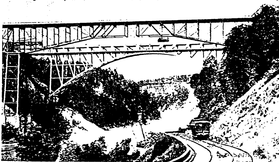
A tram of the Niagara Gorge Route passes below the Niagara Cantilever Bridge (MCRR) and behind it the steel arch bridge (GTR). The tram route would later be reduced to a narrow pathway for those willing to hike.
