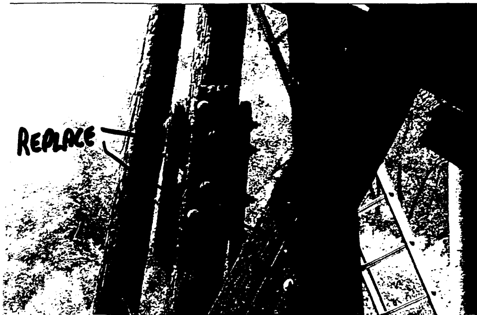
Bent 5, Post 5 and cross bracing.
