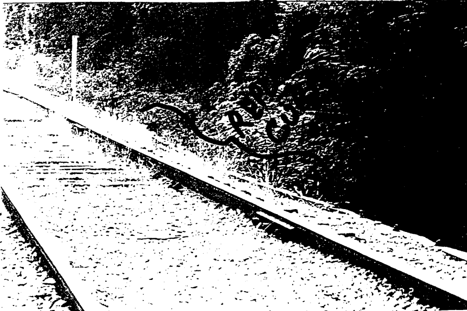
Curbing to be replaced on east side.
