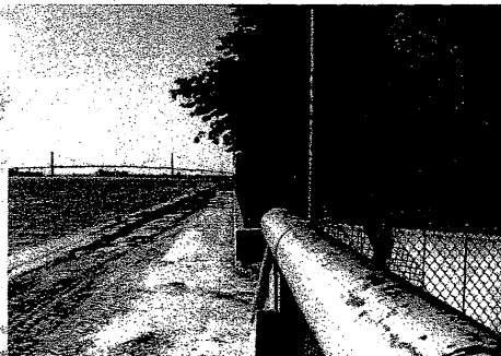
Views of the Civic Center Riverfront Promenade construction in late summer of 2000.
