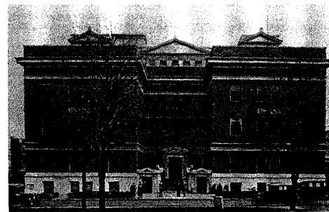
The 1914 building, the first building built for an integrated group medical practice.
