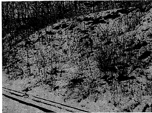
Figure 4A: Small slump immediately uphill of the existing tracks, 1/2 mile east of Le Hillier. The debris from the slump is removed. The scar of the slope failure is highlighted by the absence of snow on the nearly vertical surface. Small slumps of this nature could periodically cover the tracks with earthen and plant debris. Simple retaining walls or reshaping the slope will alleviate negative impacts on the existing rail corridor.
