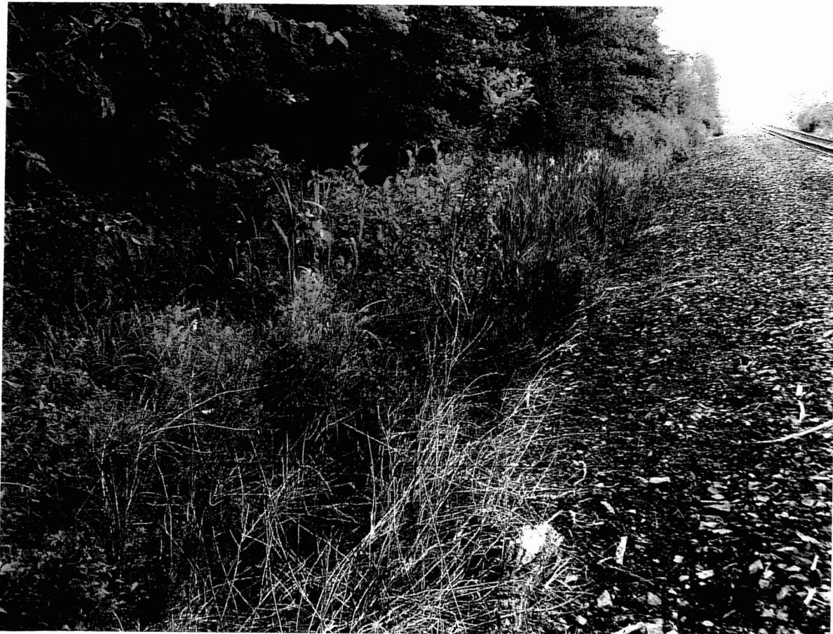
Photograph No. 8: Area of new crossing of the creek (to left through woods) and tie down location on existing railroad line.
