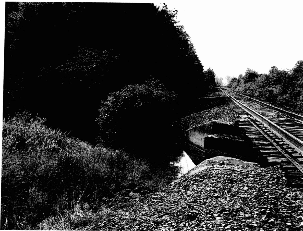
Photograph No. 5: Existing railroad where new Laurel Run creek crossing segment ties down.
