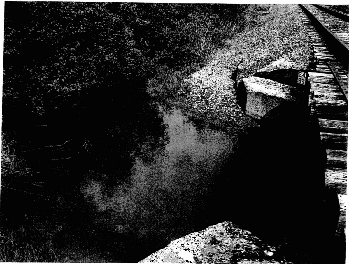
Photograph No. 7: Opposite side of existing bridge with no Sparganium in direct area but is just out of the work area so indirect impacts could occur if bridge replacement occurs.
