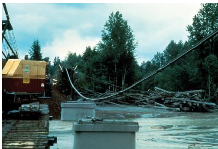
South Toutle Bridge during reconstruction
