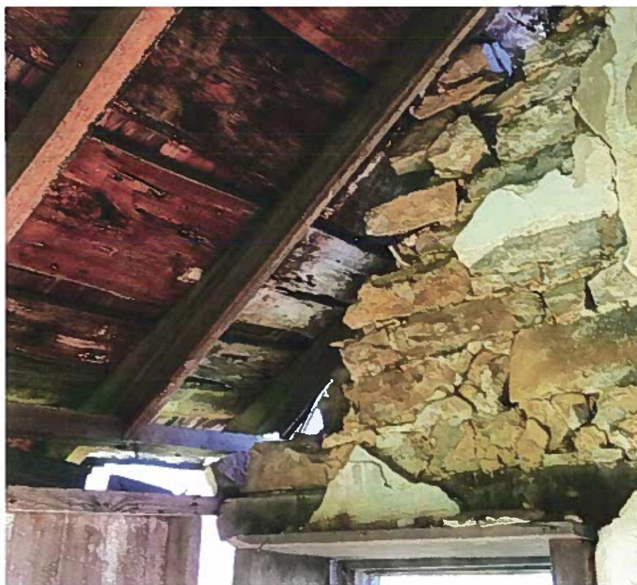
PHOTO 6: VIEW OF SOUTH WEST END OF HEADER BEAM
