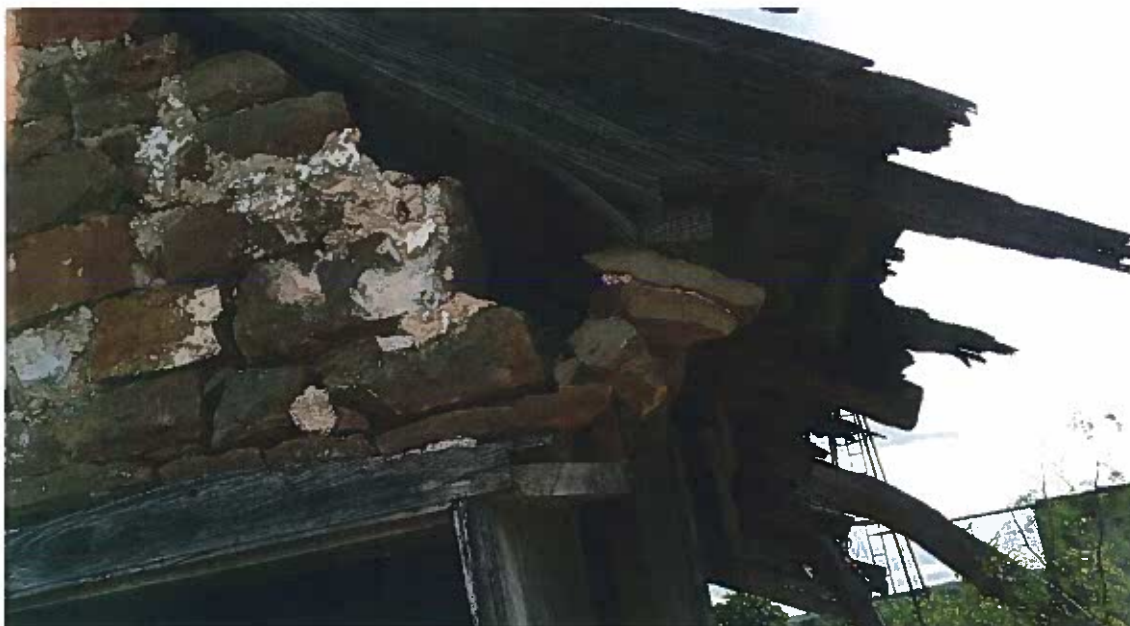
PHOTO 7: VIEW OF OUTSIDE OF SOUTH WEST HEADER BEAM SITTING ON STONE
