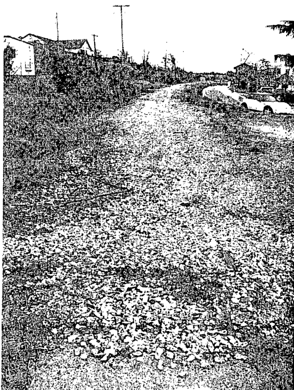
Photo 2: Looking east from Hwy 49 crossing, Martel Depot in background.
