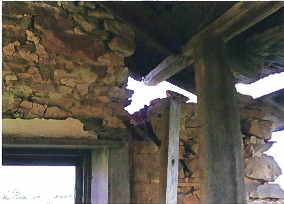
PHOTO 5: VIEW AT NORTH WEST END OF HEADER BEAM
