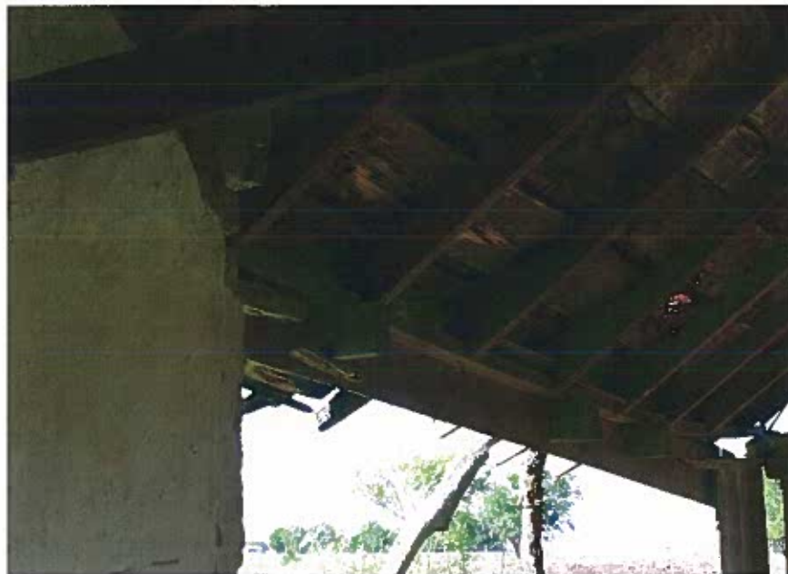
PHOTO 8: VIEW SHOWING REMOVED TIE BEAMS FOR RAFTER ON WEST SIDE
