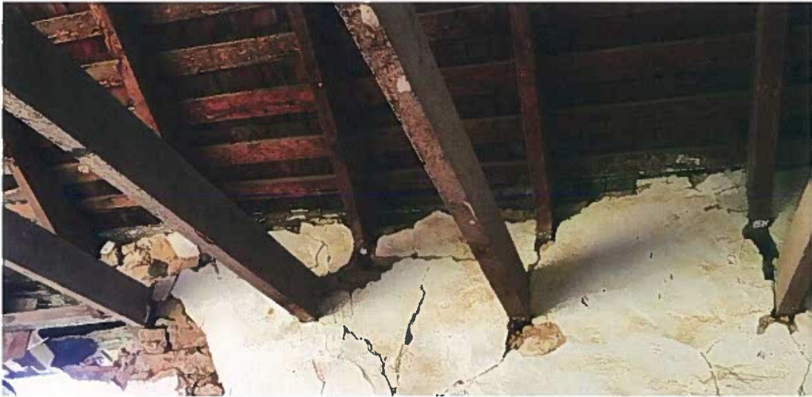
PHOTO 9: VIEW SHOWING TIE BEAM FOR RAFTER ON EAST SIDE
