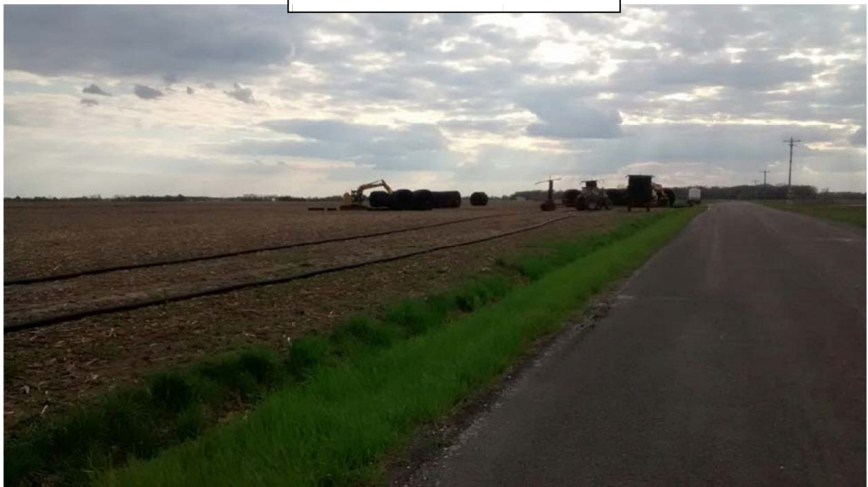
Drainage system installed on 400 South, Spring 2016 by Peterson Farms.
