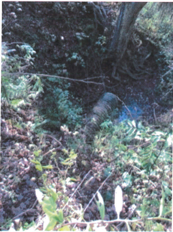
Stone Culvert at milepost CAJ 0.4
