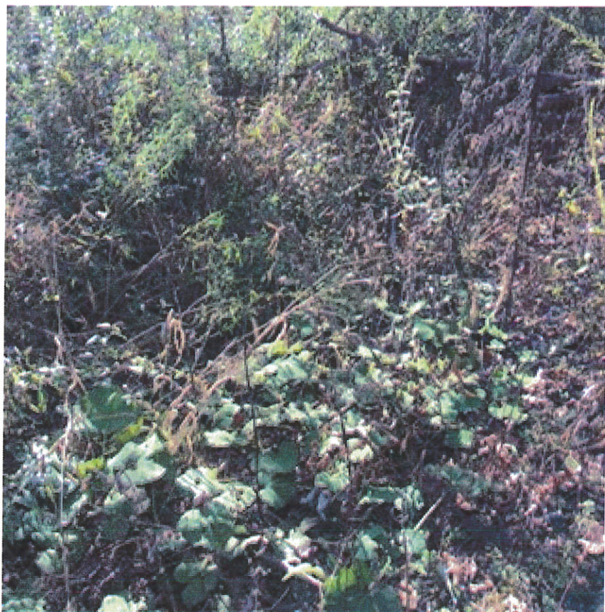
Cast Iron Culvert at milepost CAJ 0.8
