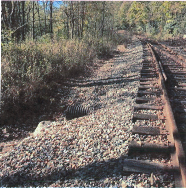
Stone Culvert at milepost CAJ .48
