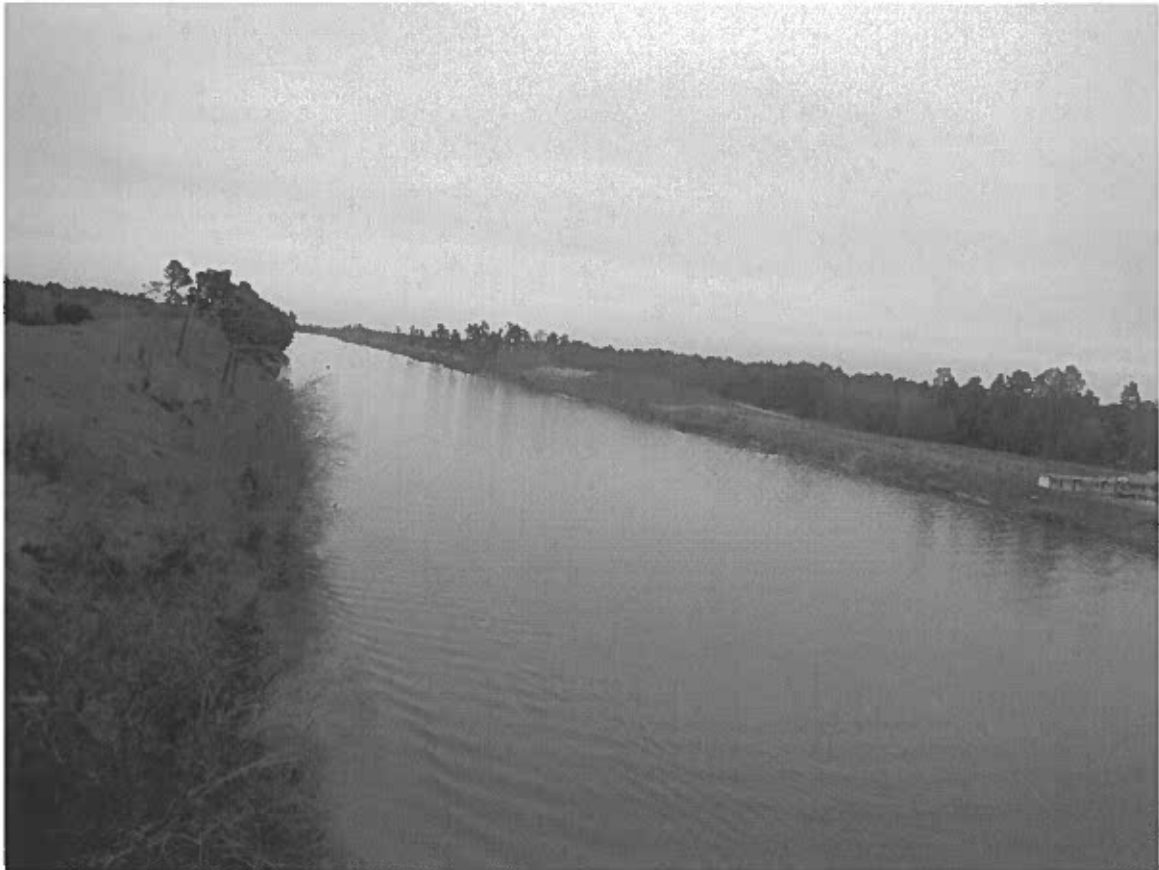
Photograph 2 Diversion Canal, view southeast
