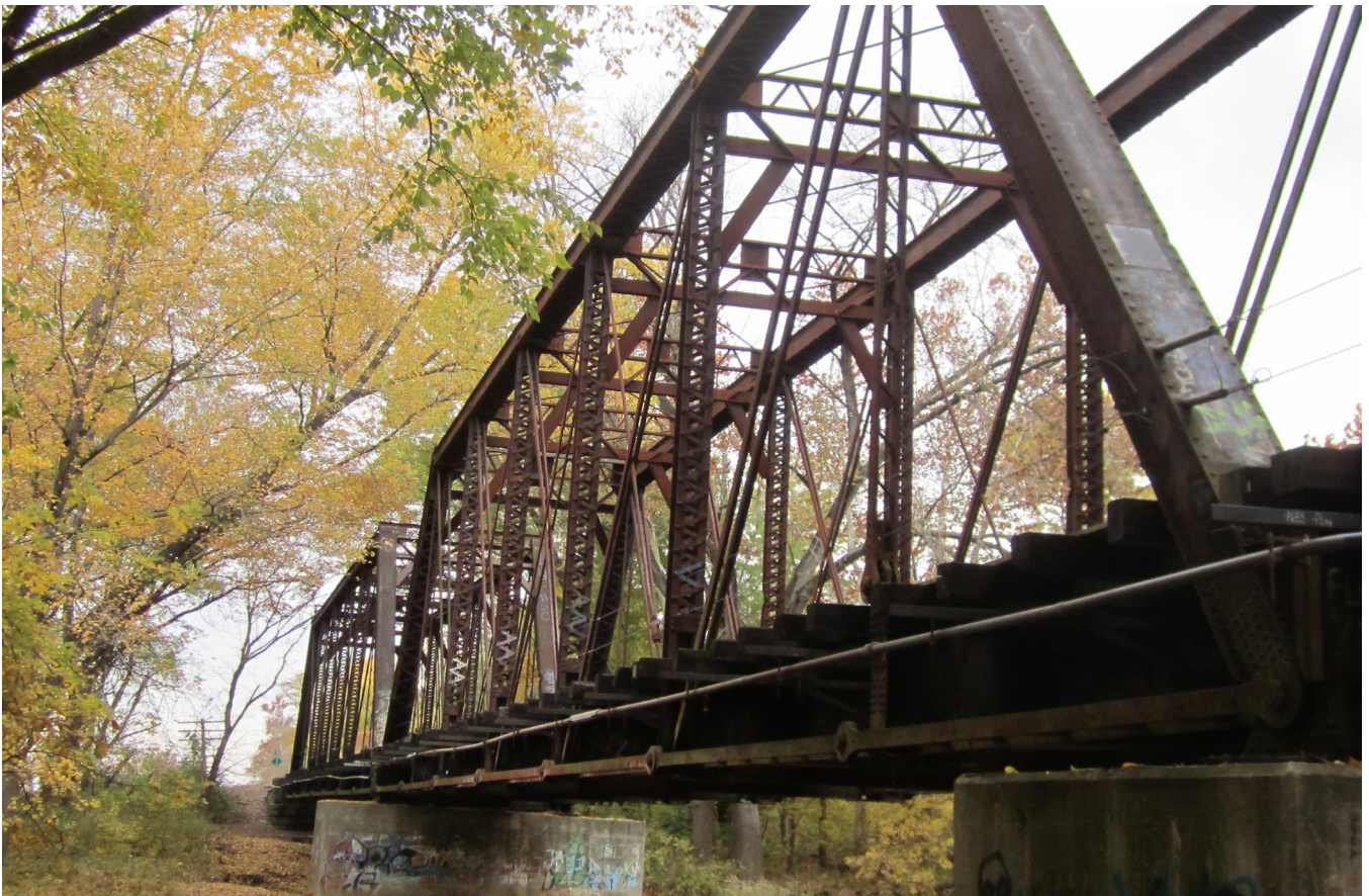
Bridge MP 40.19 Photo 4 - Looking Northeast at Concrete Piers, Top Chord, Floor Beams, Portal Struts and Bracing, Sway Bracing, Lateral Bracing, Bottom Chord, Eyebars & Verticals
