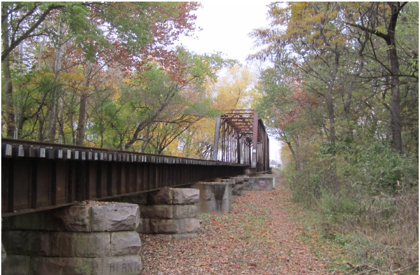
Bridge MP 40.19 Photo 1 - Looking North at South Masonry Piers, South Concrete Abutment, Bridge Superstructure, & Truss Members
