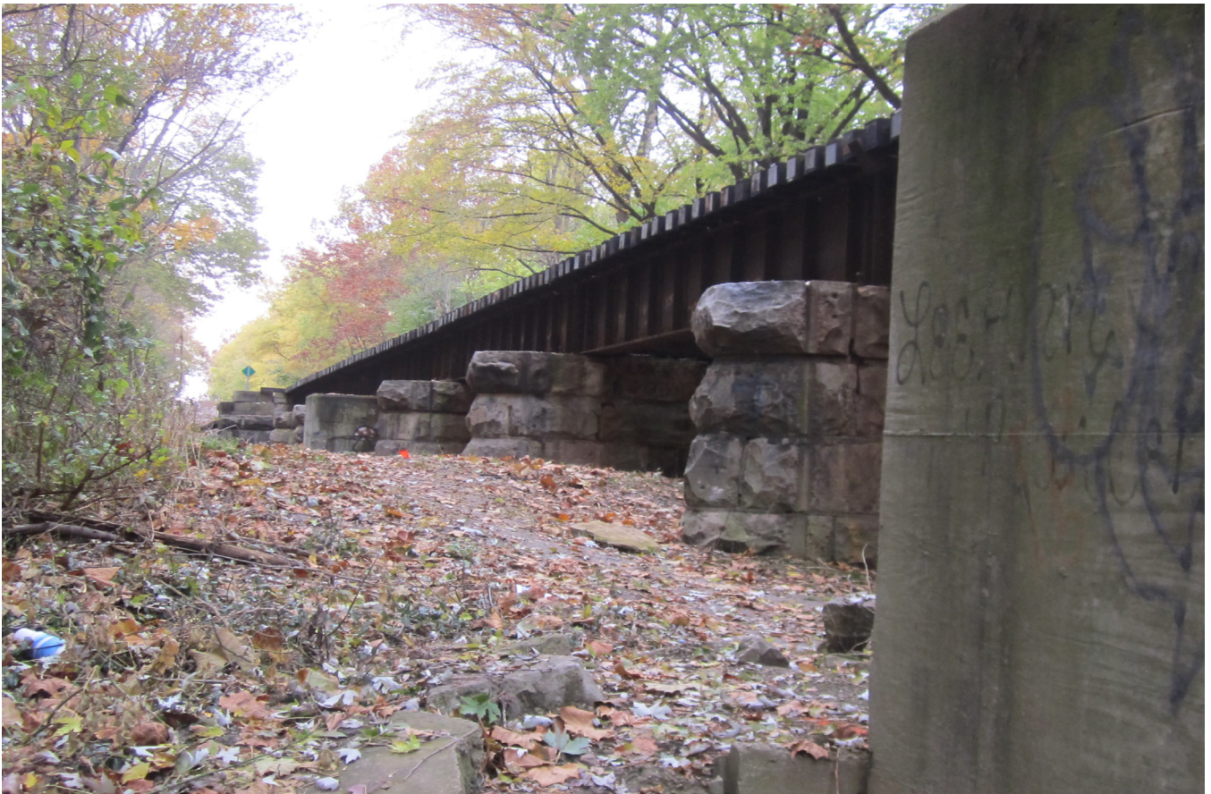
Bridge MP 40.19 Photo 13 - Looking Southeast at Bridge South Abutment & Piers
