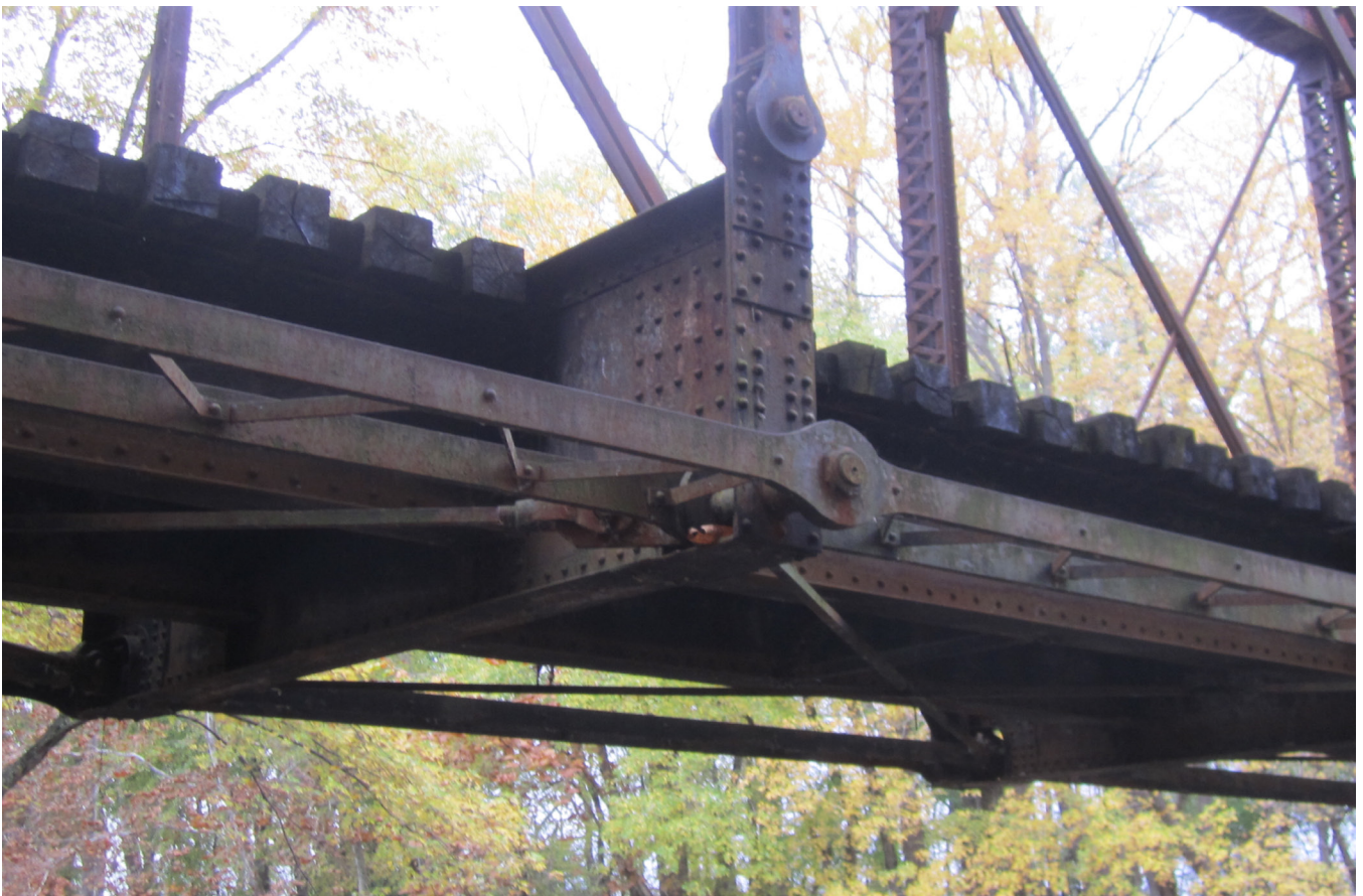
Bridge MP 40.19 Photo 9 - Looking Northeast at East Elevation Pinned Connection, Lower Chord, Floor Deck, Lower Lateral Bracing & Floor Beam
