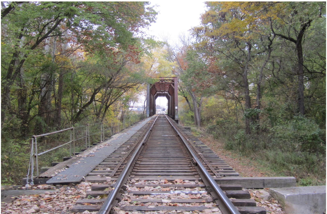
Bridge MP 40.19 Photo 2 - Looking Northwest at Bridge Deck, Two Truss Lines, & South Abutment
