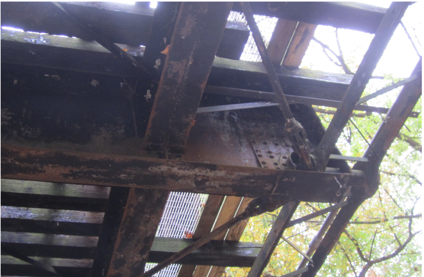
Bridge MP 40.19 Photo 8 - Looking Northeast at Bridge Substructure Connection
