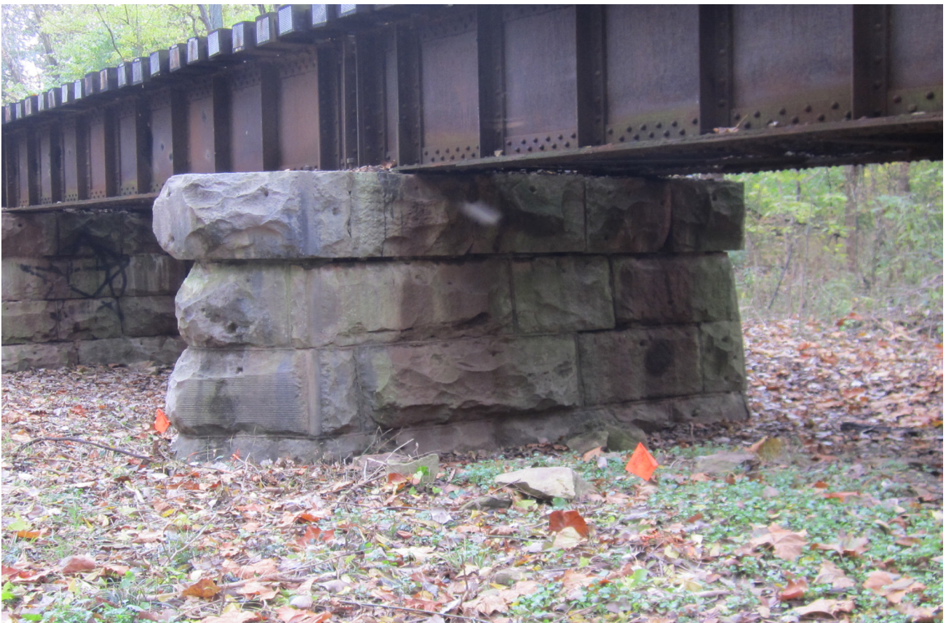
Bridge MP 40.19 Photo 5 - Looking Southwest at South Stone Masonry Pier
