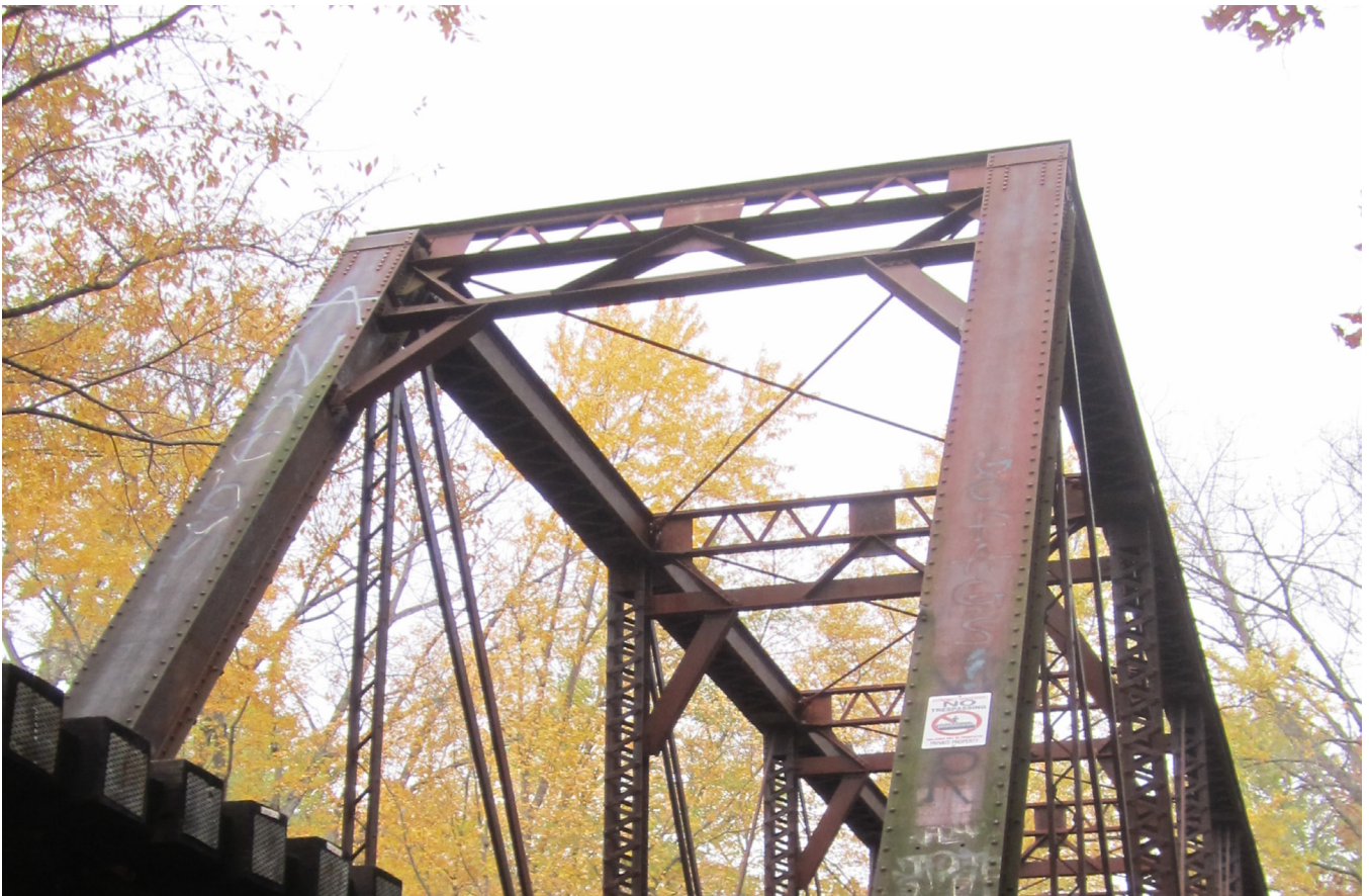
Bridge MP 40.19 Photo 6 - Looking Northwest at South End Posts, Portal Bracing, Sway Bracing, Lateral Bracing & Floor Beams
