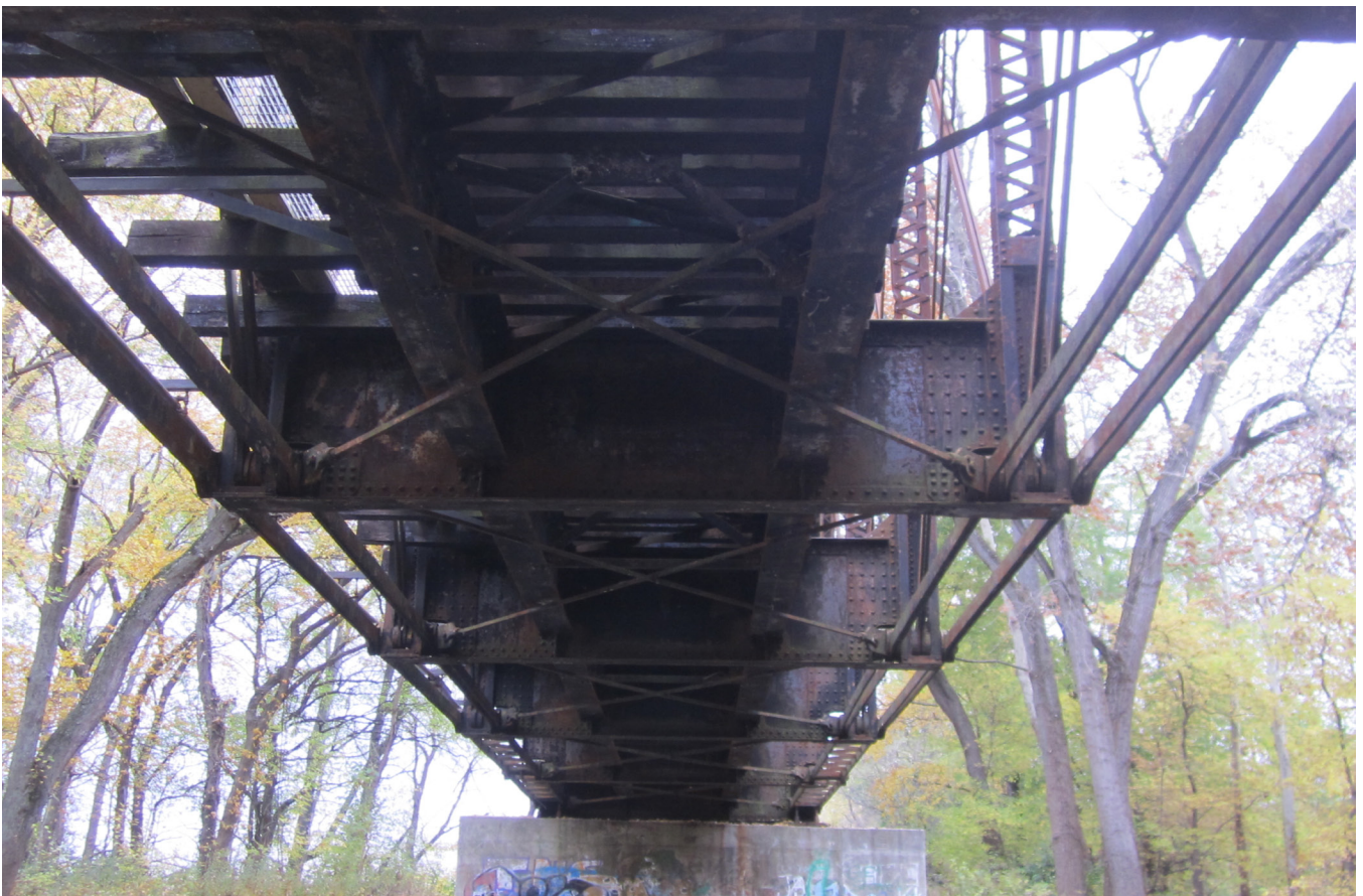
Bridge MP 40.19 Photo 7 - Looking Northeast at Bridge Substructure, Lower Lateral Bracing, Lower Chord, Floor Beams, Stringers & Eyebars
