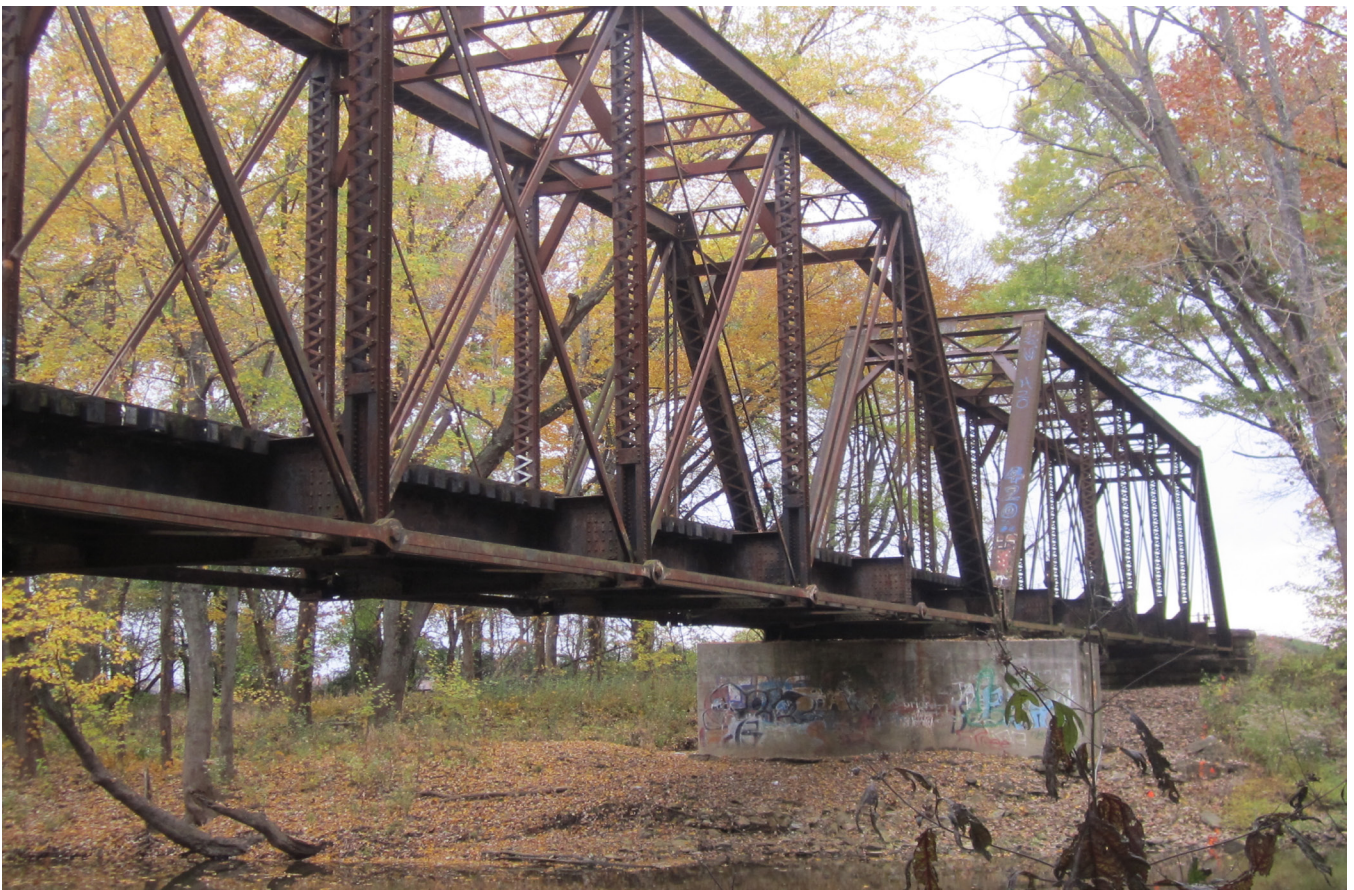
Bridge MP 40.19 Photo 3 - Looking Northwest at Top Chord, Floor Beams, Portal Struts and Bracing, Sway Bracing, Lateral Bracing, Bottom Chord, Eyebars, Piers & South Abutment
