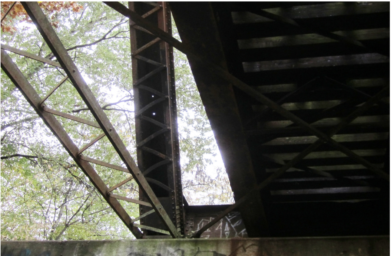
Bridge MP 40.19 Photo 12 - Looking Southeast at South End Substructure, Vertical Member & Eyebars
