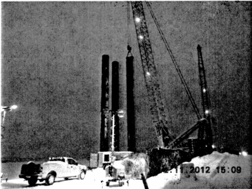
Figure 2. Pier 7: Lofting and Splicing Top Pile
