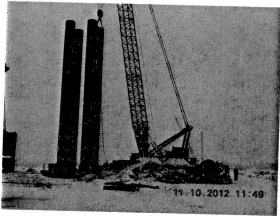
Figure 5. Ready to Drive 72" Piling at Pier 15, November 10, 2012
