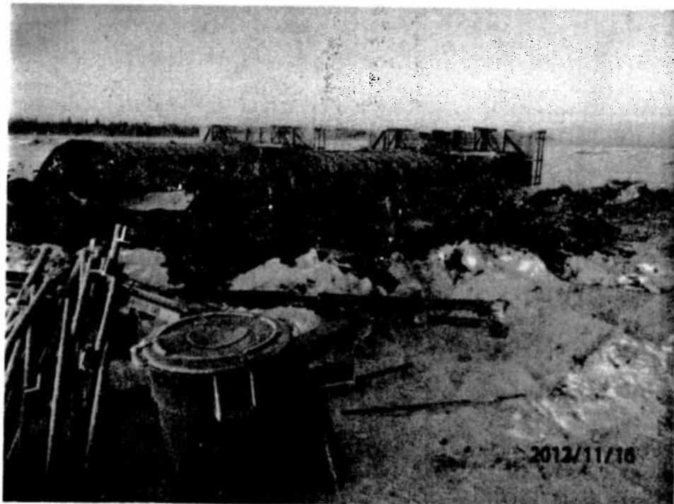
Figure 4. Heating Column Cap Forms, November 16, 2012
