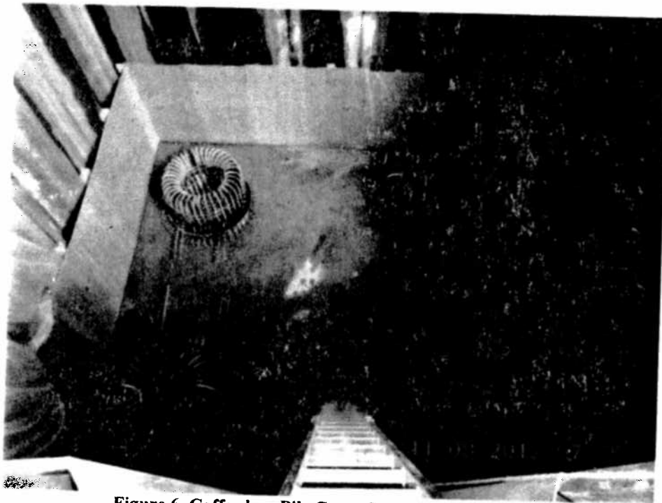
Figure 6. Cofferdam Pile Cages Set, November 8, 2012
