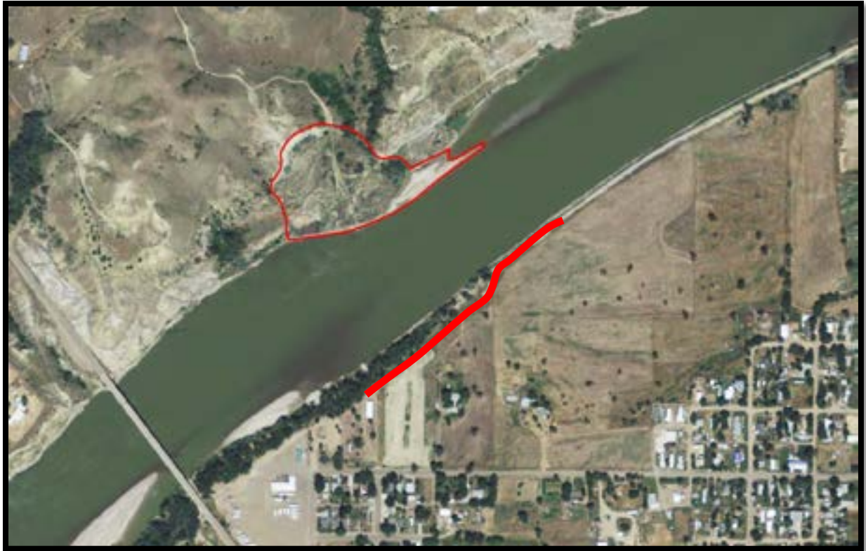
Figure 14: 2013 Aerial Image of Riverbank Failure (NAIP 2013)
