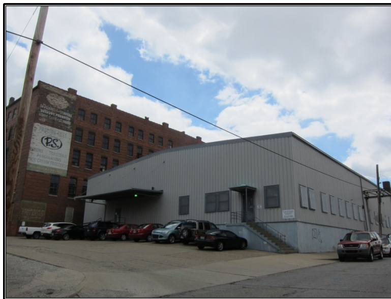
Figure 80. Site 34 (JFWS 985): Western finished products warehouse.
