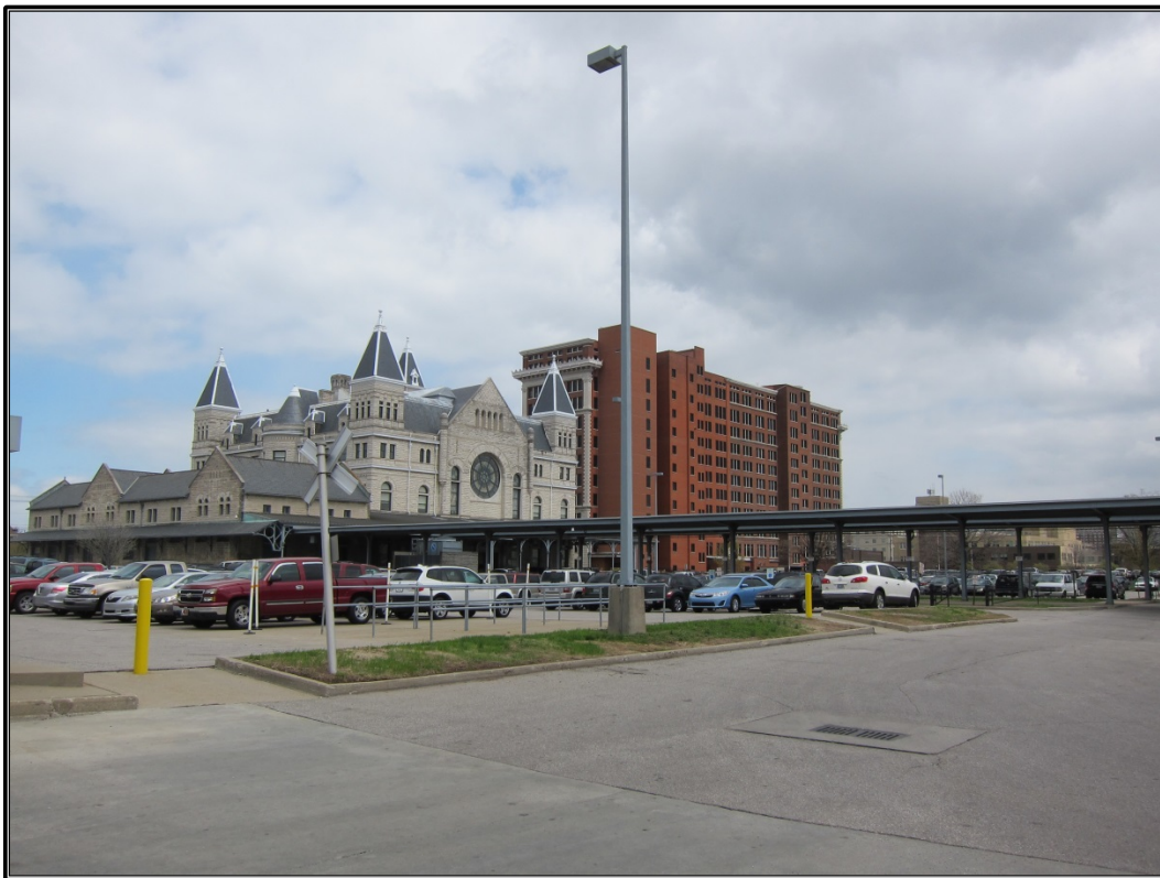
Figure 91. Site 38 (JFSW 401): Rear elevation.
