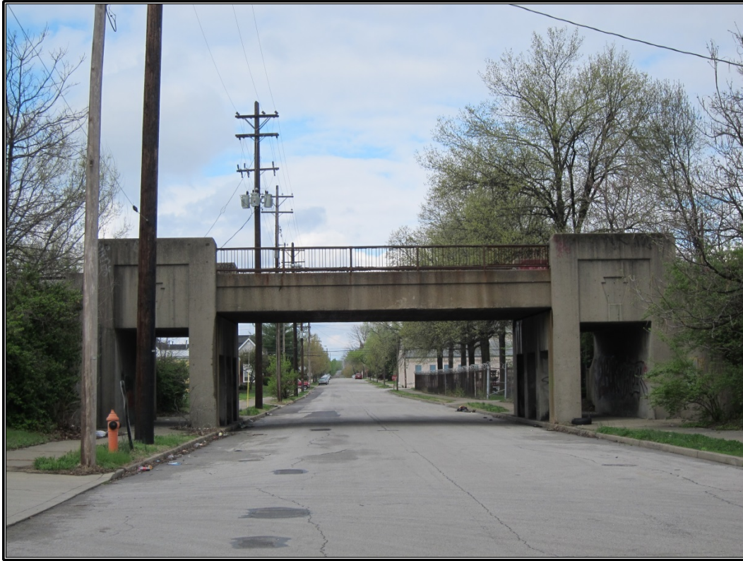
Figure 101. Site 19 (JFWR 3835): Westerly view of bridge.
