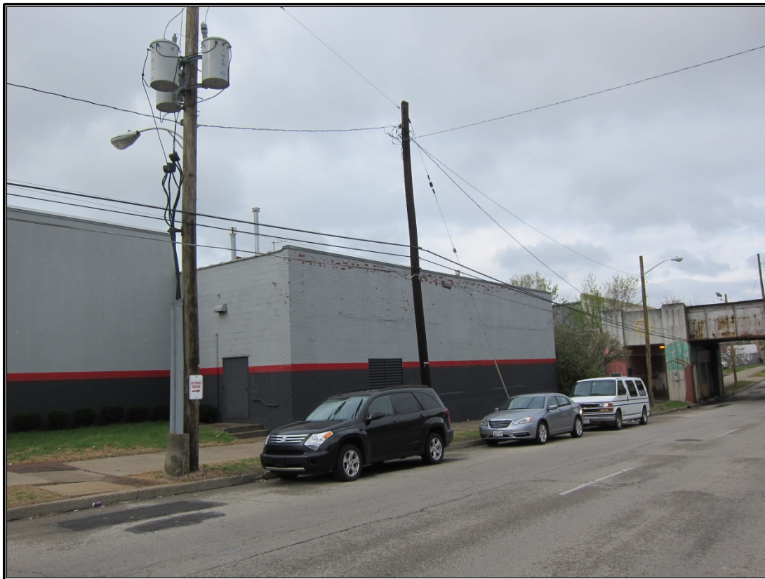
Figure 42. Site 14 (JFWR 3830): Original portion of the building constructed in 1945.
