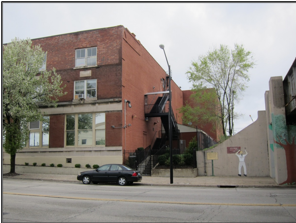
Figure 41. Site 13 (JFWR 3829): Large fire escape attached to the east elevation.
