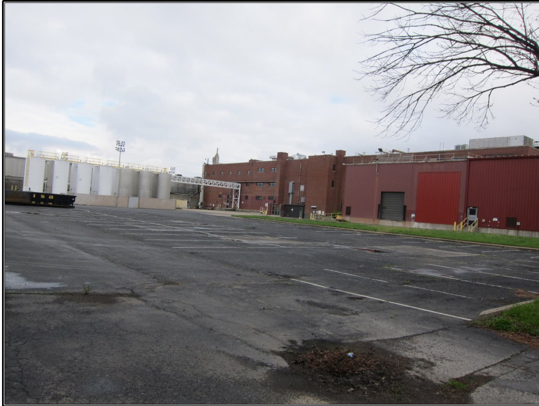
Figure 45. Site 15 (JFWR 3831): Rear elevation.
