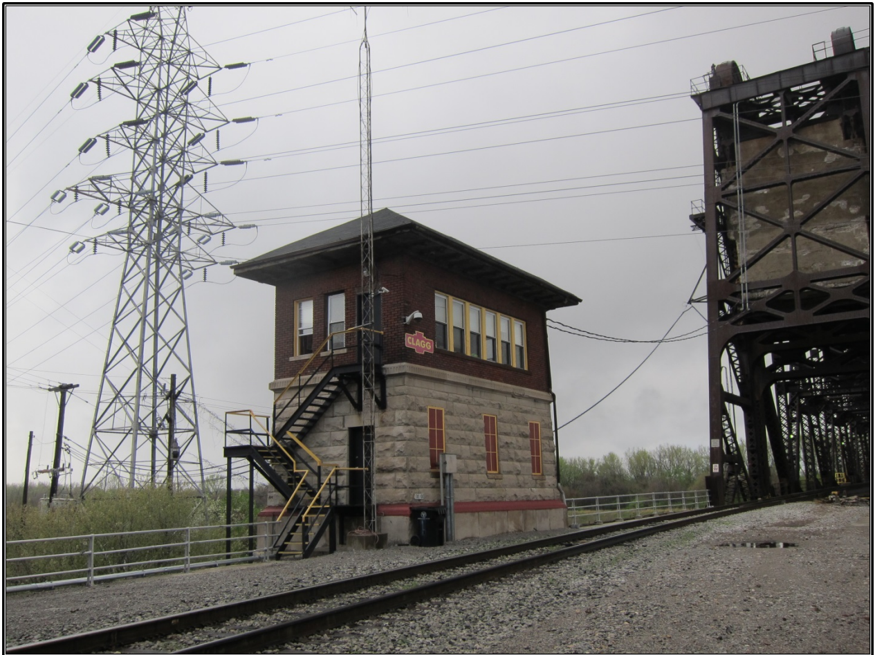
Figure 15. Site 1 (JFWP 327): Signal tower.
