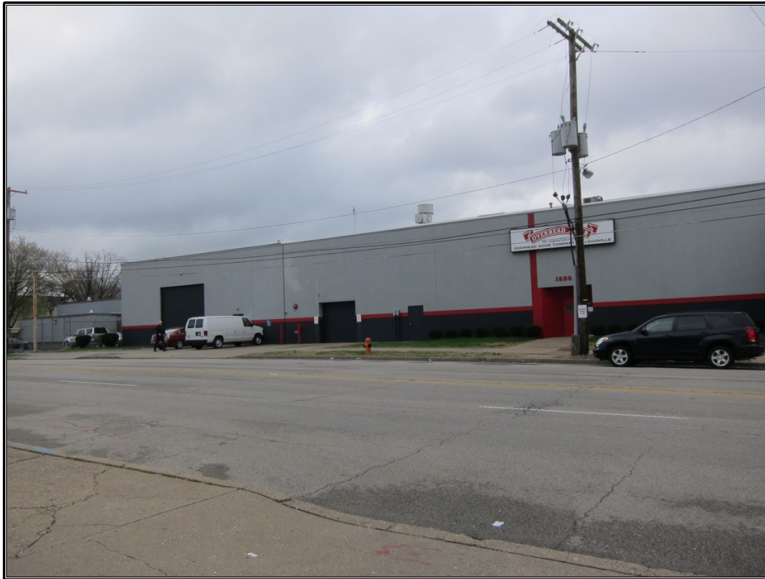
Figure 43. Site 14 (JFWR 3830): Later addition.
