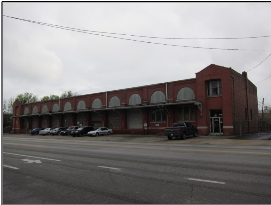
Figure 36. Site 9 (JFWR 3825): Northwesterly view of building.
