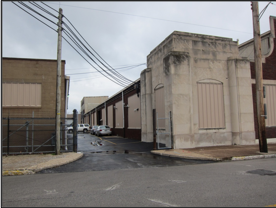
Figure 35. Site 8 (JFWP 616): Rear elevation.
