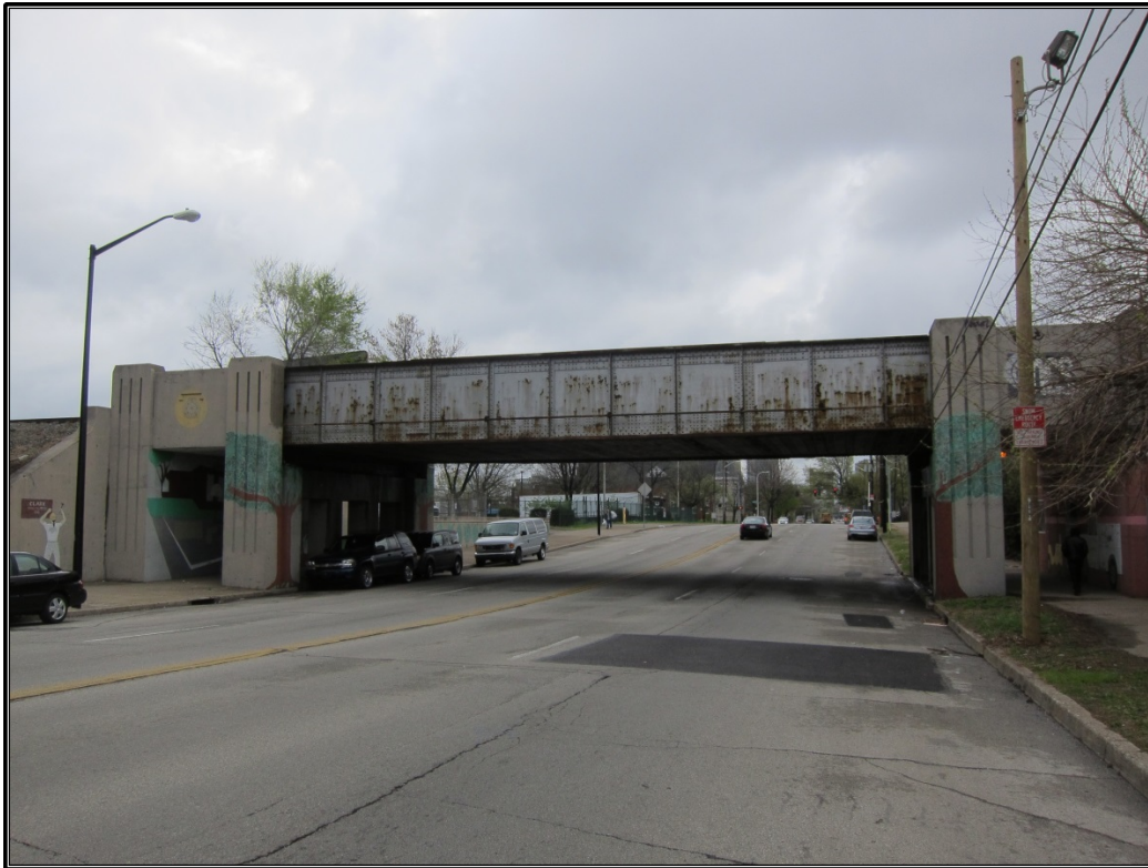
Figure 96. Site 12 (JFWR 3828): Easterly view of bridge.
