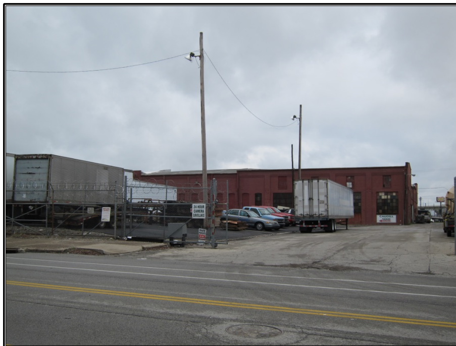
Figure 32. Site 7 (JFWP 149): Rear elevation of the former National Foundry and Machine Company.
