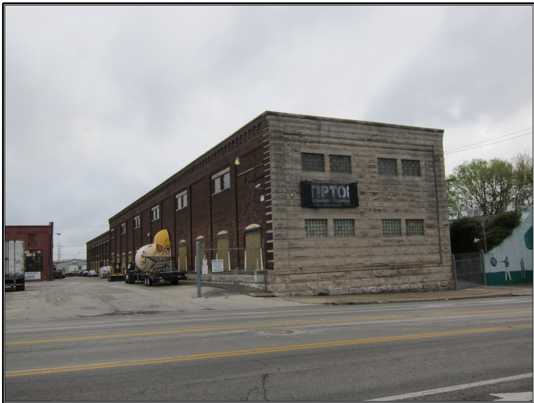
Figure 28. Site 6 (JFWP 148): Rear elevation of the Monon Freight Depot.
