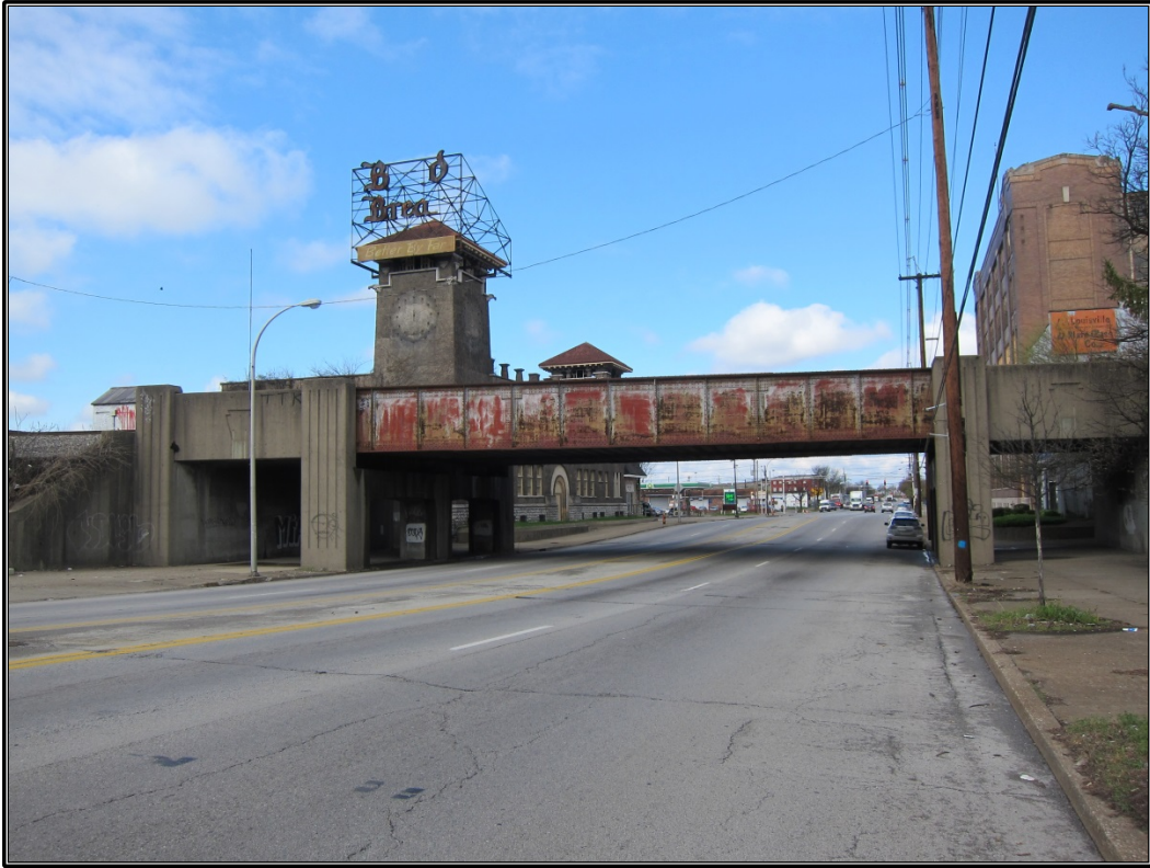
Figure 99. Site 25 (JFWR 3840): Westerly view of bridge.
