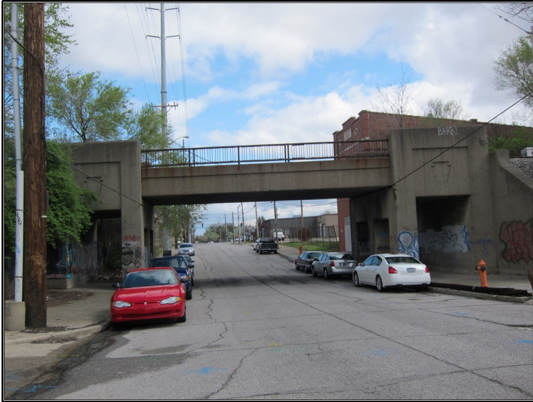
Figure 103. Site 31 (JFSW 982): Northerly view of bridge.
