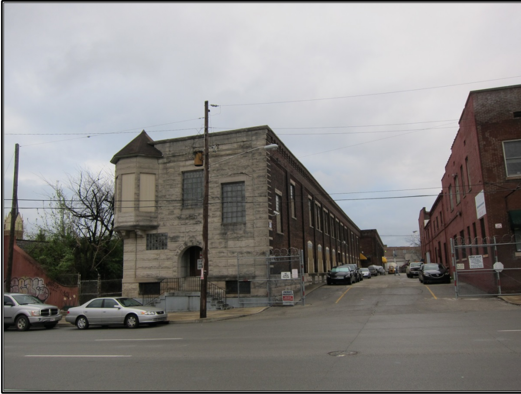
Figure 27. Site 6 (JFWP 148): Monon Freight Depot.
