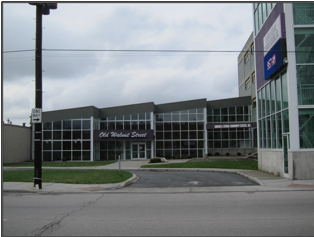
Figure 48. Site 17 (JFWR 3833): Breezeway.
