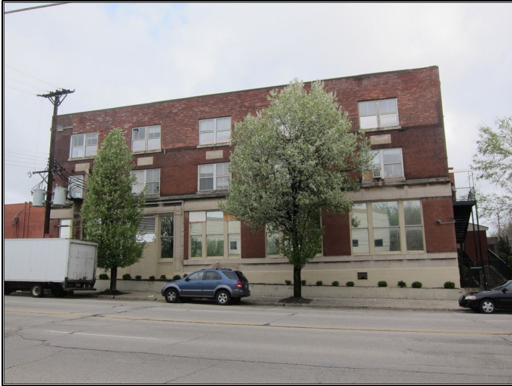
Figure 40. Site 13 (JFWR 3829): Northerly view of building.
