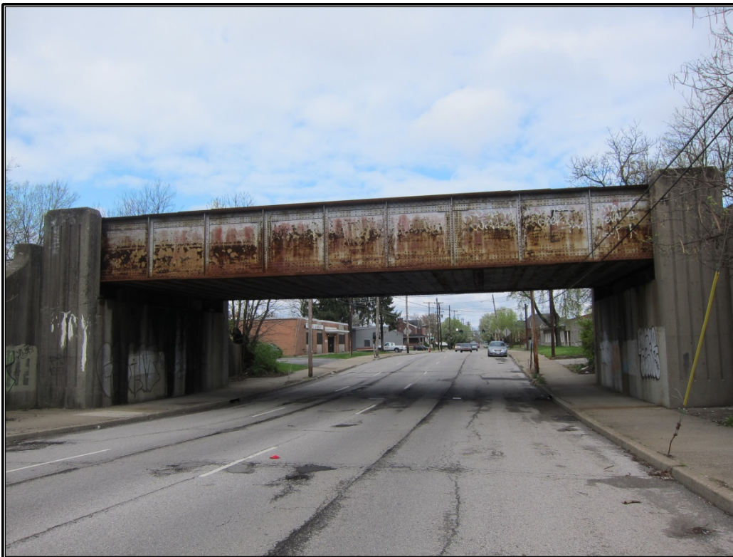
Figure 98. Site 21 (JFWR 3837): Westerly view of bridge.
