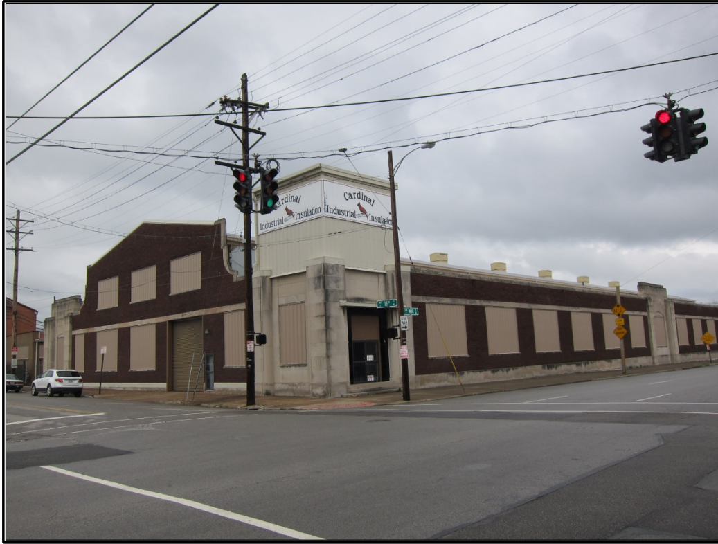
Figure 34. Site 8 (JFWP 616): Southwesterly view of warehouse.
