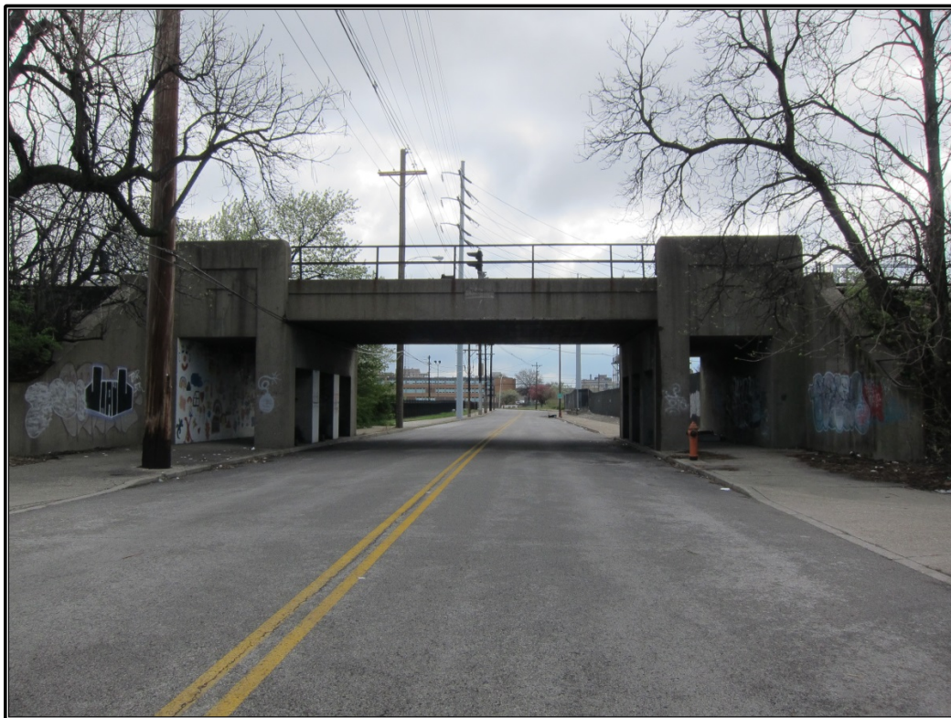
Figure 102. Site 23 (JFWR 3839): Easterly view of bridge.
