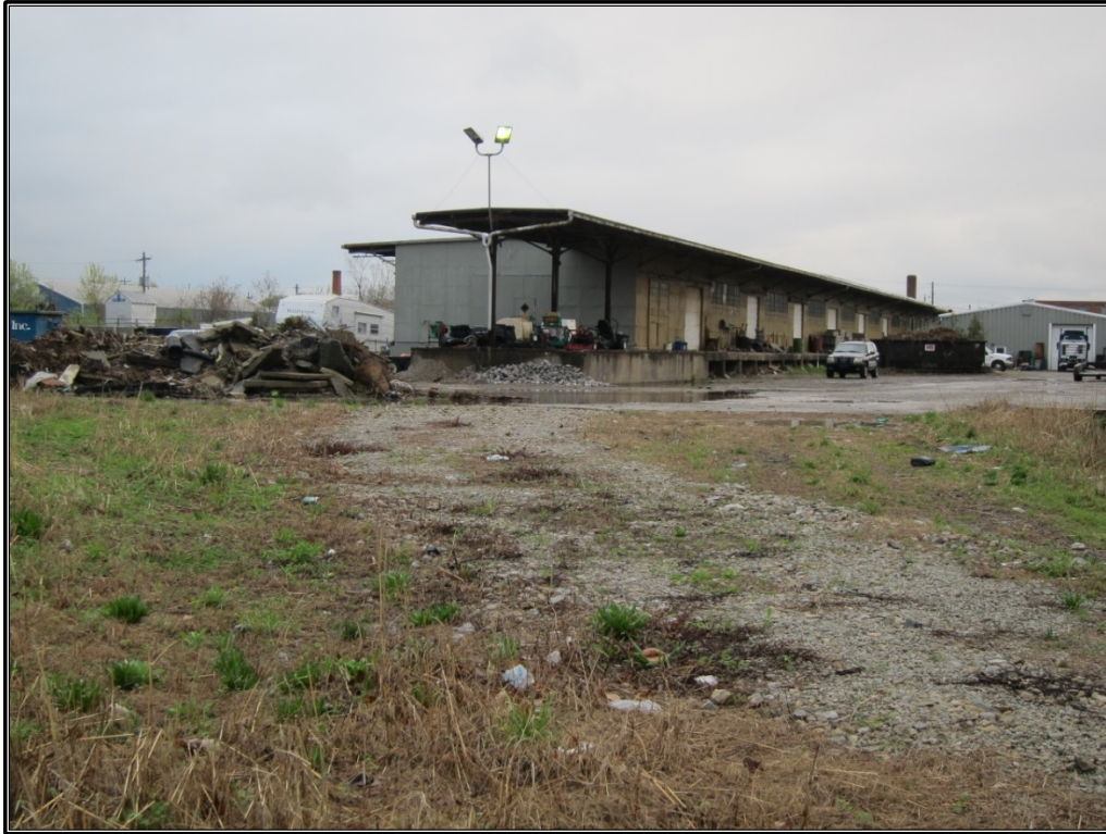
Figure 23. Site 3 (JFWP 614): Southeasterly view of warehouse.
