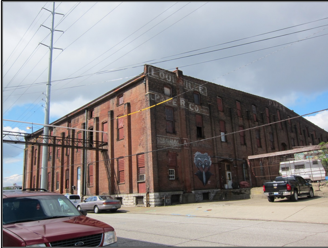
Figure 70. Site 32 (JFSW 983): Rear elevation of Site 32.
