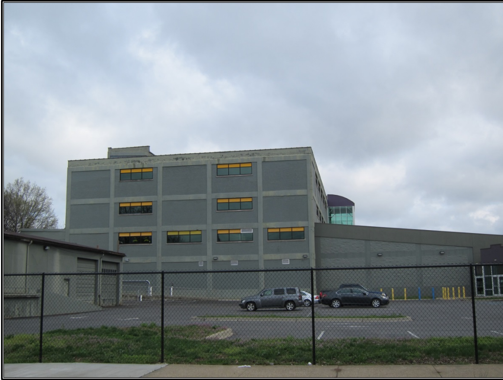
Figure 47. Site 17 (JFWR 3833): Rear elevation.
