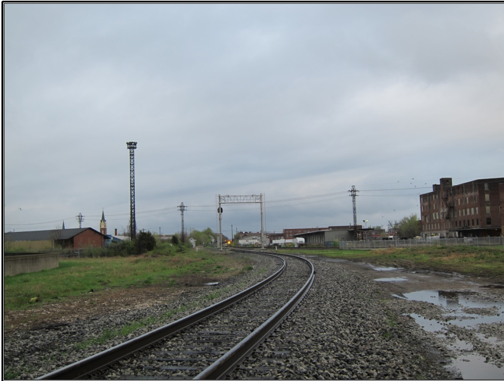
Figure 4. Overview of L&I railroad from just south of the Pennsylvania Railroad bridge.
