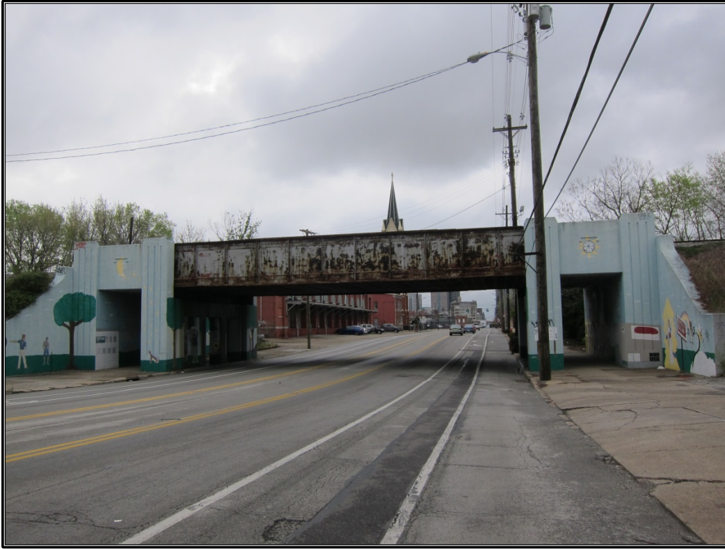
Figure 95. Site 10 (JFWR 3826): Easterly view of bridge.
