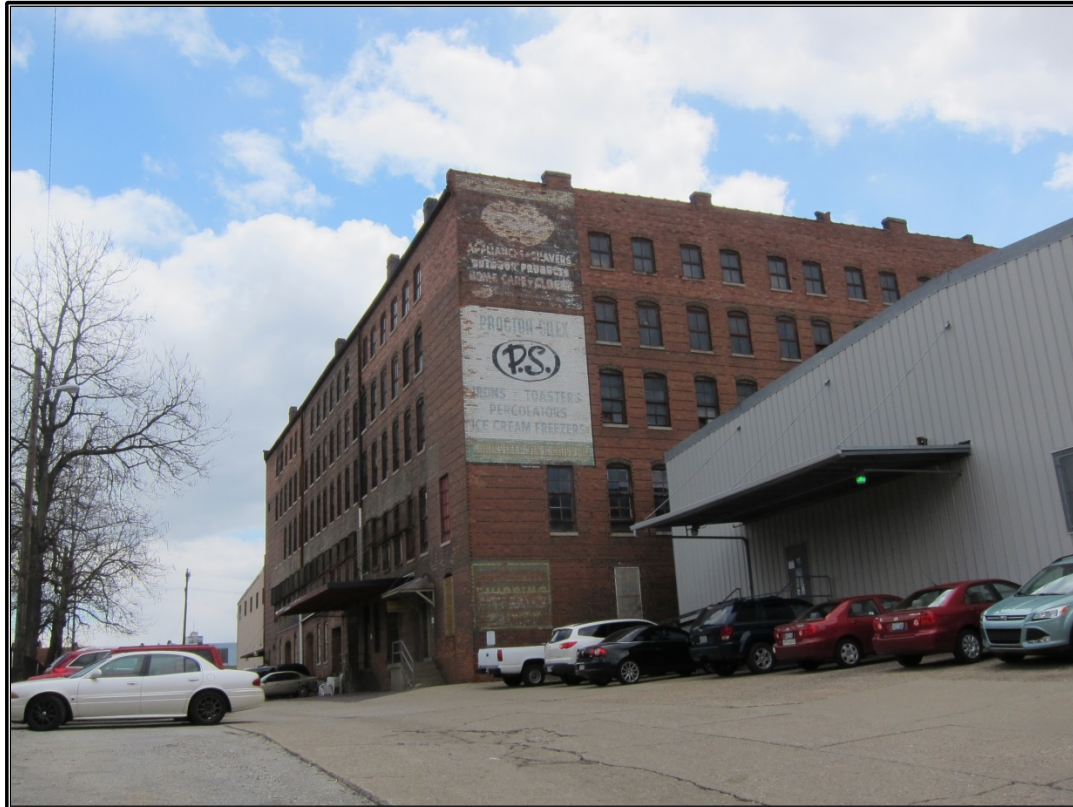
Figure 76. Site 34 (JFSW 985): Southeasterly view of central factory building.
