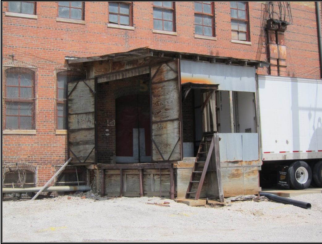
Figure 78. Site 34 (JFSW 985): Detail of loading dock.
