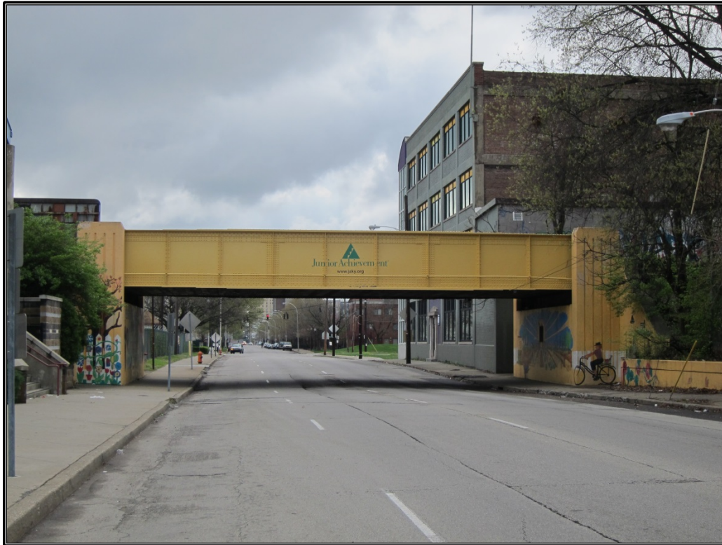
Figure 97. Site 16 (JFWR 3832): Easterly view of bridge.
