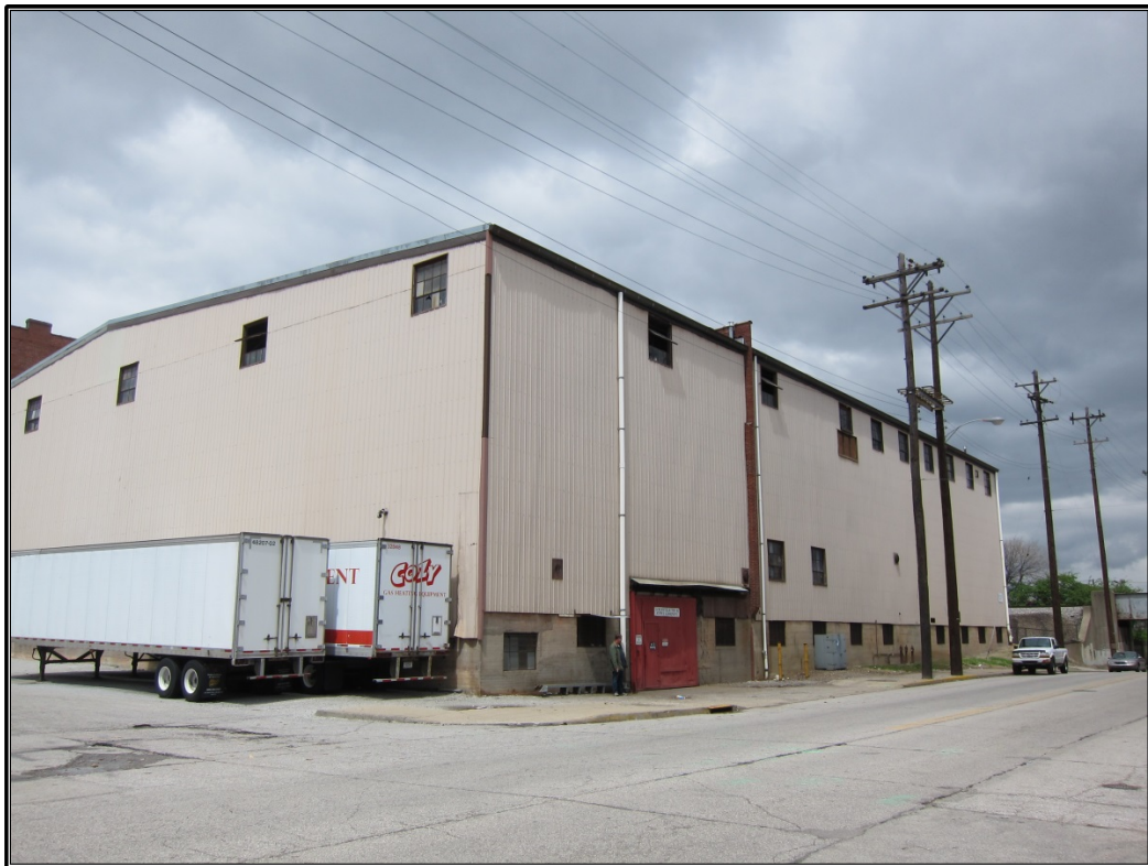
Figure 79. Site 34 (JFWS 985): Eastern finished products warehouse.
