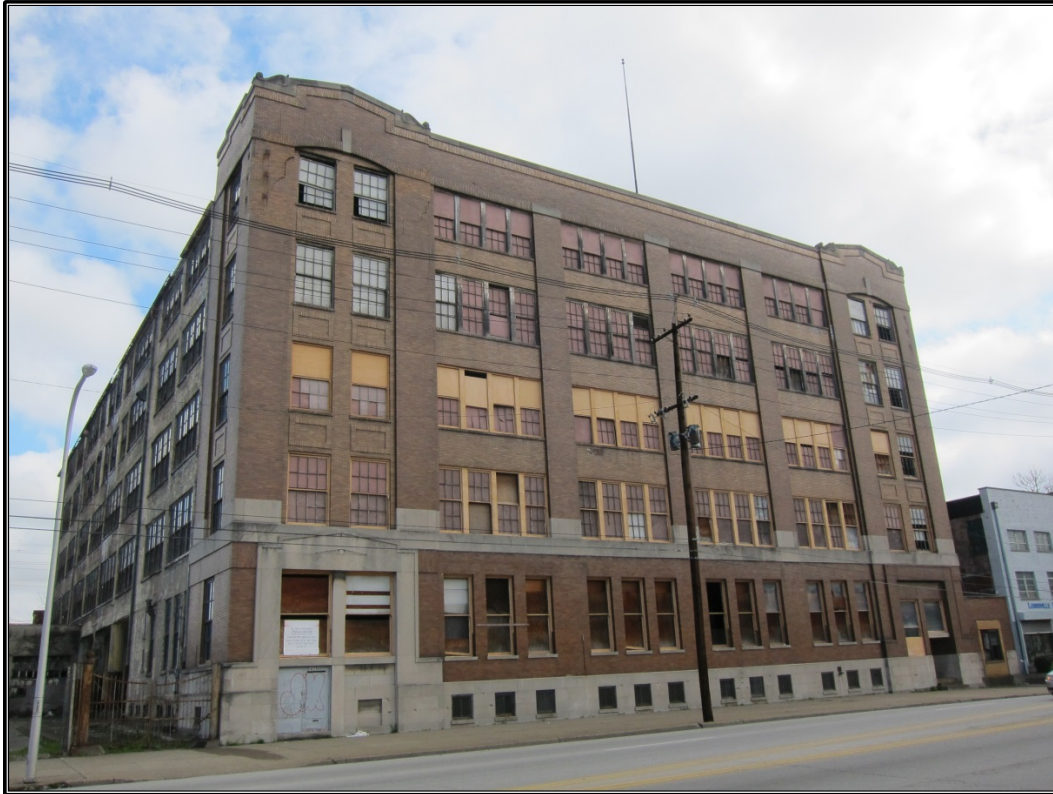
Figure 54. Site 24 (JFSW 436): Axton-Fisher Tobacco Company Warehouse.
