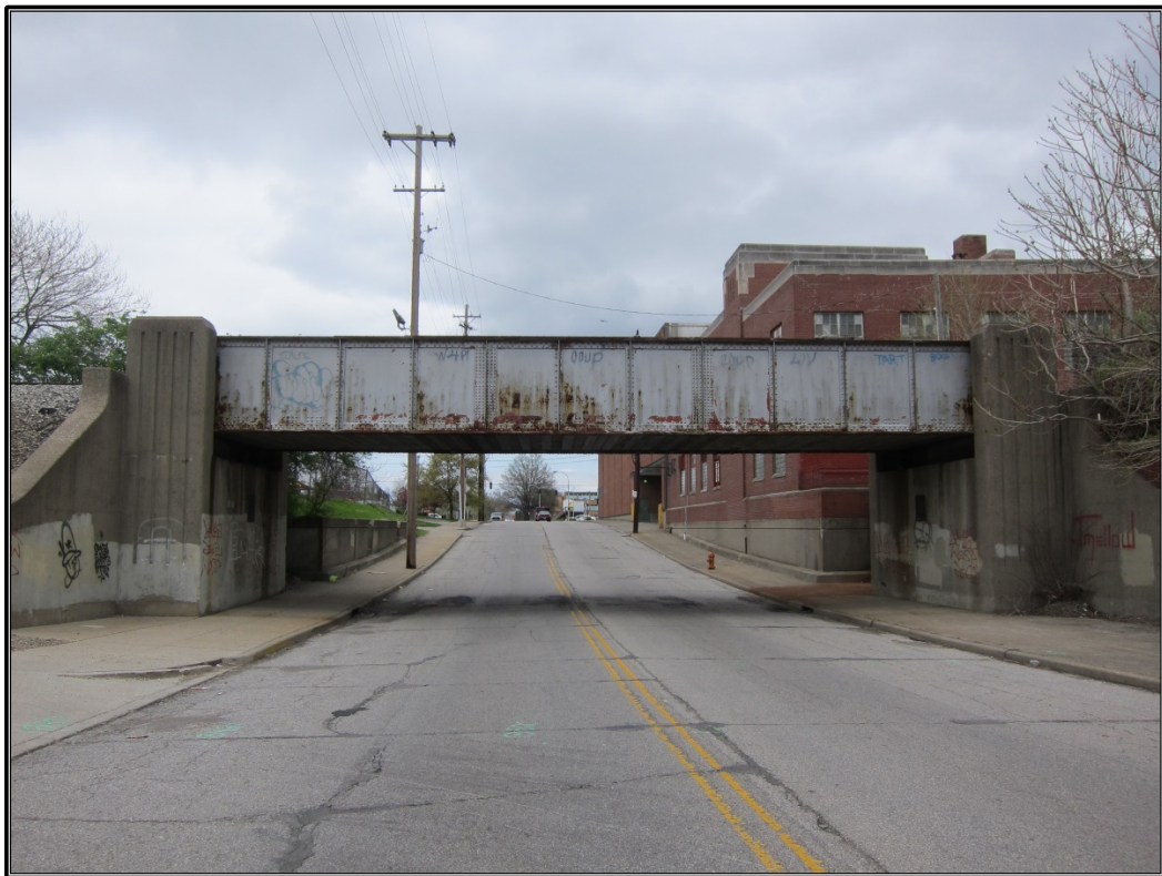
Figure 100. Site 36 (JFSW 987): Northerly view of bridge.
