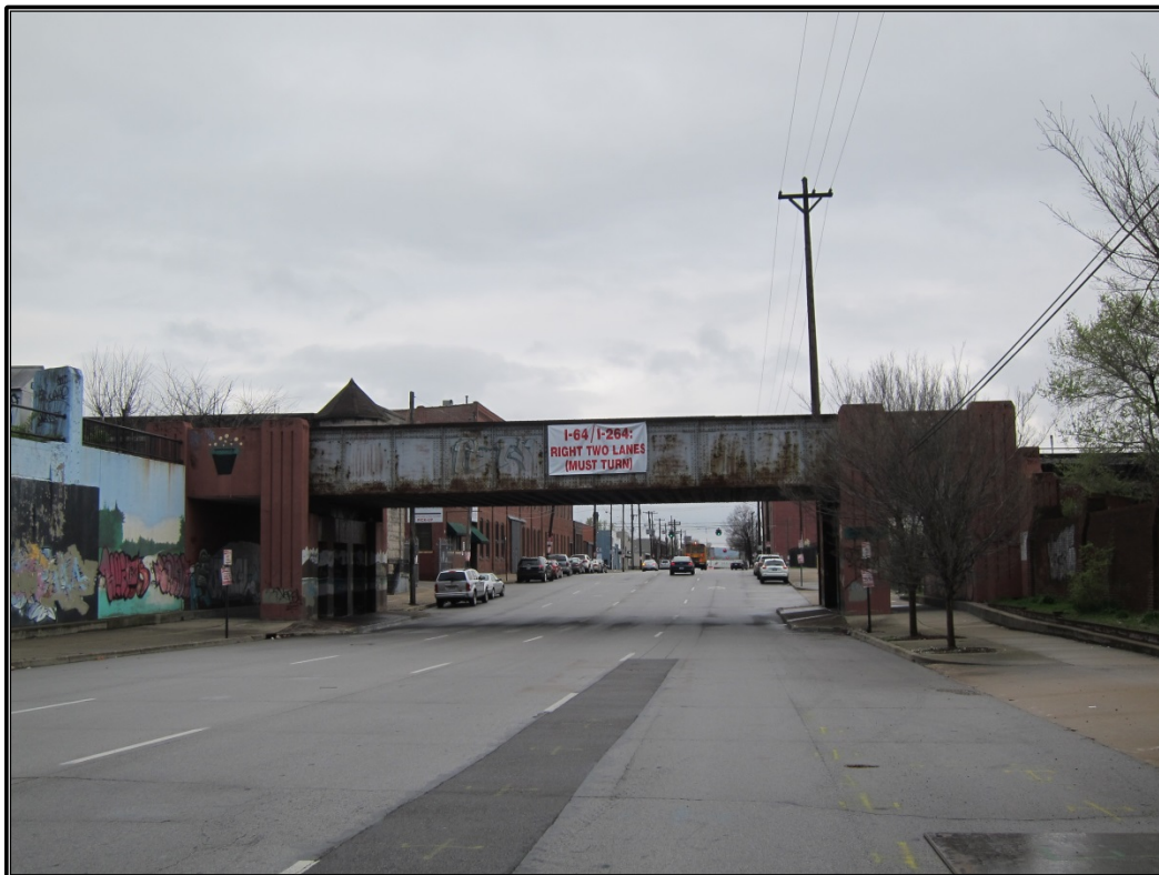
Figure 94. Site 5 (JFWP 615): Westerly view of bridge.
