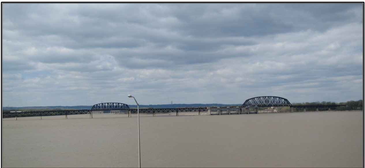
Figure 13. Site 1 (JFWP 327): Northern portion of the bridge.
