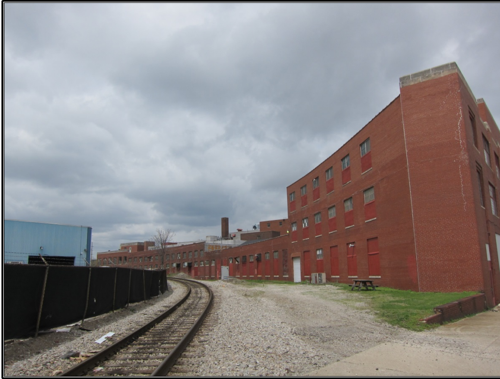
Figure 86. Site 37 (JFSW 988): South elevation of the original portion of the building.
