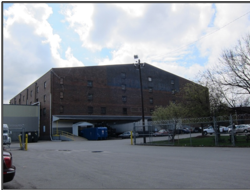
Figure 61. Site 28 (JFSW 979): Southeasterly view of Site 28.
