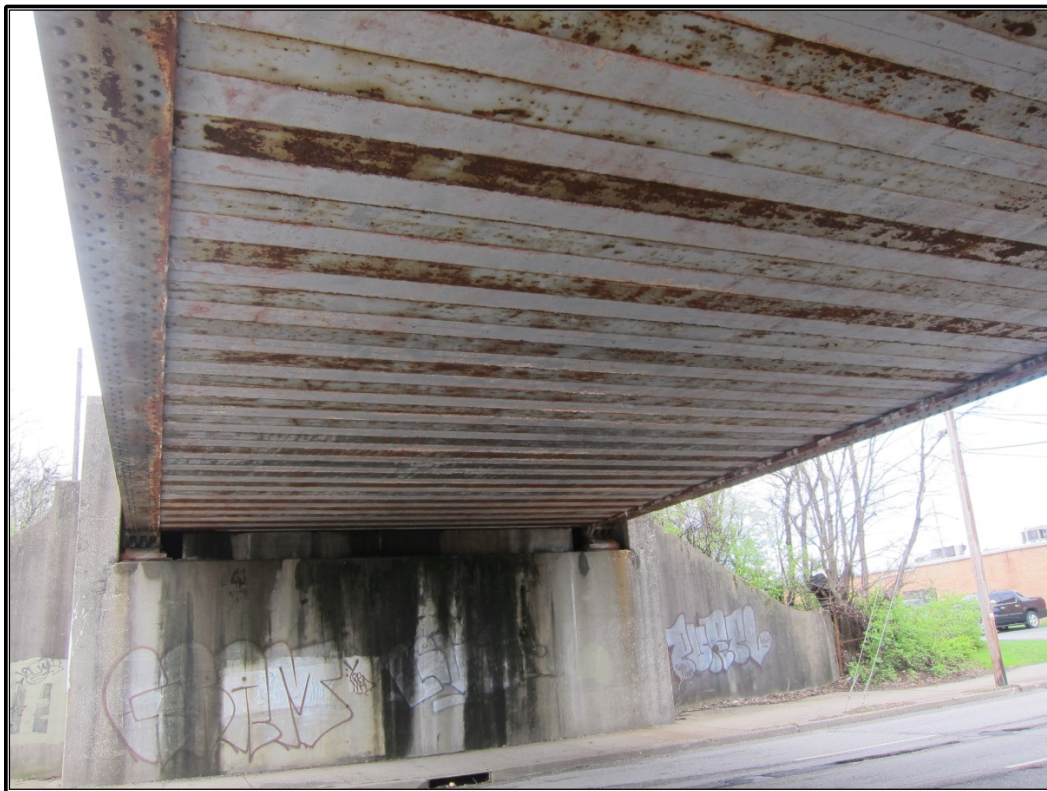
Figure 104. Site 21 (JFWR 3837): Integrated metal floor beams beneath bridge decking.
