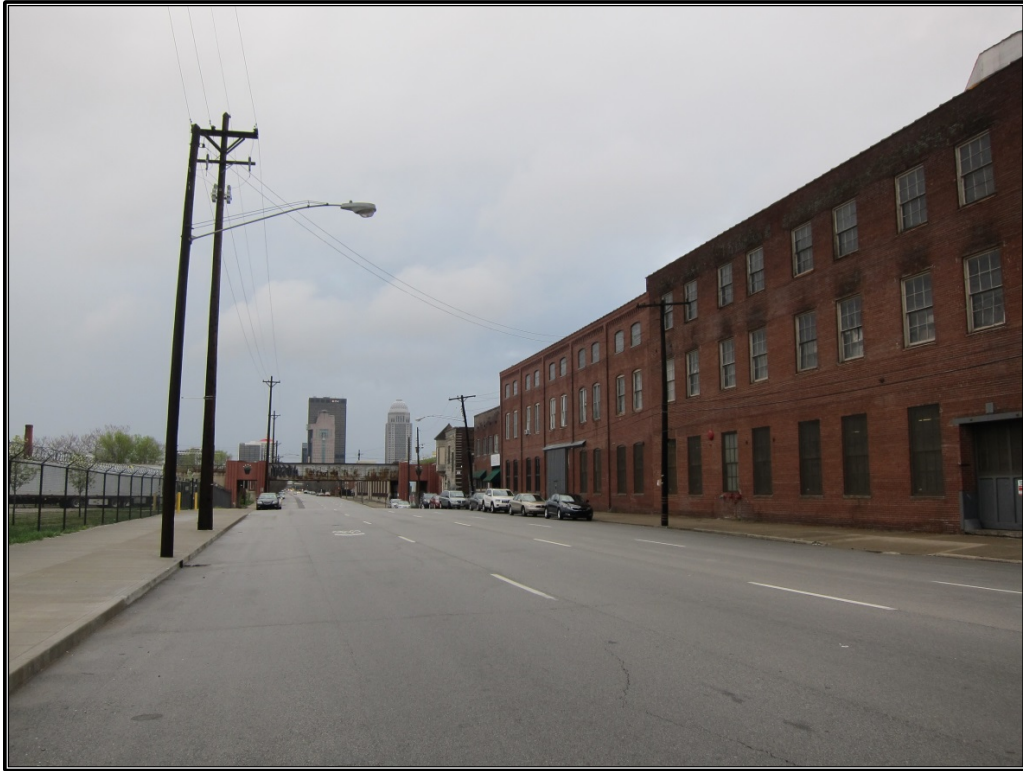
Figure 6. Overview of Main Street toward downtown Louisville from South Fifteenth Street.
