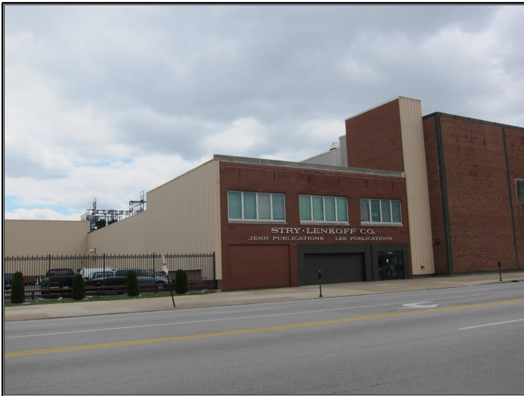
Figure 89. Site 37 (JFSW 988): One-story addition to the circa 1950–1974 portion of the building.
