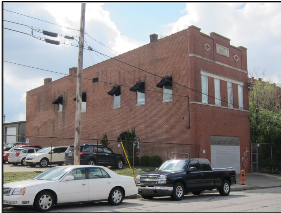
Figure 67. Site 30 (JFSW 981): Southeasterly view of Site 30.
