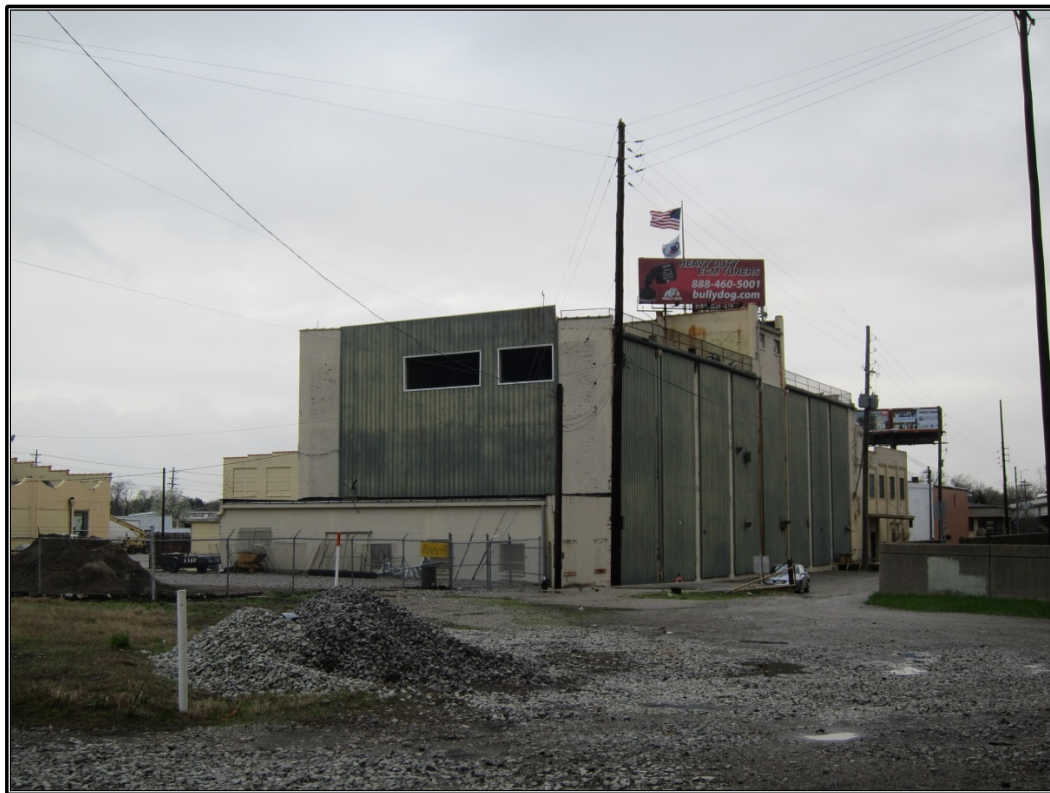
Figure 20. Site 2 (JFWP 528): Westerly view of the former shipping building.
