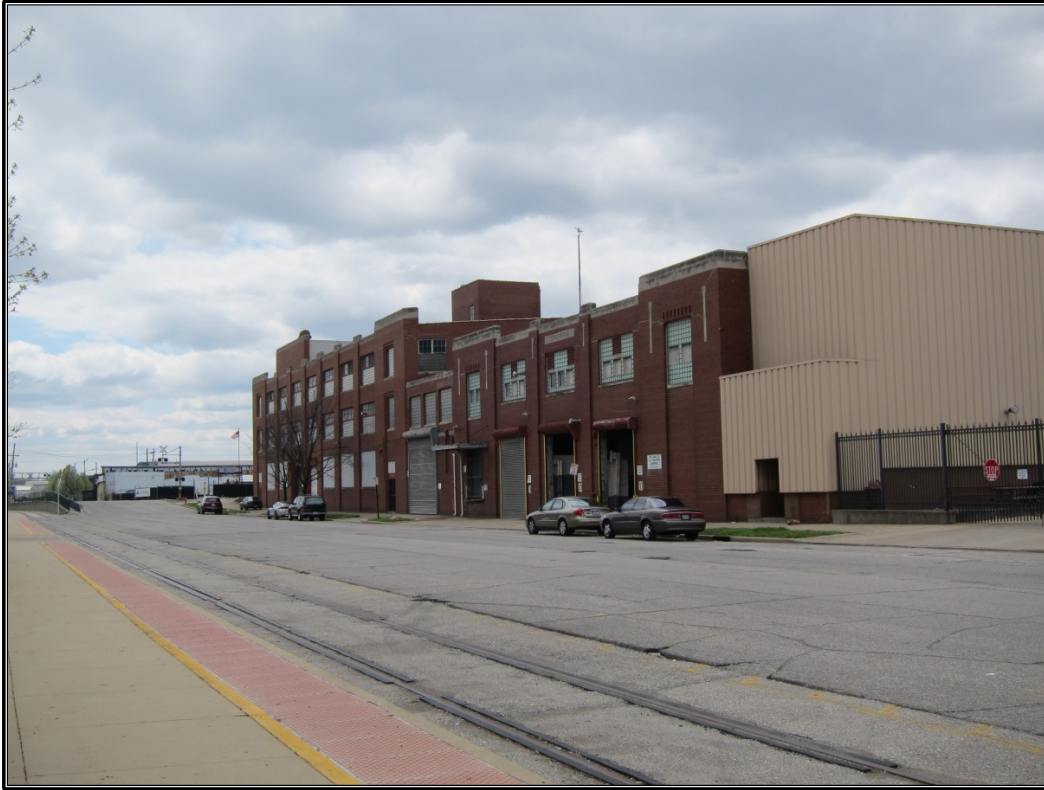
Figure 84. Site 37 (JFSW 988): Two-story section of the original portion of the building.
