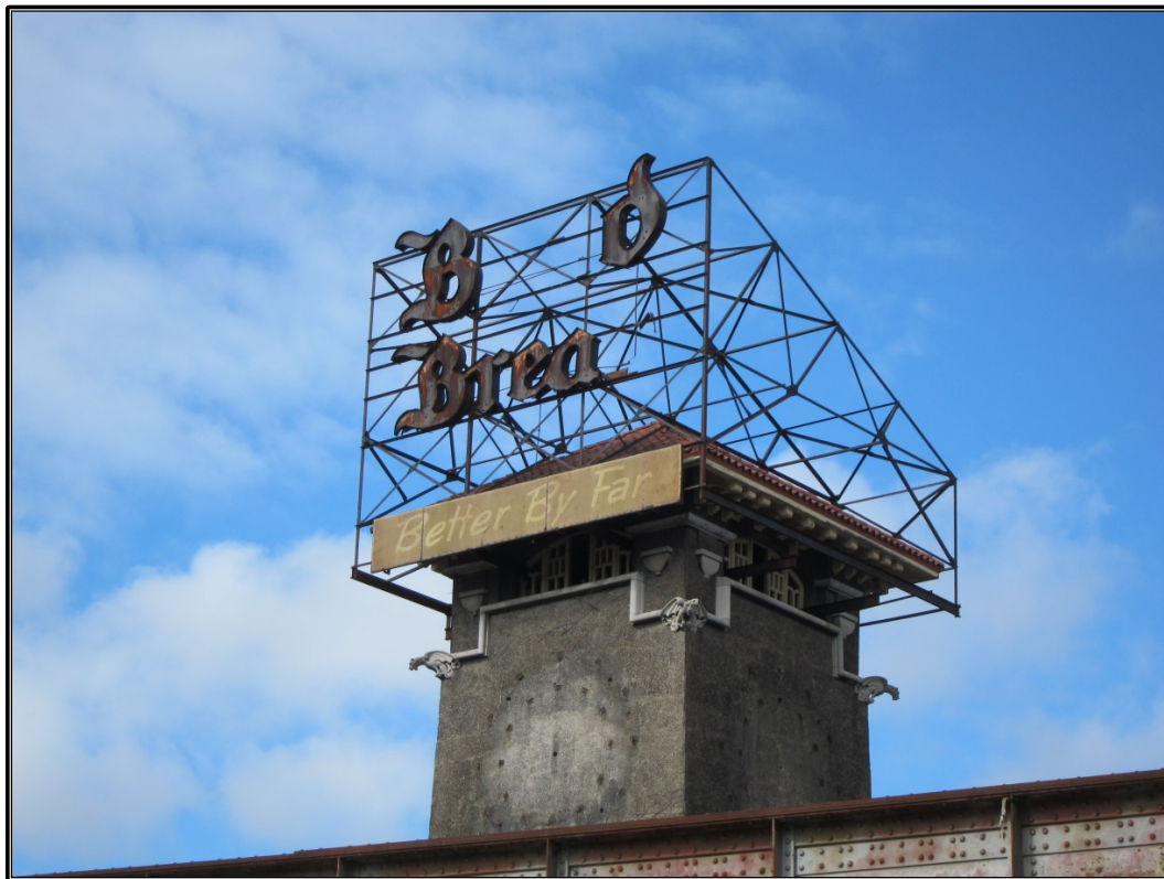
Figure 58. Site 26 (JFSW 404): Detail of eastern tower and Bond Bread sign.
