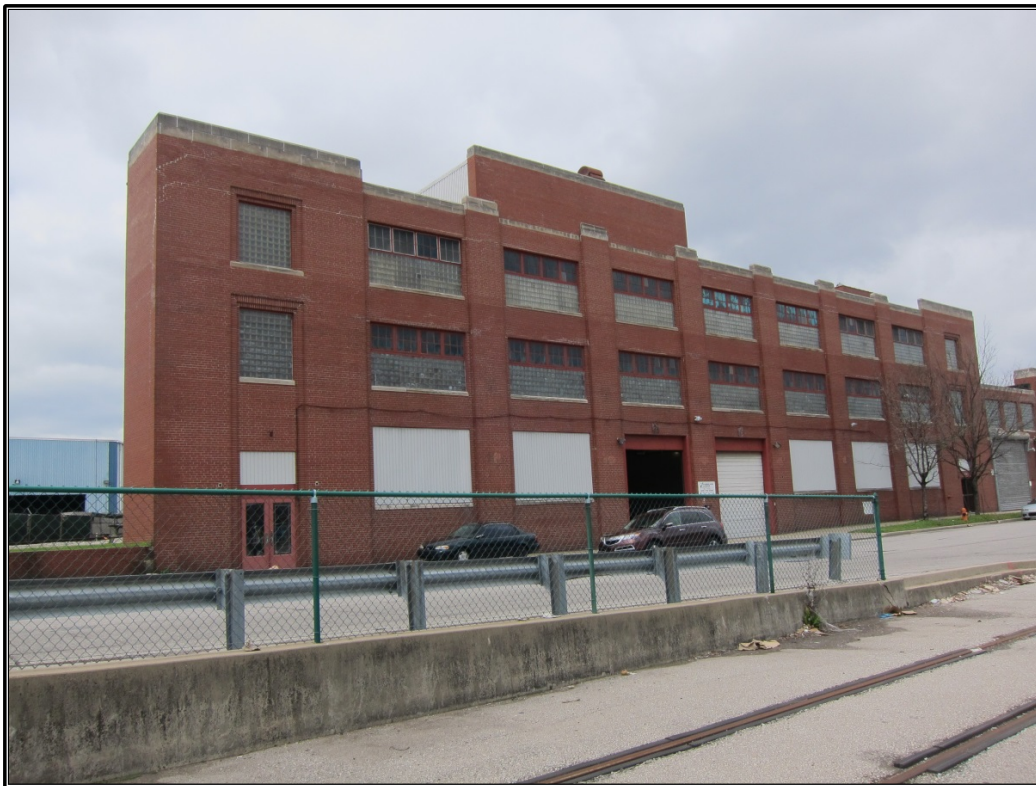
Figure 85. Site 37 (JFSW 988): Three-story section of the original portion of the building.
