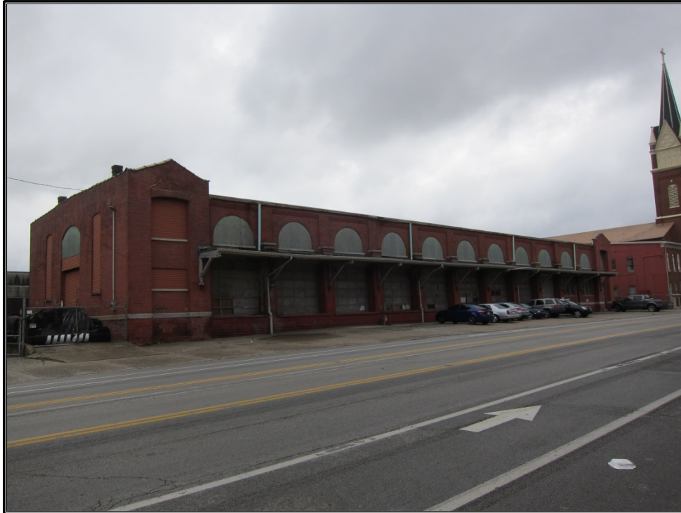
Figure 37. Site 9 (JFWR 3825): Northeasterly view of building.
