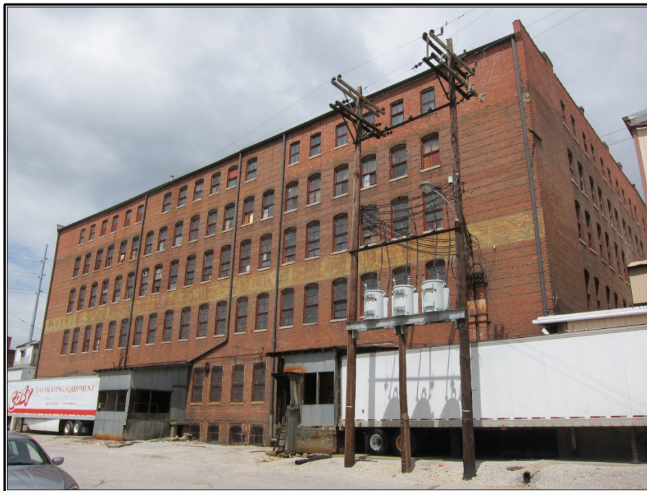
Figure 77. Site 34 (JFSW 985): Rear elevation of factory building.
