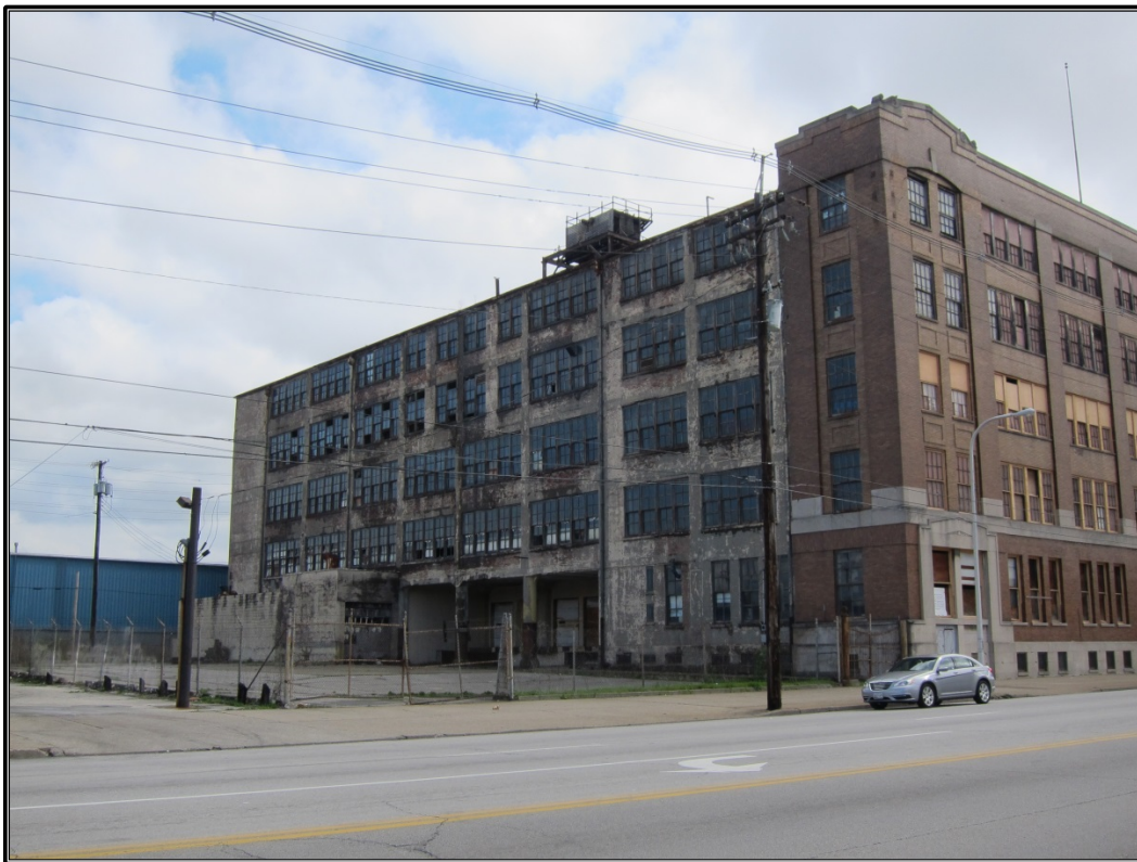
Figure 55. Site 24 (JFSW 436): West elevation.
