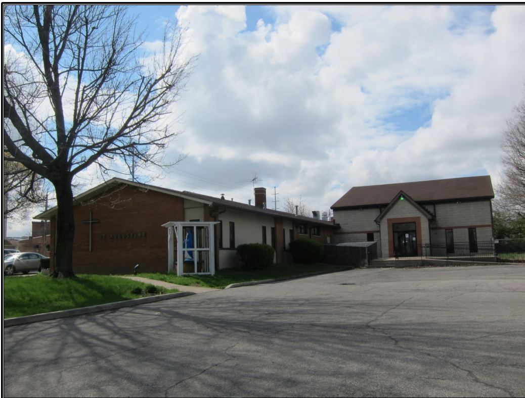
Figure 65. Site 29 (JFSW 980): Side-gabled addition.
