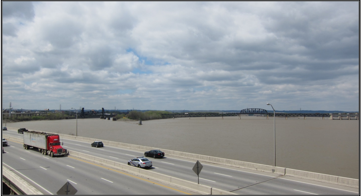
Figure 12. Site 1 (JFWP 327): Southern portion of the bridge.
