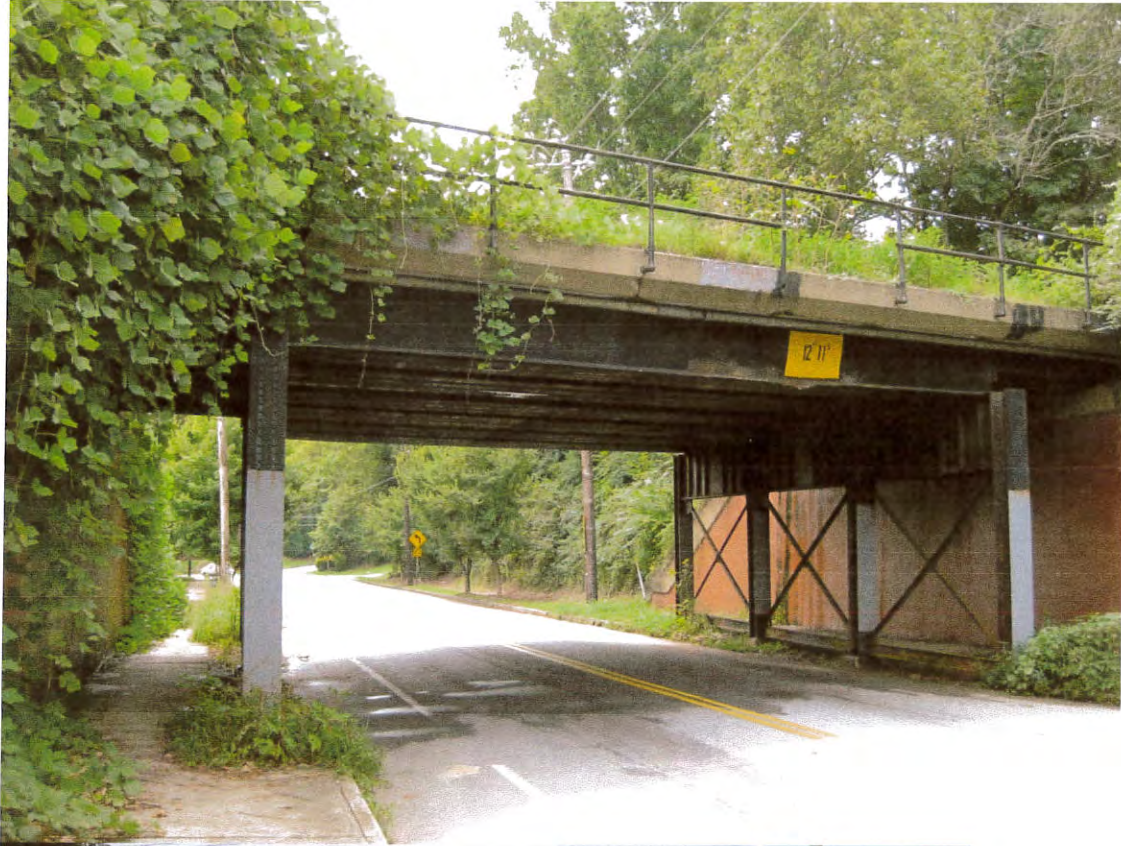
Bridge Number XXC 3.53
