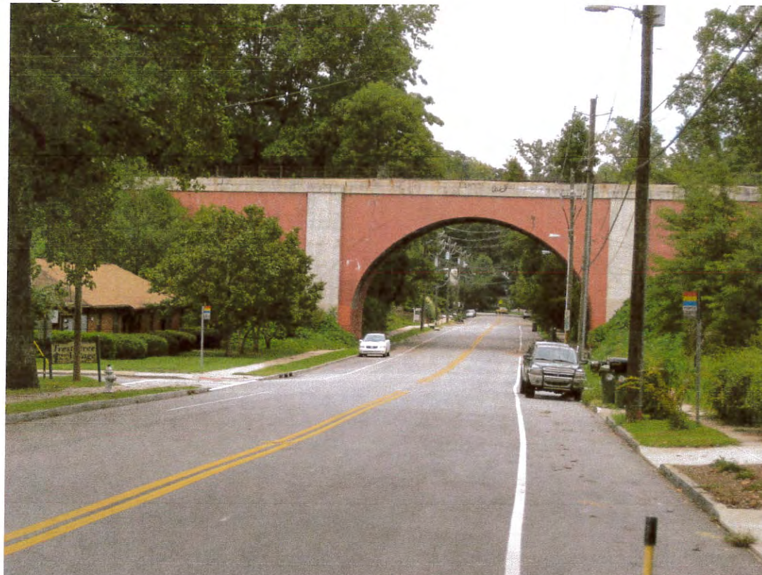
Bridge Number XXC 3.94
