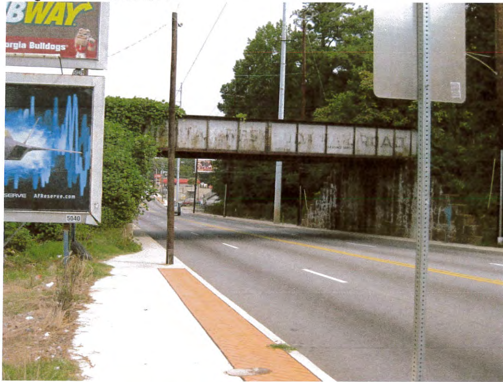
Bridge Number XXC 0.70
