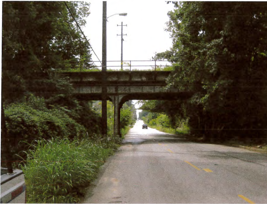
Bridge Number XXC 2.4
