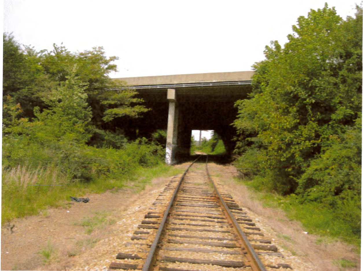
Bridge Number XXC 1.30
