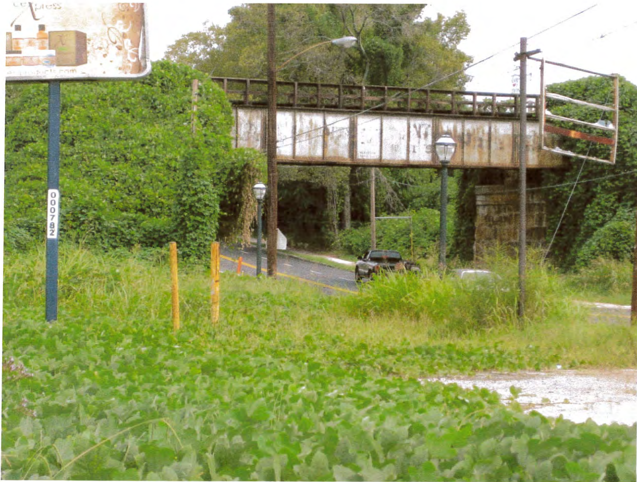
Bridge Number XXC 1.60
