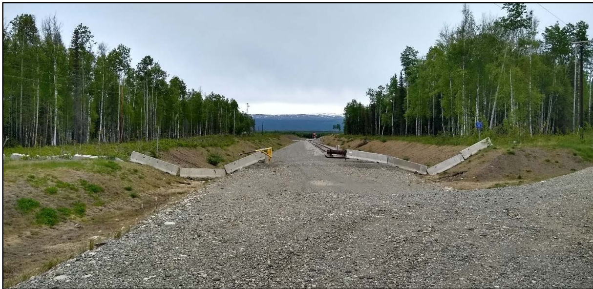
Figure 10: Millers Reach Road Crossing (Looking North)
