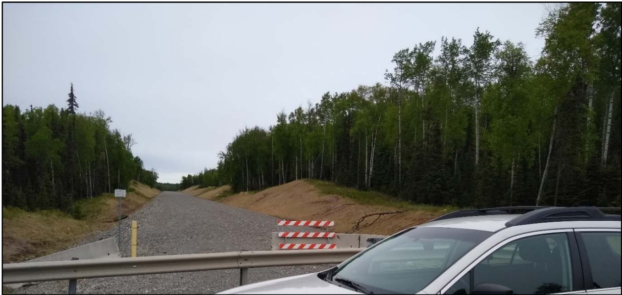
Figure 5: Susitna Parkway Crossing (Looking North)
