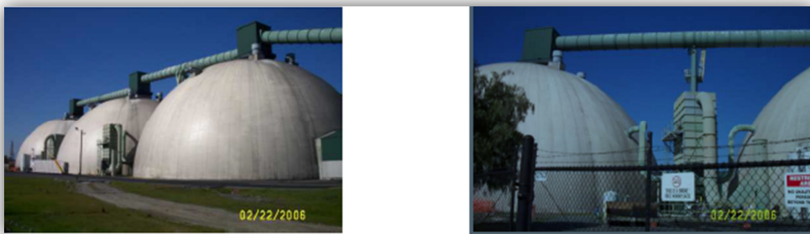
Figure 5. Photographs of the Koch Carbon, LLC Pittsburgh facility: (left) covered domes used to store piles of petcoke and (right) enclosed conveyor systems used to transfer petcoke through the facility.
