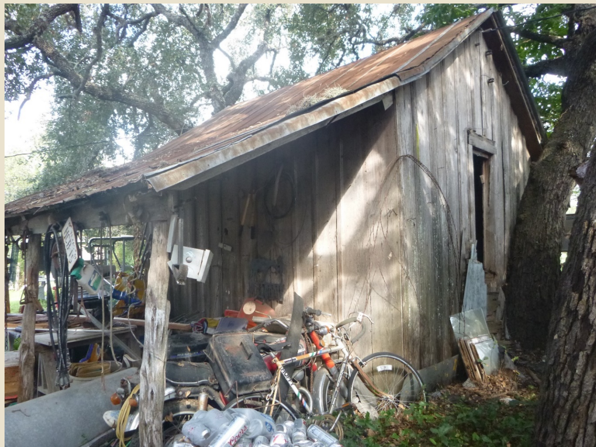
Board-and-Batten house, early 20 th century (HDR-AR-04C)
