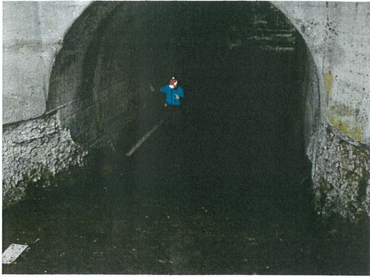
Culvert Beneath EJFE TRAILS.
