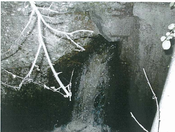
CLOSE UP OF D.S. END OF WEIR
