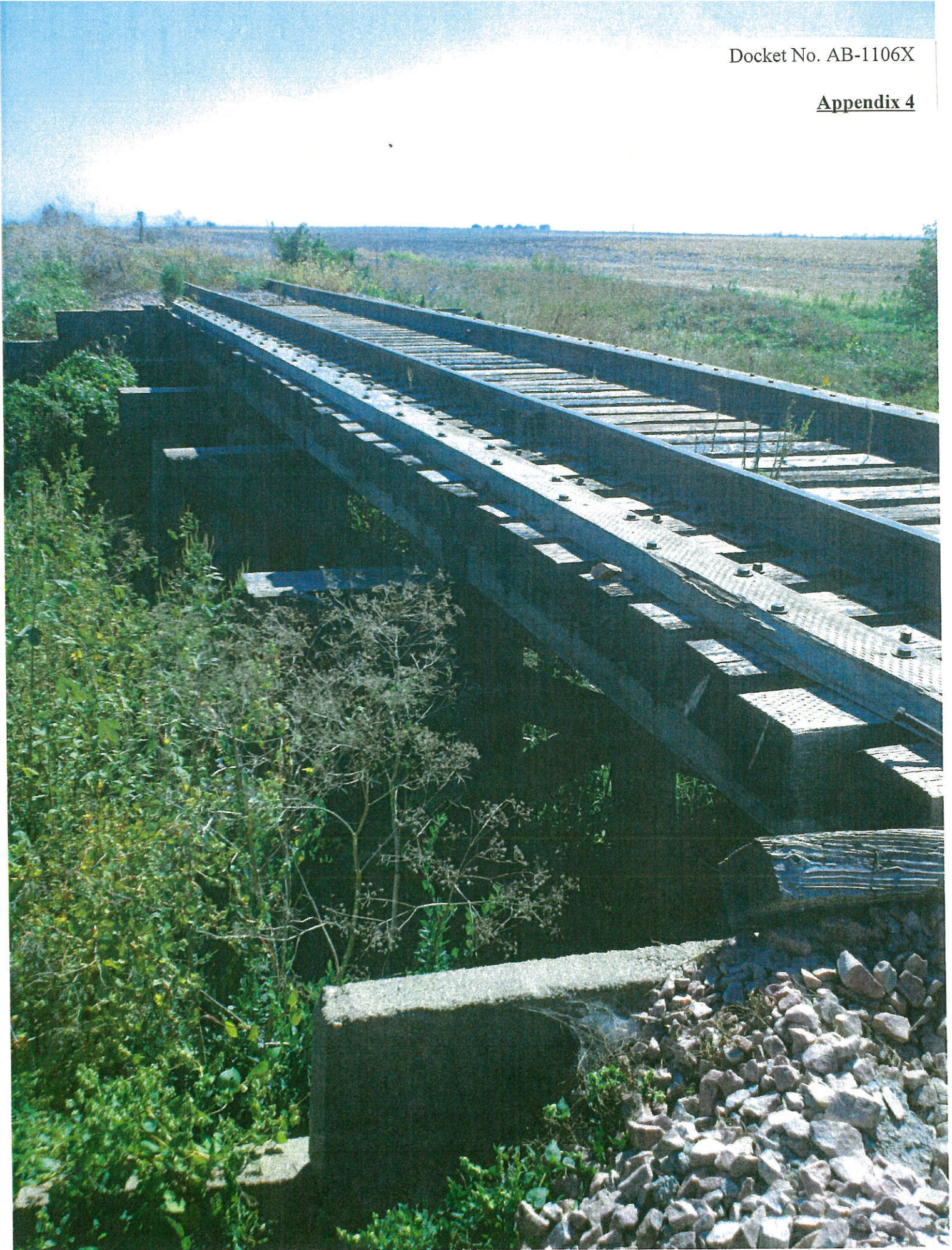
Bridge over Indian Creek in south half of rail line looking SSW
