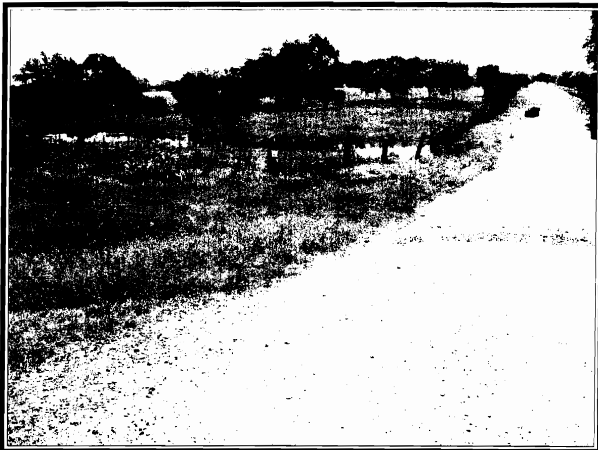
CR 450 and FM 2676 Flood Damage Aftermath
