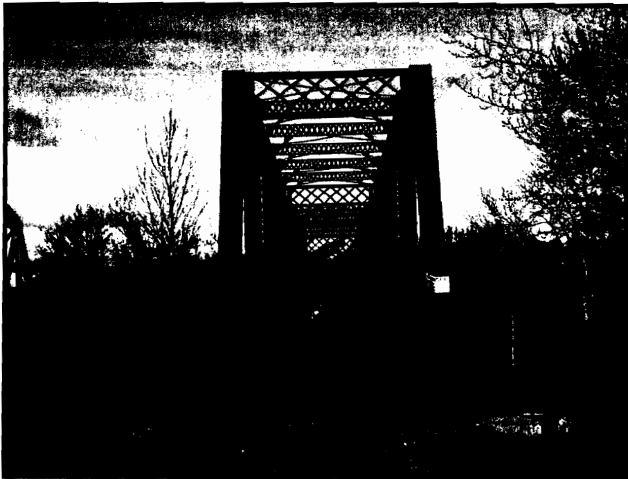
Figure 5. Naches River Bridge No. 41, eastern approach.
