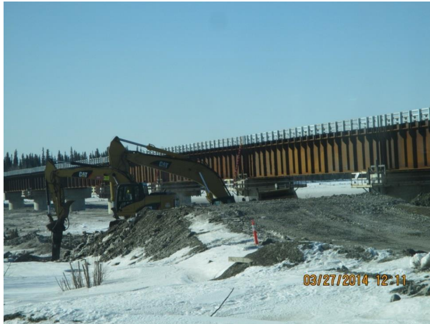
Figure 4. Causeway Removal, March 2014.
