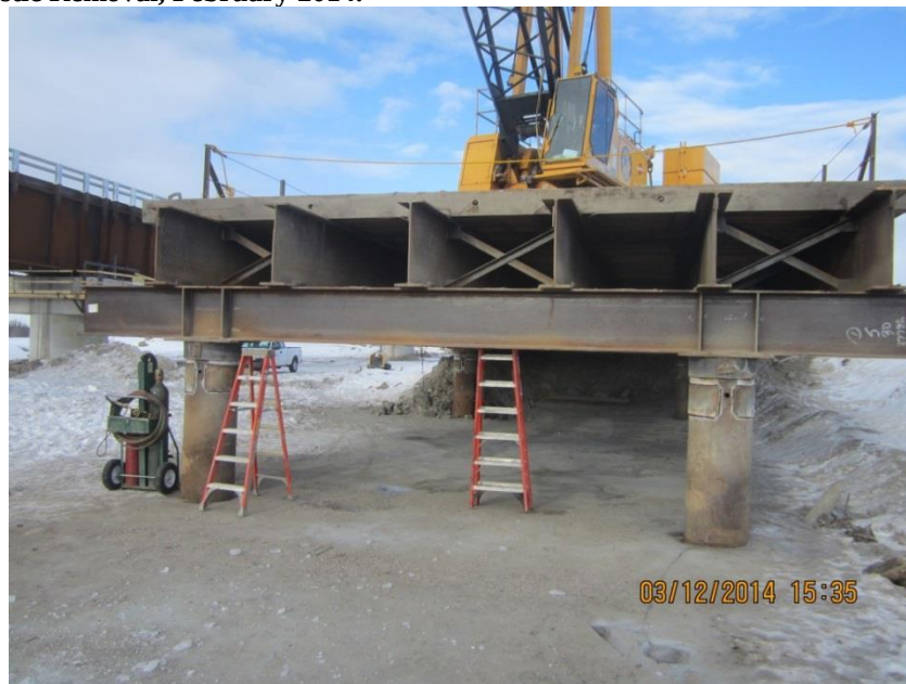
Figure 3. Trestle and Pile Removal, March 2014.
