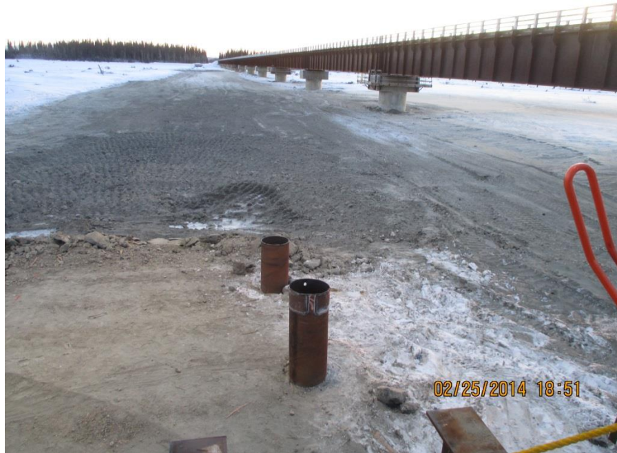
Figure 2. Trestle Removal, February 2014.
