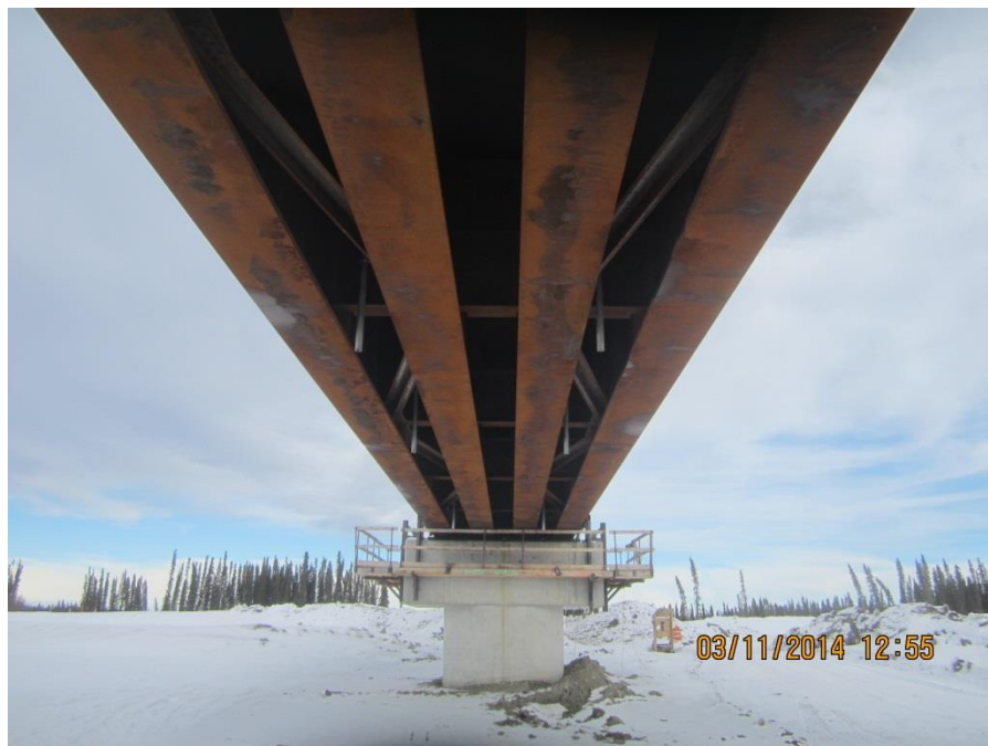
Figure 1. Girder Construction, March 2014
