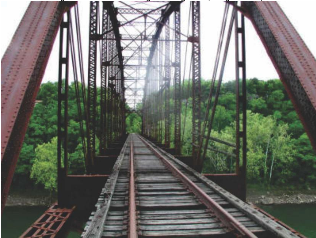
Figure 47: Deck of Bridge, Facing East (Baughn 2014)
