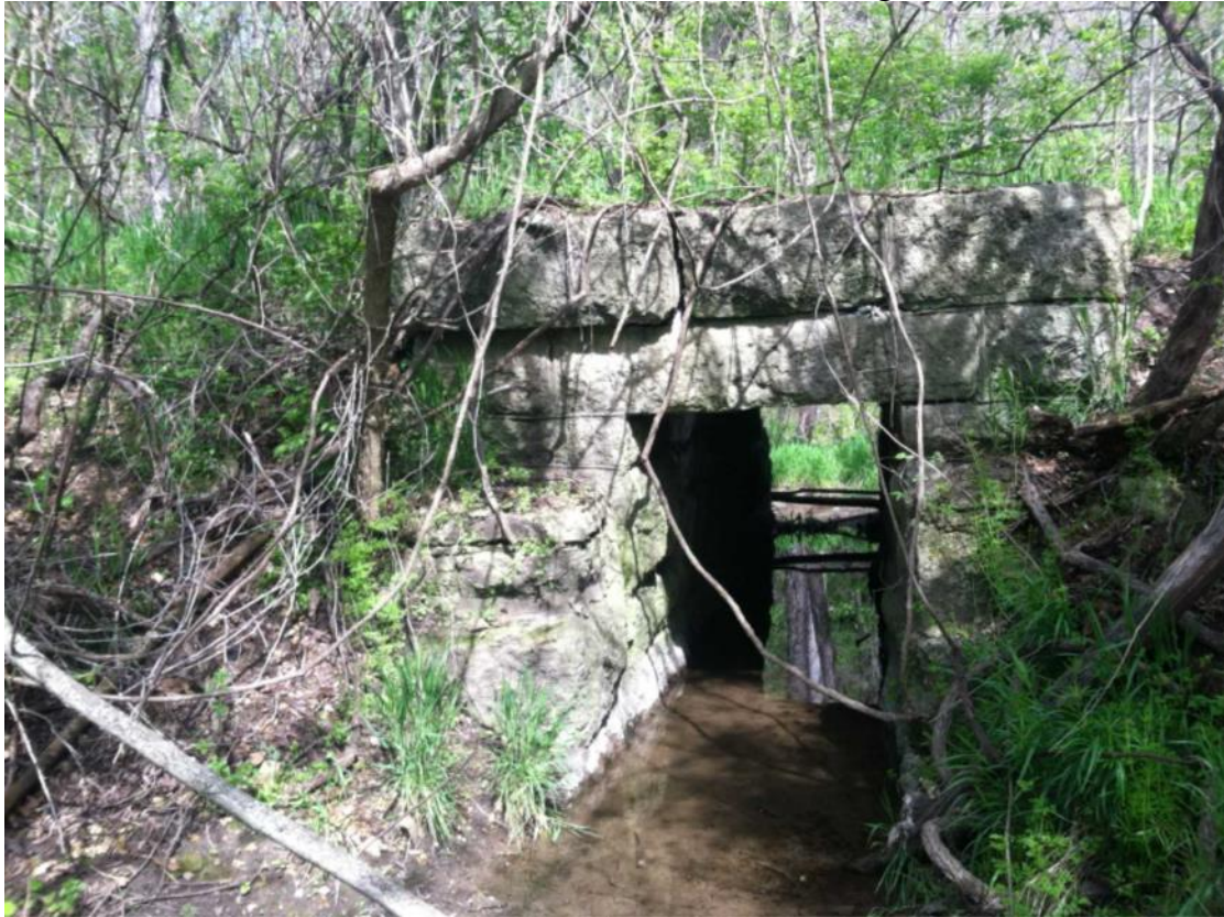
Photo 44: Culvert 135.18, Stone Box, Facing North
