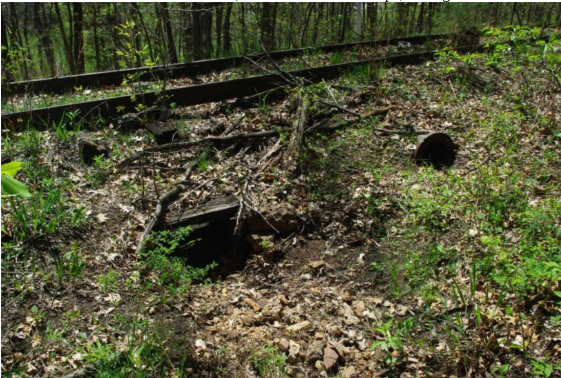
Photo 52: Culvert 132.10, Wood Box and Iron Pipe, Facing South
