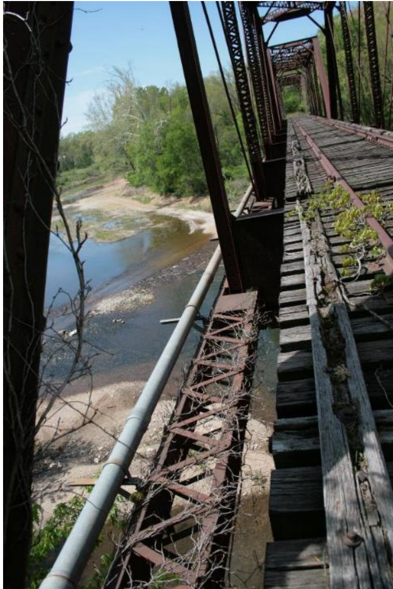
Photo 119: Bridge 121.50, Closeup of Modern Pipe Line along Side, Facing Southwest
