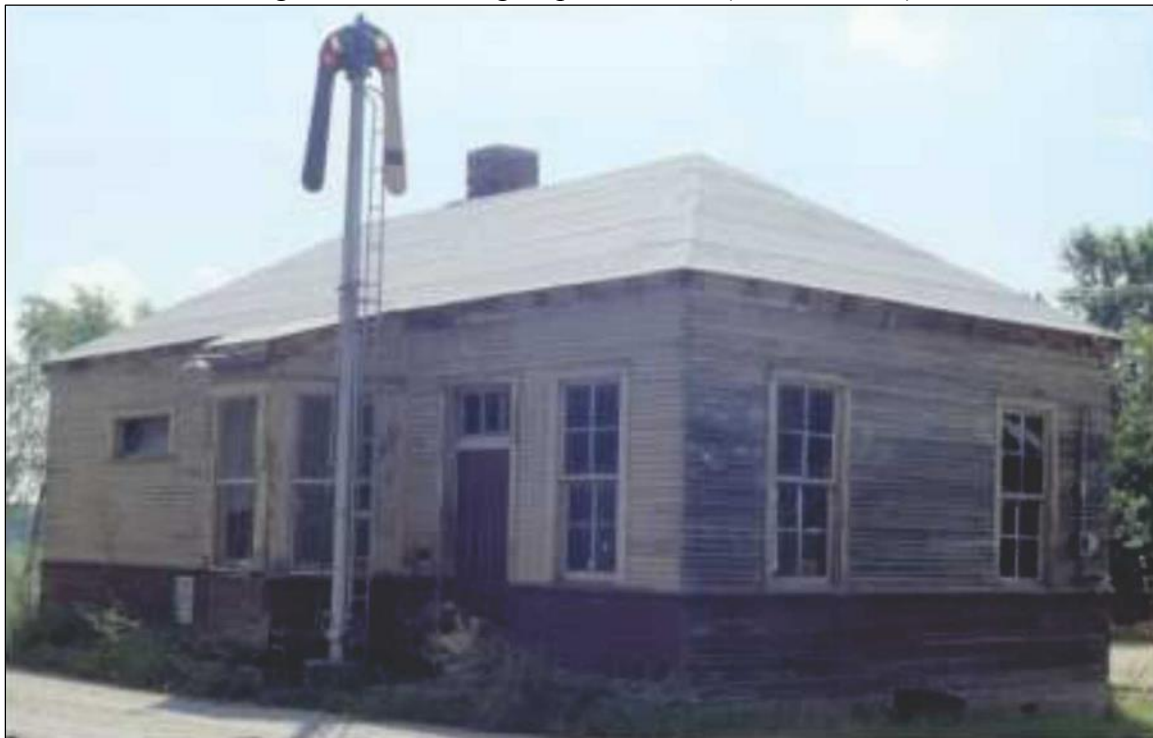
Figure 25: Freeburg Depot ca. 1980 (Forbes 2005c)
