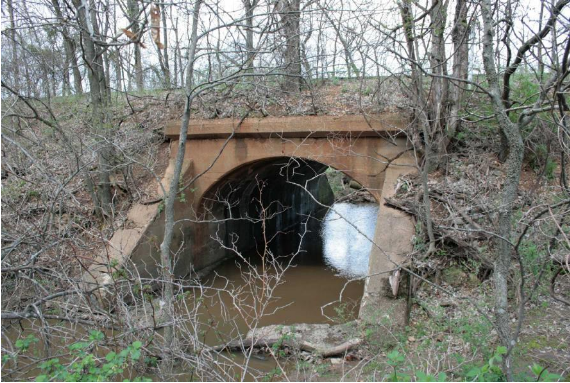
Photo 67: Culvert 179.70, Concrete Arch, Facing South
