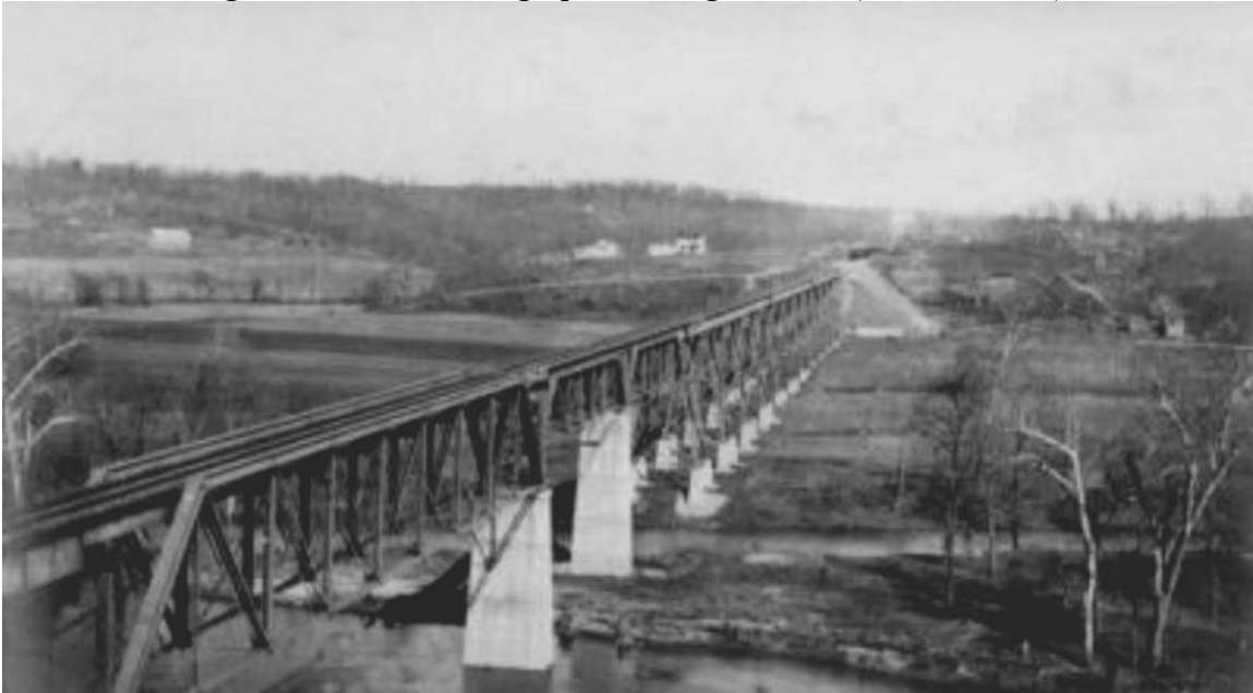
Figure 45: 1906 Photograph of Bridge 114.70 (Morrow 2004)
