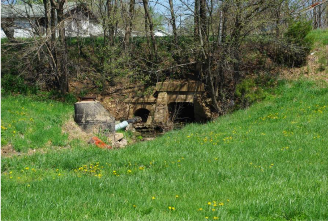
Photo 75: Double Culverts 185.85, Concrete Arch and Box, Facing North
