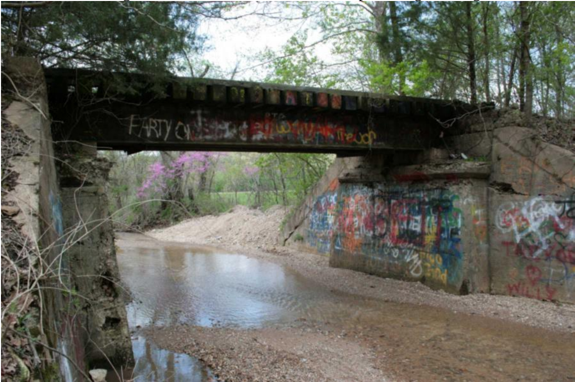
Photo 87: Bridge 137.70, Deck Beam Continuous Span Bridge, Facing Southwest
