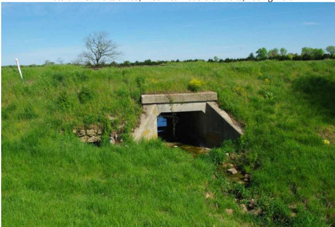
Photo 61: Culverts 92.83, Modified Double Culverts, Facing North
