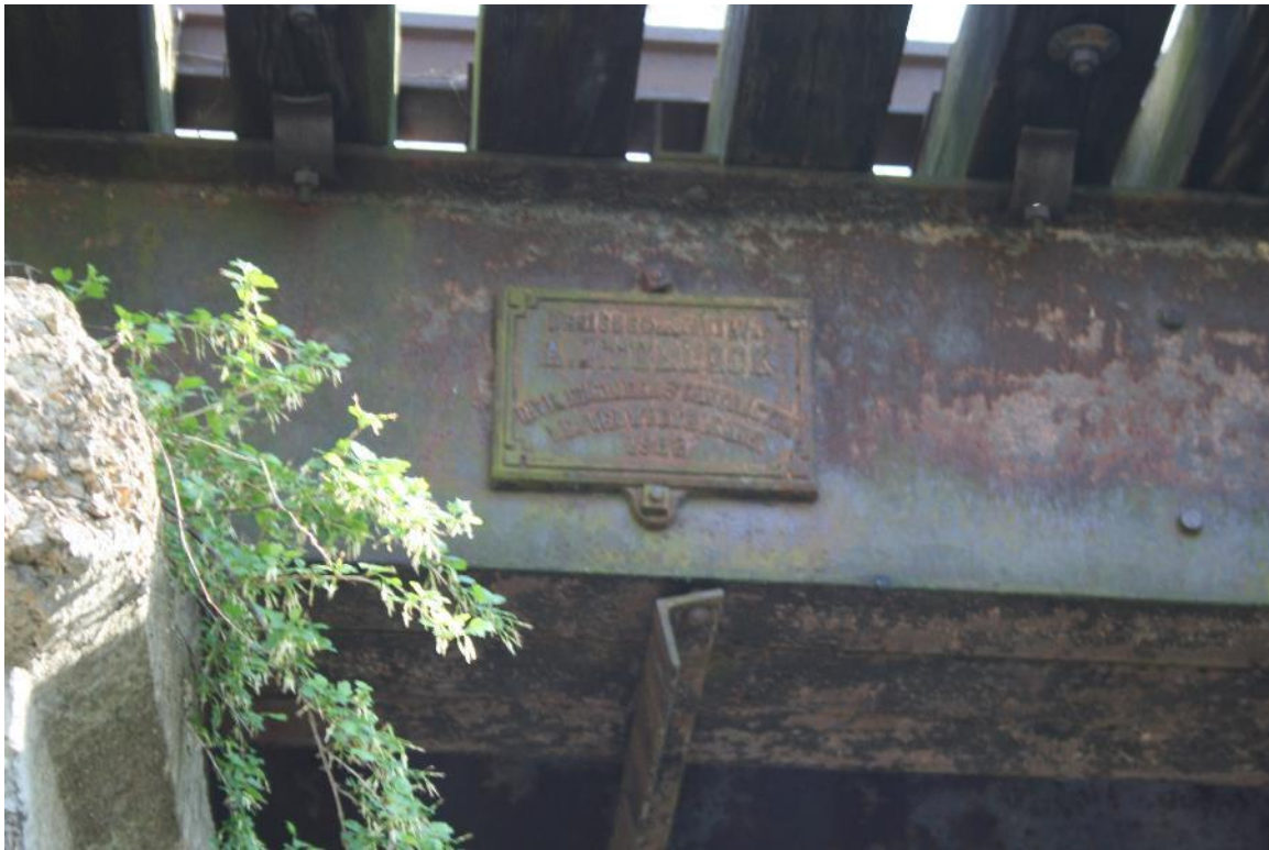
Photo 88: Bridge 126.20, Closeup of Plaque, Facing Southwest
