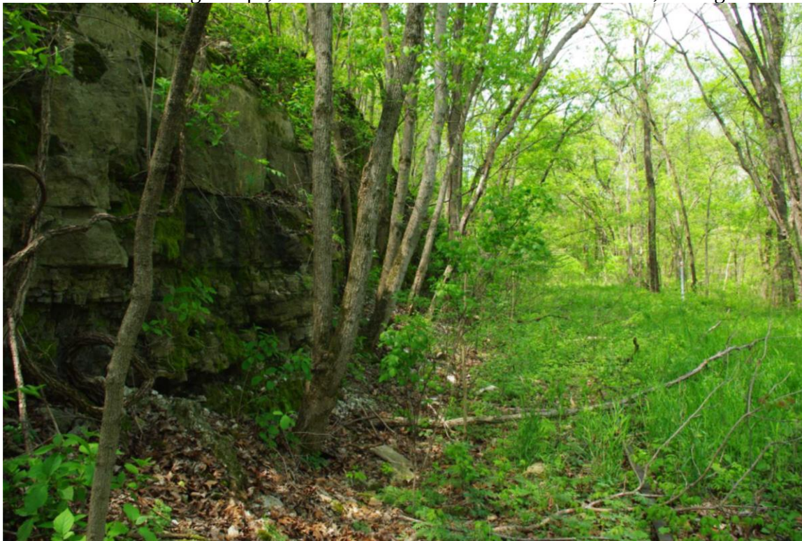
Photo 1: Cut Ridge Slope, between Mile Markers 140.00 and 141.00, Facing West
