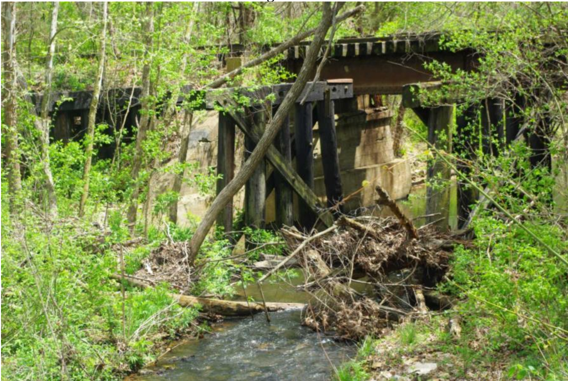
Photo 112: Bridge 144.90, Deck Beam Bridge and Wood Piers of Absent Bridge 114.90A, Facing Southeast
