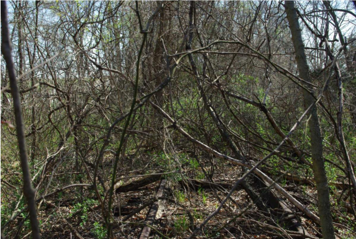
Photo 8: Trees and Brush over Rail Corridor, between Mile Markers 184.00 and 185.00, Facing East
