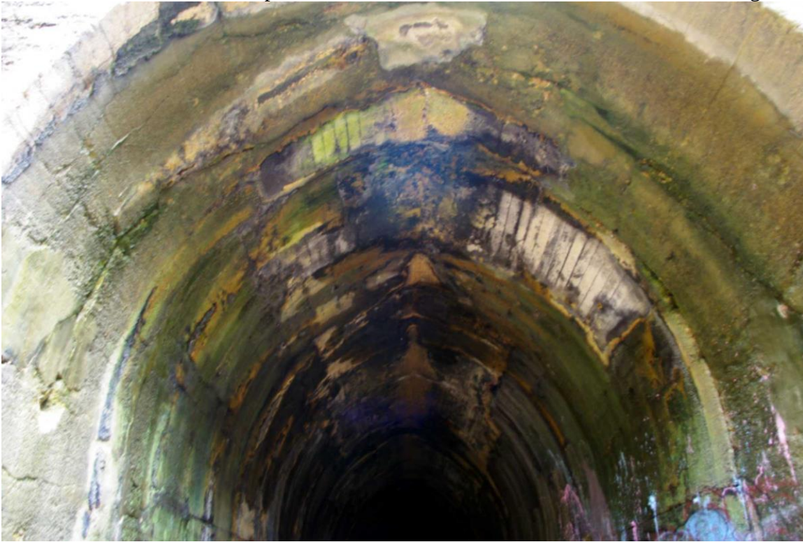
Photo 136: Tunnel 3, Closeup of Board Formed Concrete Gothic Arch Roof, Facing East
