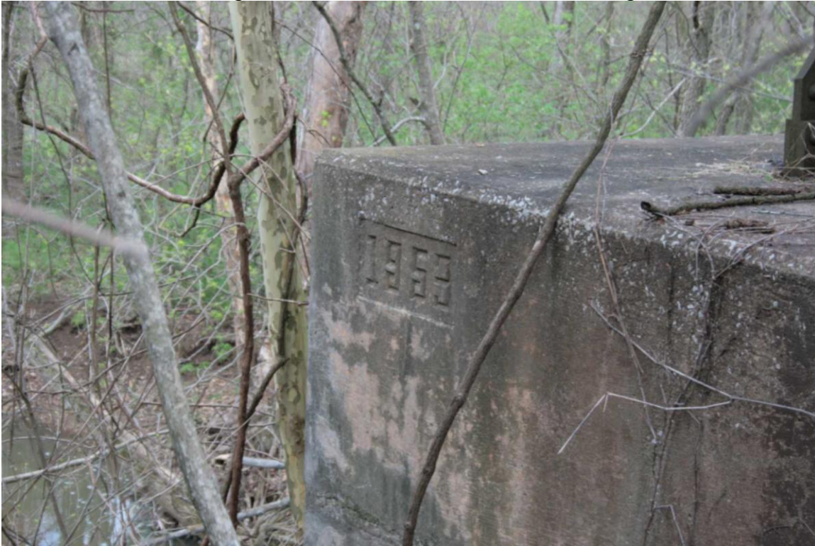
Photo 108: Bridge 162.70, Date “1953” on East Pier, Facing Southwest
