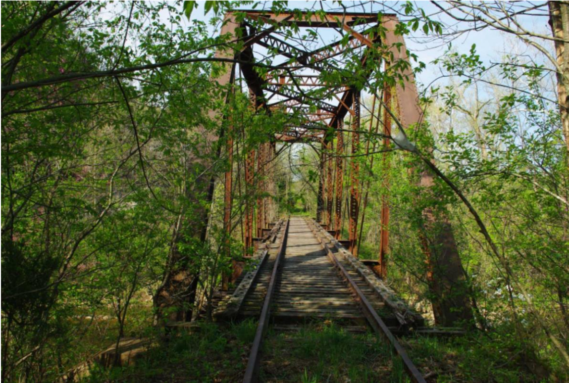
Photo 120: Bridge 135.53, Pratt Through Truss Deck, Facing West
