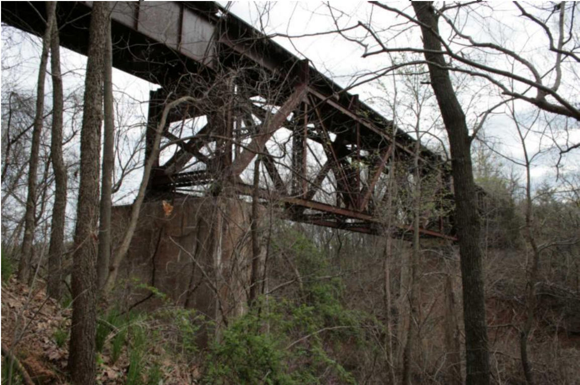
Photo 105: Bridge 189.75, Pratt Deck Truss Continuous Span, Facing Northeast
