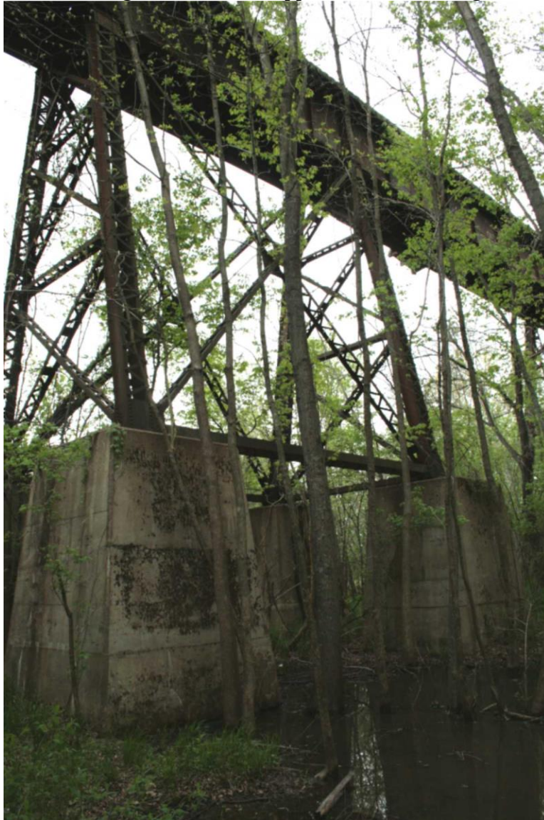
Photo 125: Bridge 143.33, East Approach Piers, Facing Southwest
