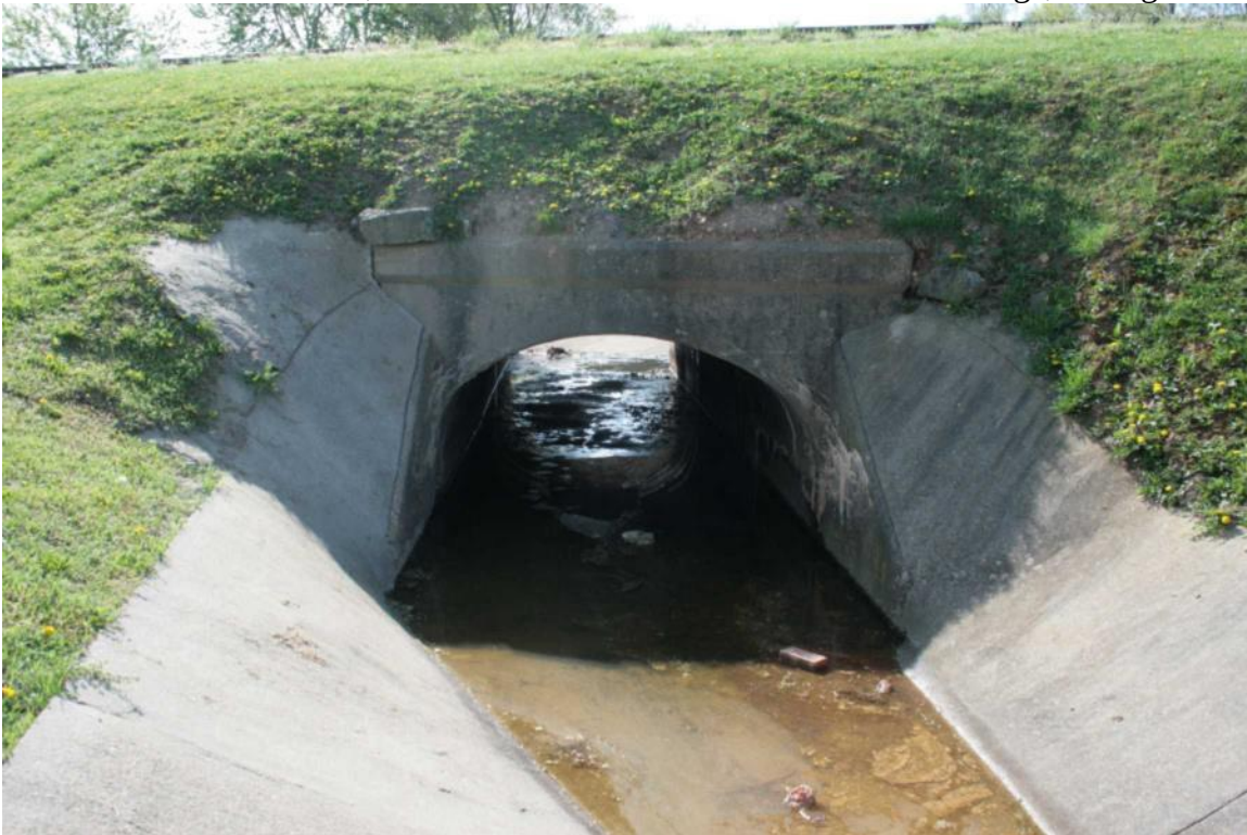
Photo 74: Culvert 177.85, Concrete Arch with Modern Concrete Drainage, Facing South
