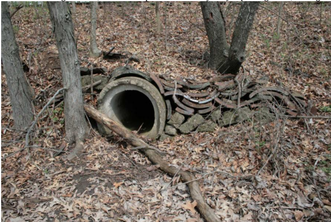
Photo 77: Drainage 173.39, Concrete Pipe Surrounded by Clay Pipe Fragments, Facing East
