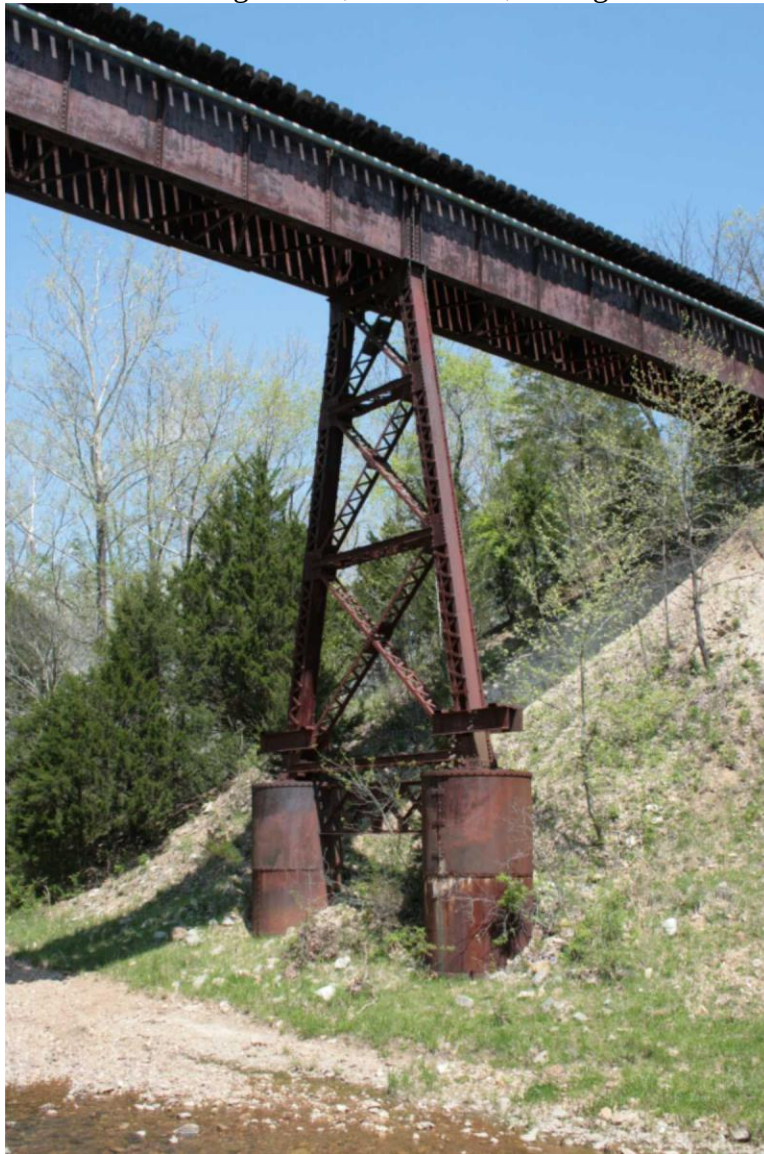
Photo 94: Bridge 86.95, Metal Piers, Facing Northeast
