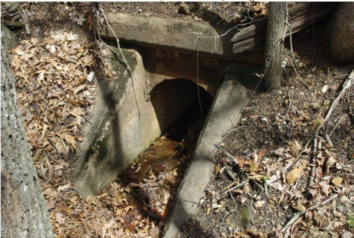
Photo 68: Culvert 193.60, Concrete Arch, Facing Northwest
