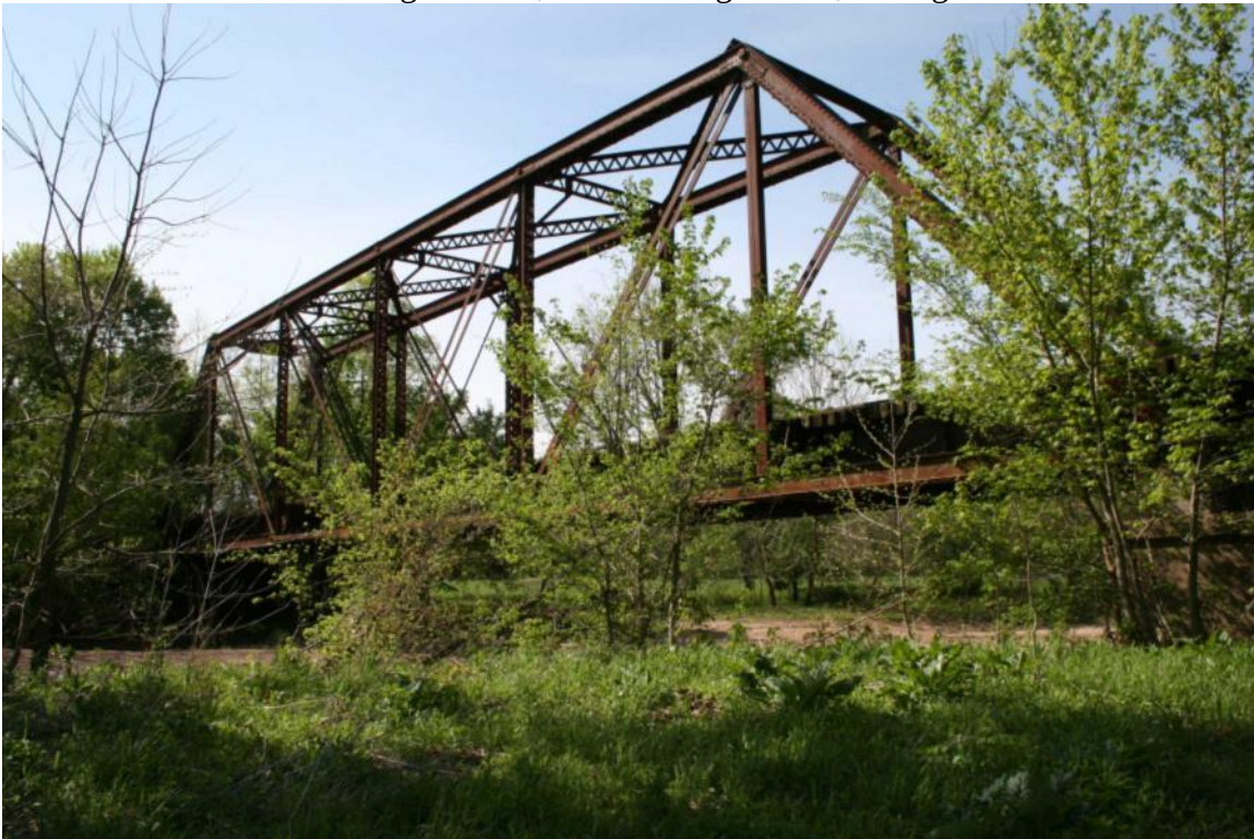
Photo 116: Bridge 137.05, Pratt Through Truss, Facing Southeast
