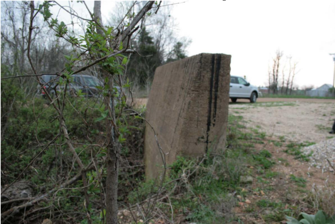
Photo 131: Bridge 165.65, Concrete Abutment for Bridge over Beacon Street in Barnett, Facing North
