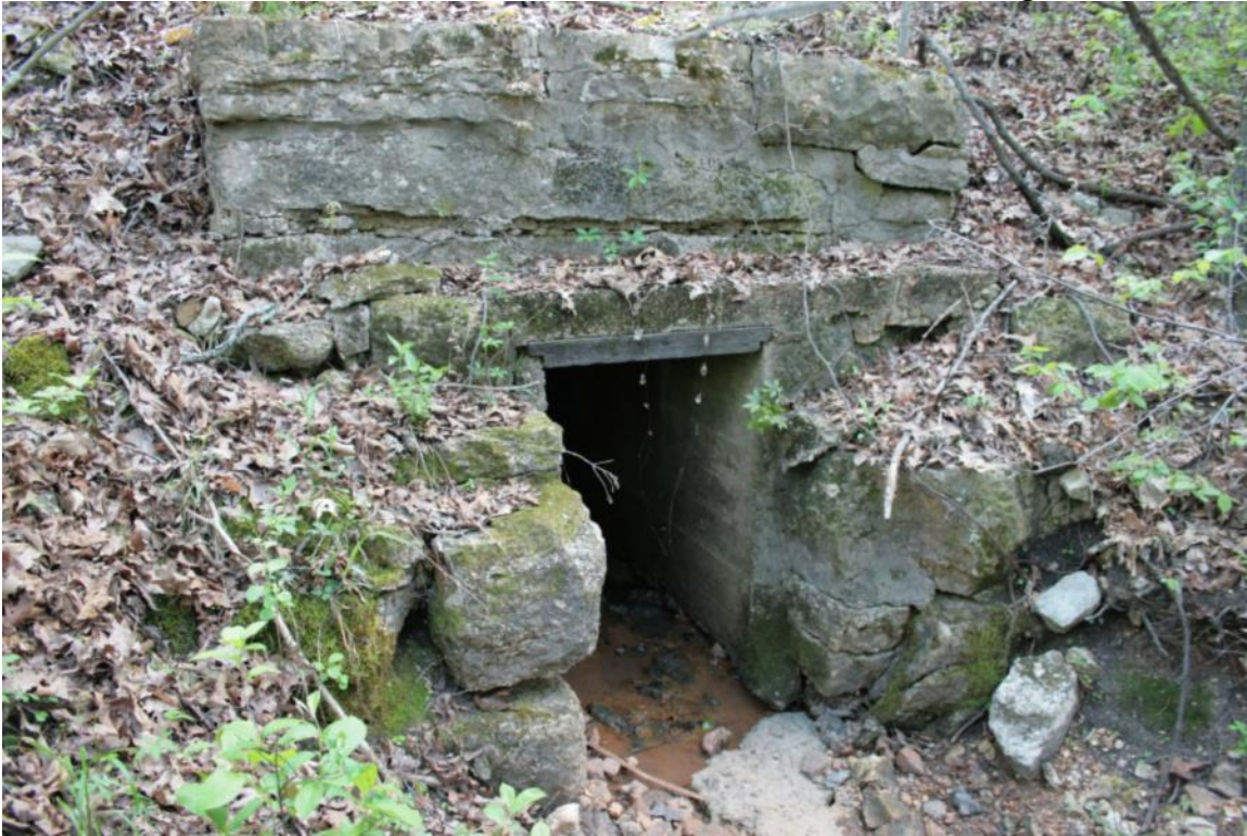
Photo 59: Culvert 86.00, Stone Box with Concrete Insert, Facing South
