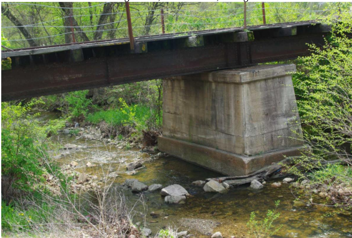
Photo 92: Bridge 134.8, Concrete Pier, Facing Southwest
