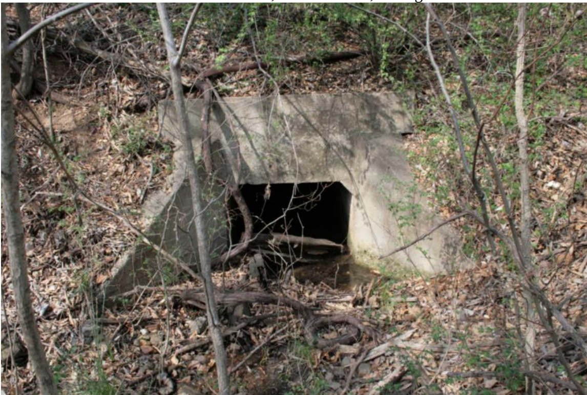
Photo 46: Culvert 170.35, Concrete Box, Facing Northeast
