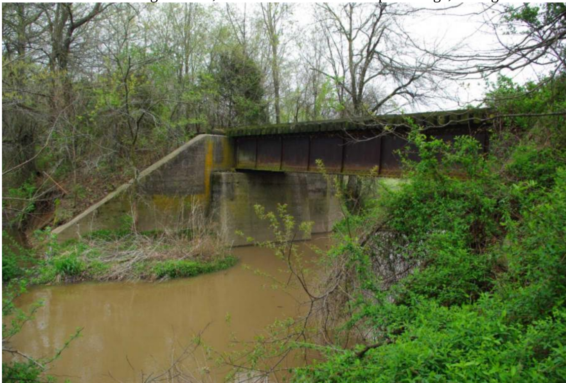
Photo 91: Bridge 210.55, Deck Plate Continuous Span Bridge, Facing Southeast
