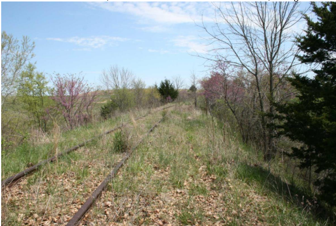
Photo 3: Clear Tracks, between Mile Markers 130.00 and 131.00, Facing East
