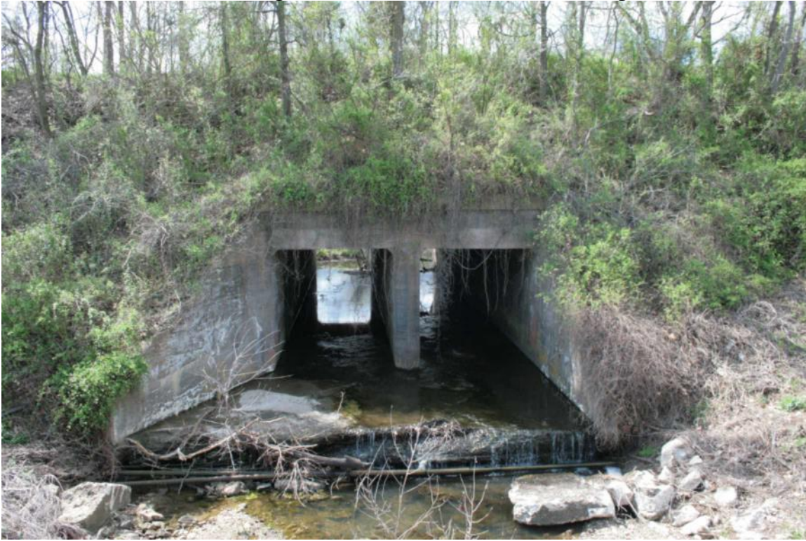
Photo 128: Bridge 155.20, Double Box Culvert, Facing Northwest
