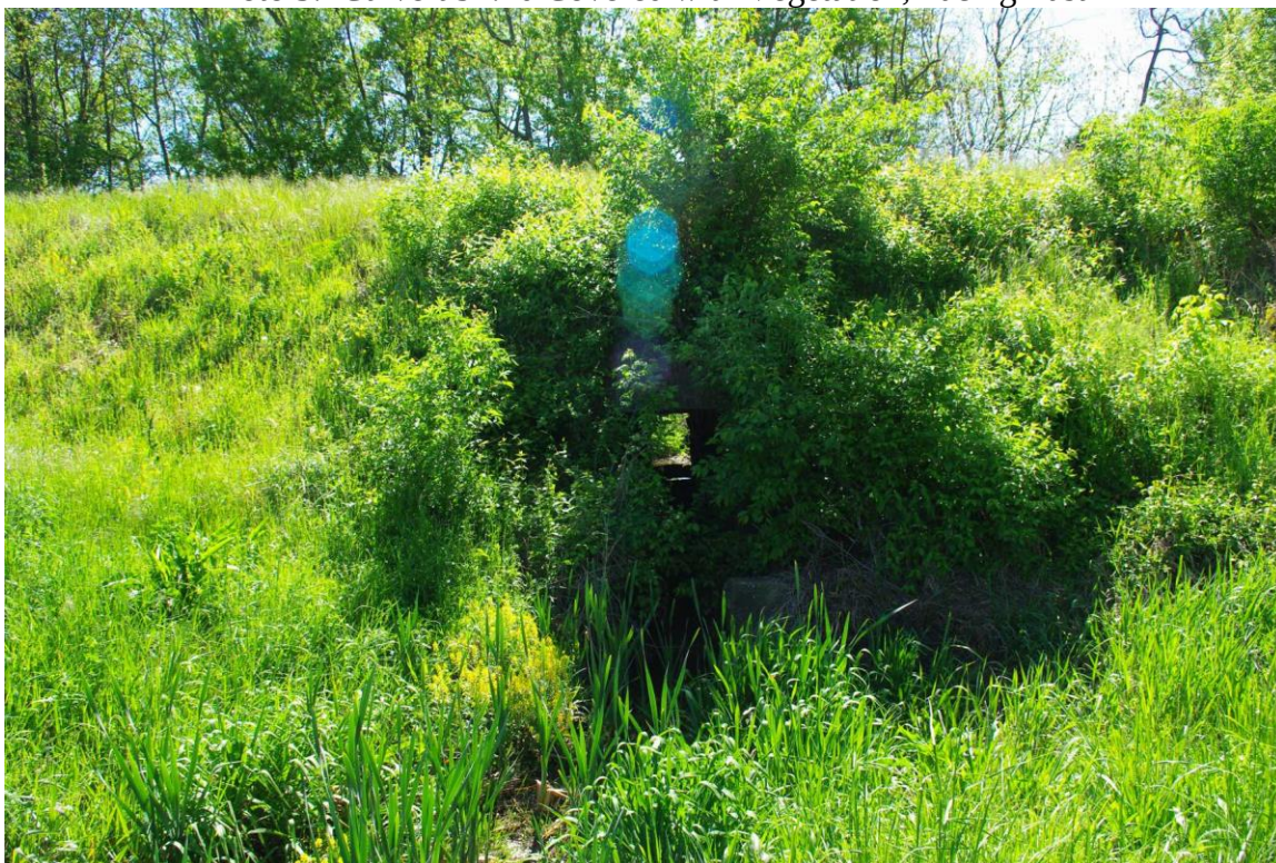
Photo 5: Culvert 91.10 Covered with Vegetation, Facing East
