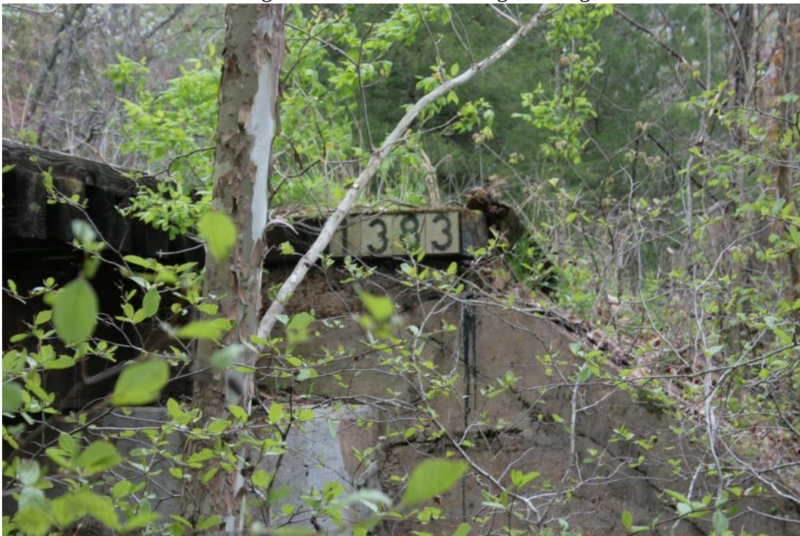
Photo 89: Bridge 138.35, Mile Marker Sign, Facing Northeast
