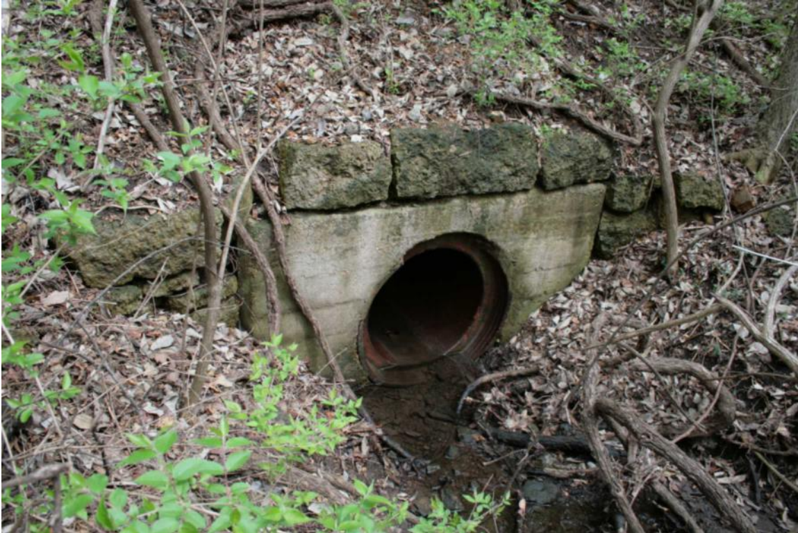
Photo 78: Drainage 160.65, Single Concrete Block with Stone and Clay Pipe, Facing North
