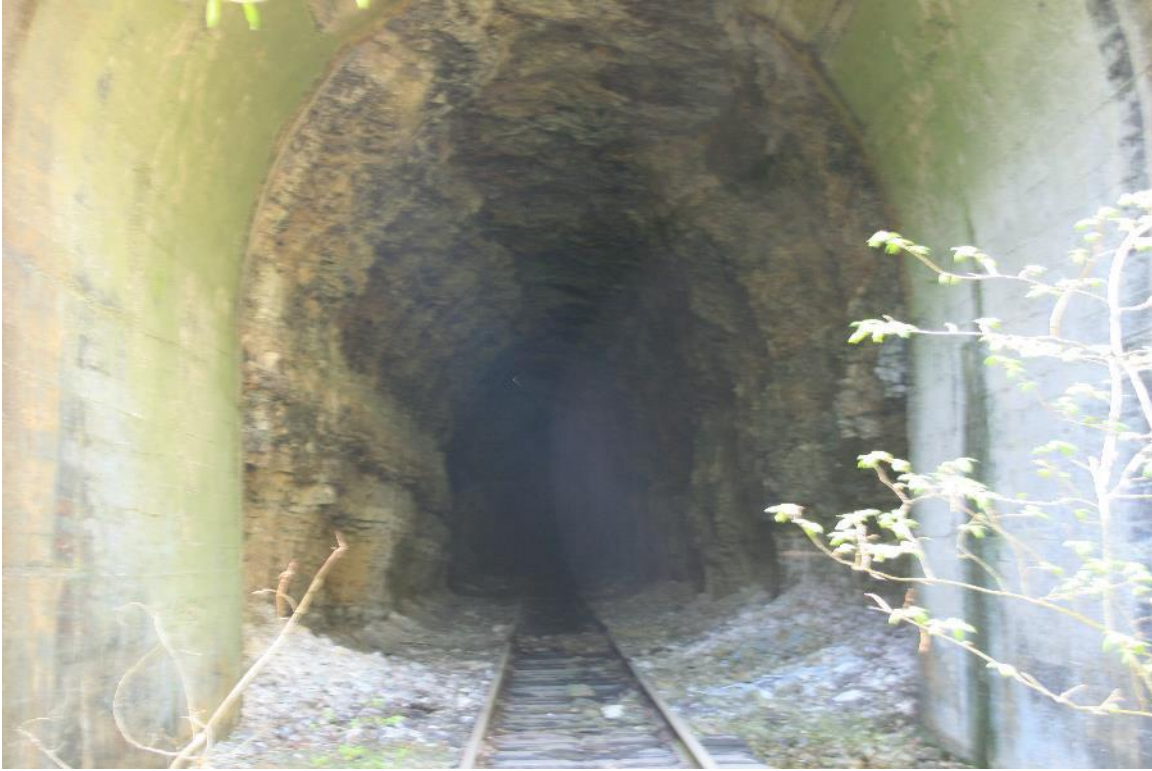
Photo 142: Tunnel 2, Meta Tunnel, Interior Bedrock Walls and Concrete Entrance, Facing West
