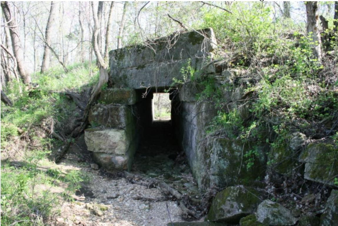
Photo 58: Culvert 126.50, Stone Box on North Side, Facing Southeast
