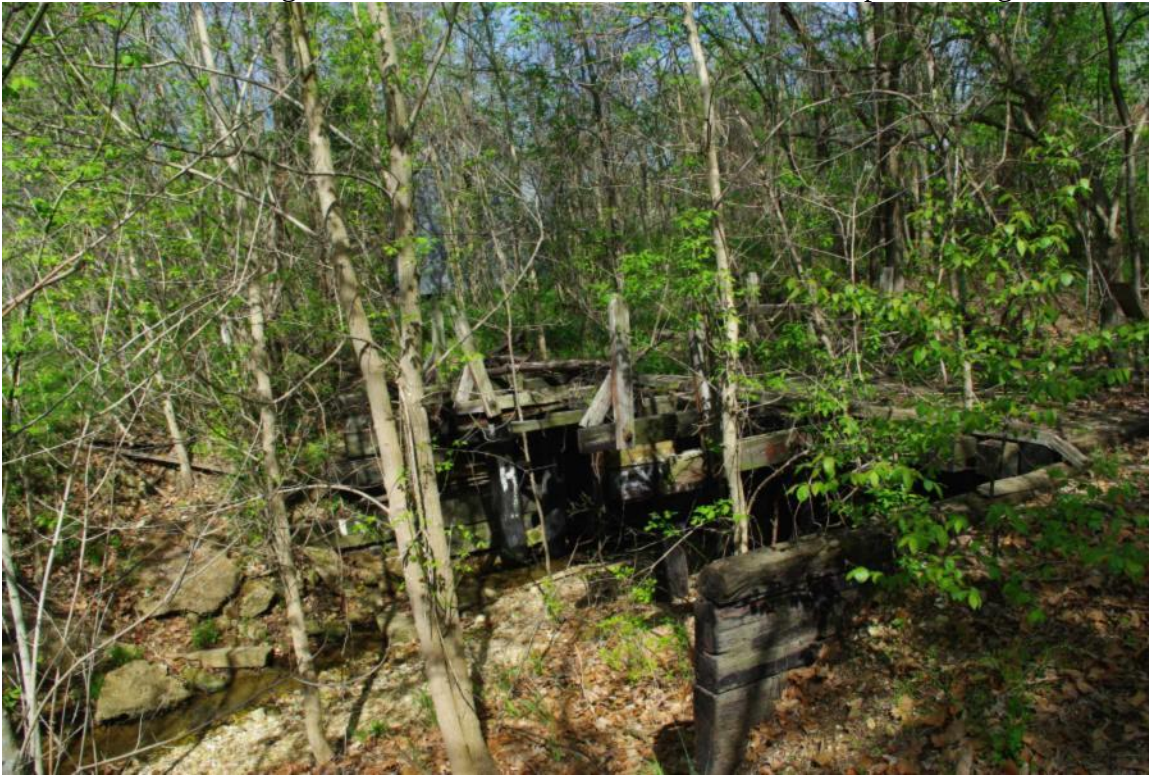
Photo 114: Bridge 149.40A, Wood Deck Beam Continuous Span, Facing West
