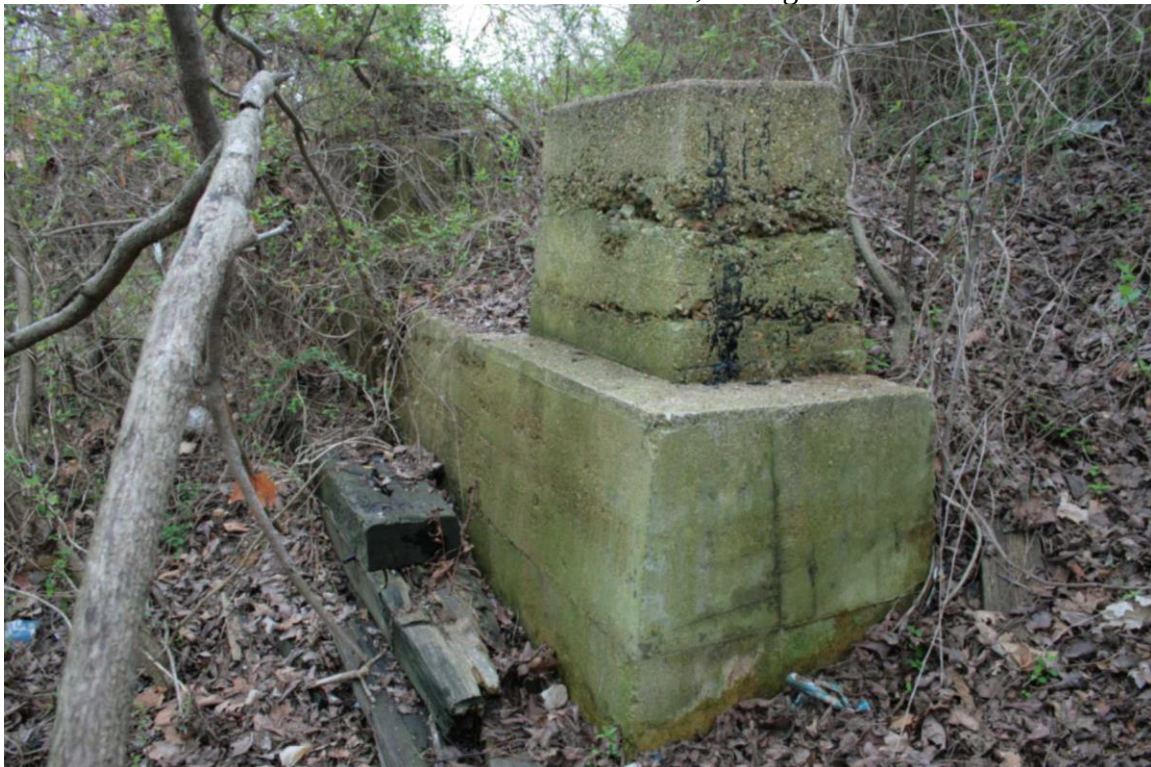
Photo 130: Bridge 160.47, South Concrete Abutment for Removed Bridge over South Walnut Avenue in Eldon, Facing Southeast
