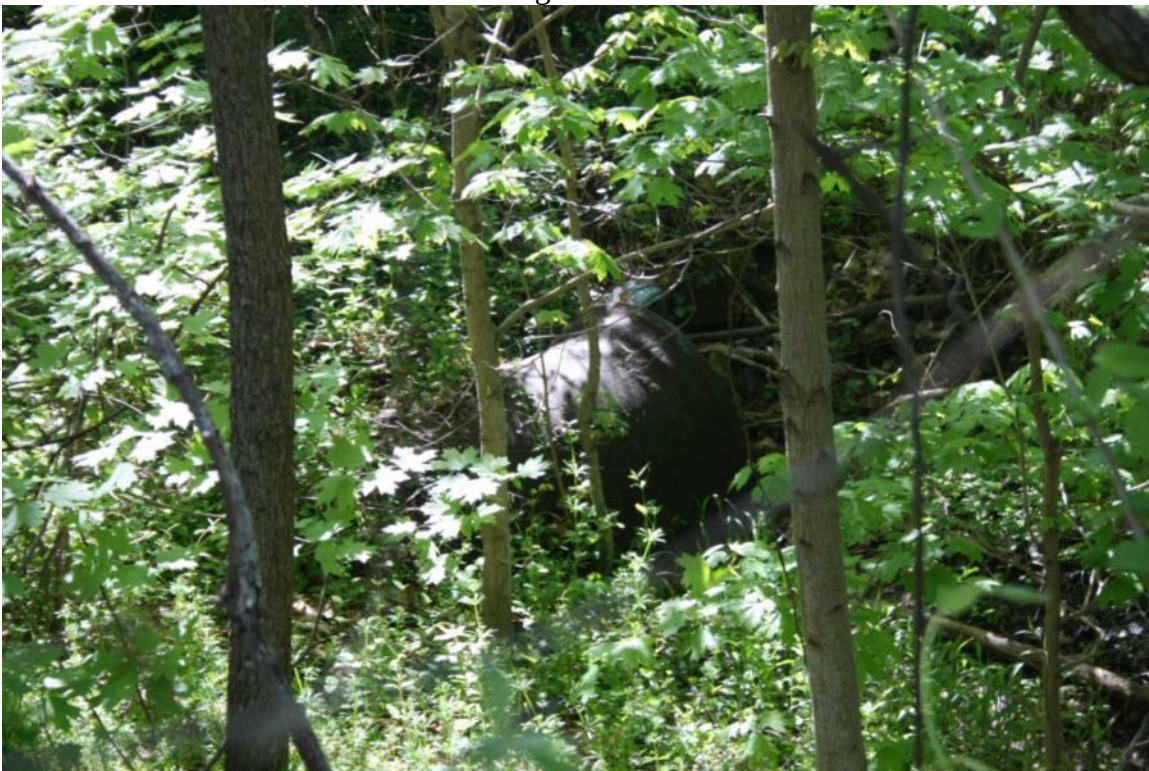
Photo 60: Culvert 74.27, Metal Drainage Pipe Inserted into Stone Box Culvert, Facing Southwest
