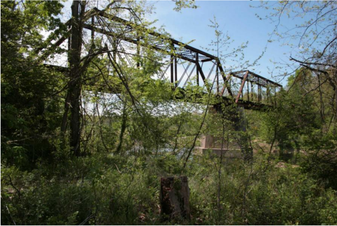
Photo 115: Bridge 121.50, Pratt Through Truss, Facing Southwest
