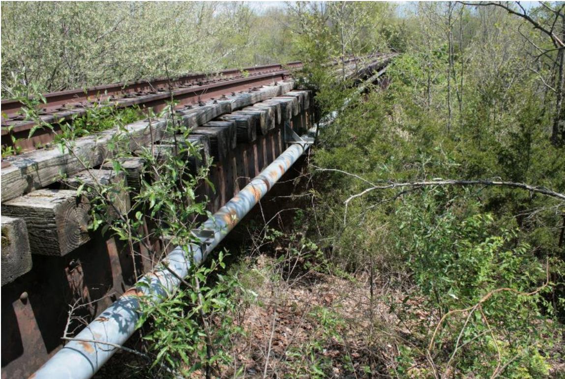
Photo 99: Bridge 86.95, Closeup of Modern Pipe along Side of Bridge, Facing Northeast
