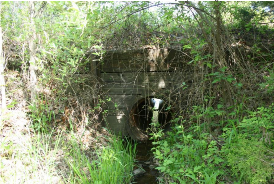
Photo 54: Culvert 83.62, Wood Tie with Clay Pipe, Facing North
