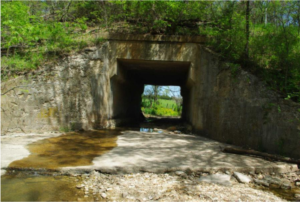
Photo 48: Culvert 88.92, Concrete Box Drive Through, Facing North
