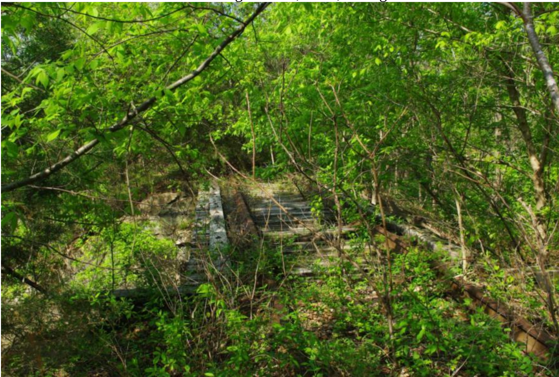
Photo 98: Bridge 135.70, Deck, Facing West
