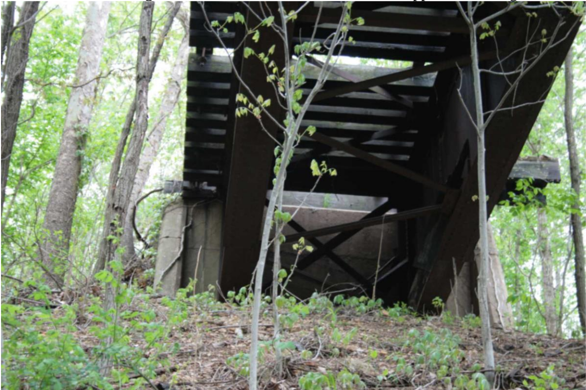
Photo 124: Bridge 143.33, Concrete Abutment on East Approach, Facing East
