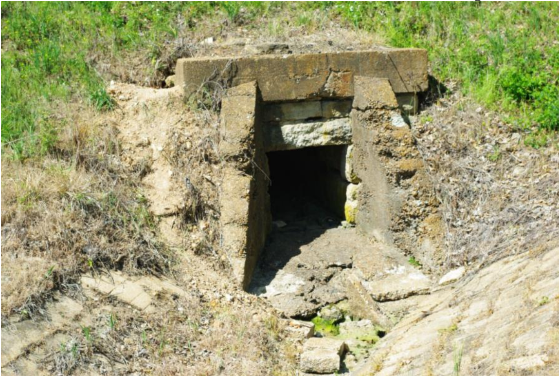
Photo 56: Culvert 100.38, Stone Box with Concrete Box Over, Facing North
