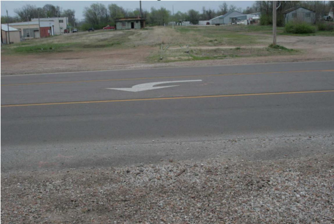
Photo 10: Removed Tracks at Walnut Street, between Mile Markers 177.00 and 178.00, Facing Northeast
