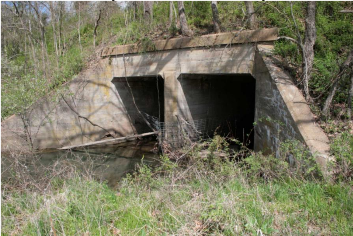
Photo 128: Bridge 155.20, Double Box Culvert, Facing Northwest
