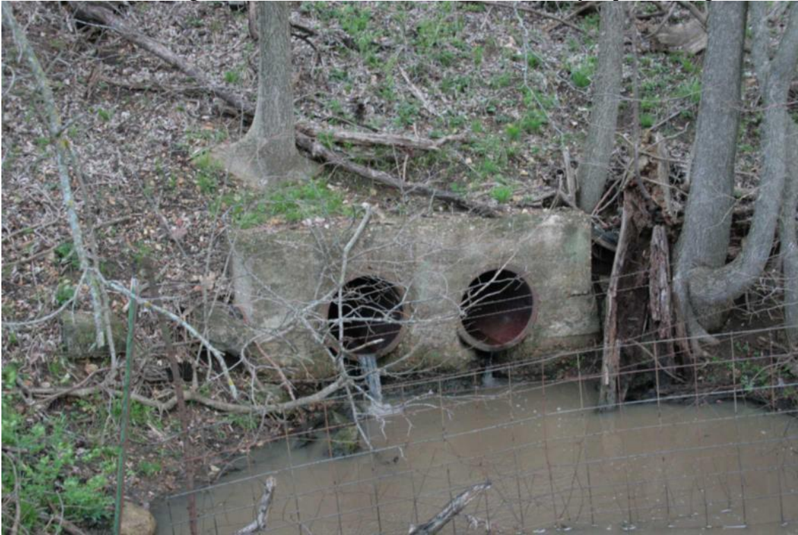
Photo 79: Drainage 163.62, Concrete Block with Double Clay Pipes, Facing North
