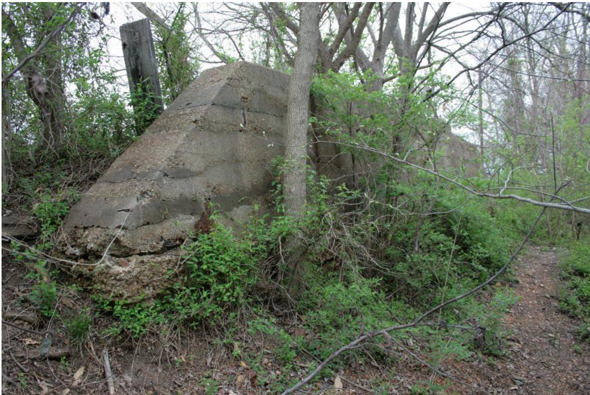
Photo 129: Bridge 160.47, North Concrete Abutment for Removed Bridge over South Walnut Avenue in Eldon, Facing Northwest
