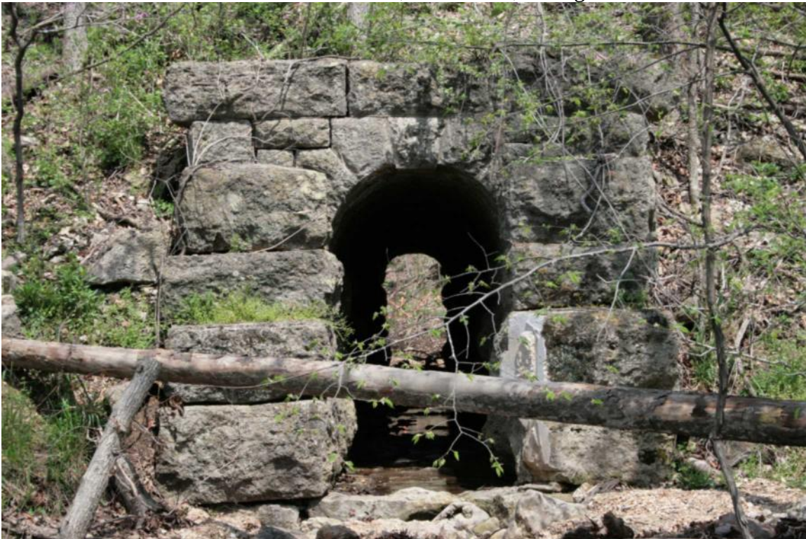
Photo 63: Culvert 147.30, Stone Arch, Facing North
