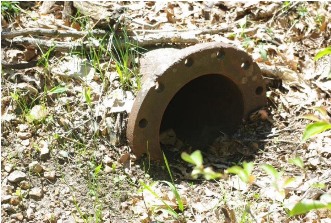
Photo 81: Drainage 132.10, Iron Pipe, Facing Southwest
