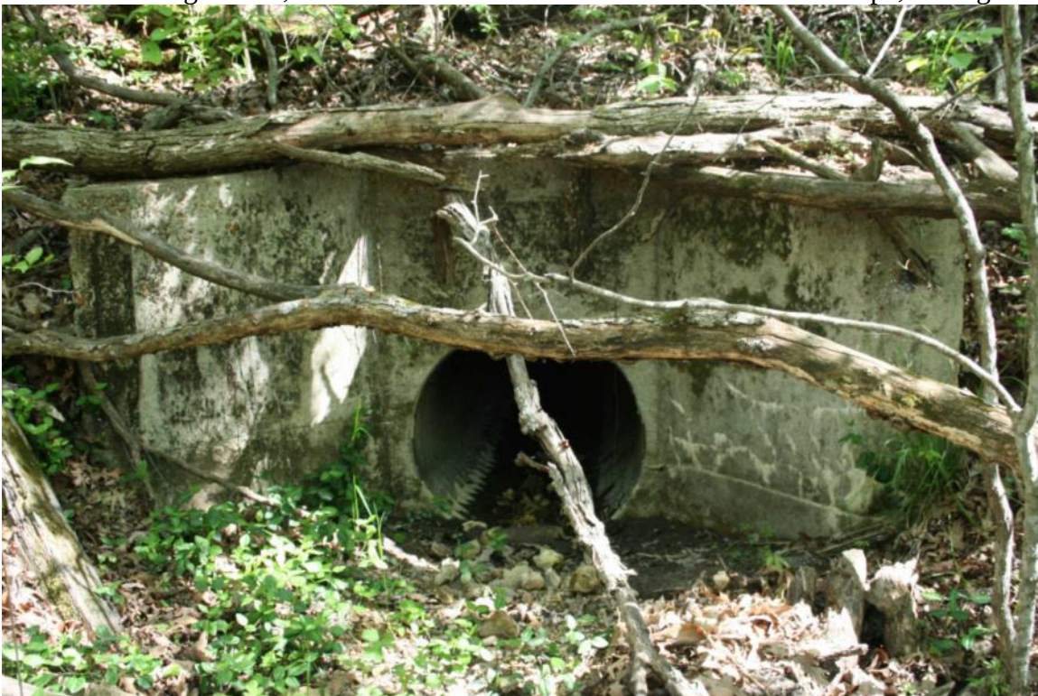
Photo 85: Drainage 73.25, Modern Concrete Block with Galvanized Steel Pipe, Facing North
