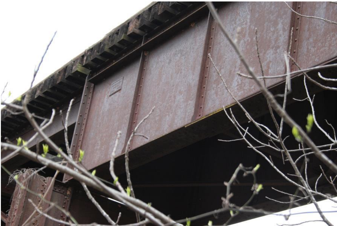
Photo 109: Bridge 189.75, American Bridge Plaque, Facing Northwest
