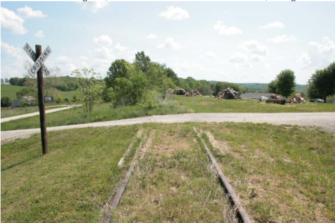
Photo 9: Missing Ties, between Mile Markers 110.00 and 111.00, Facing East
