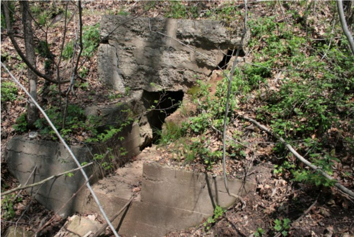
Photo 55: Culvert 147.18, Stone Box Reinforced with Concrete, Facing North
