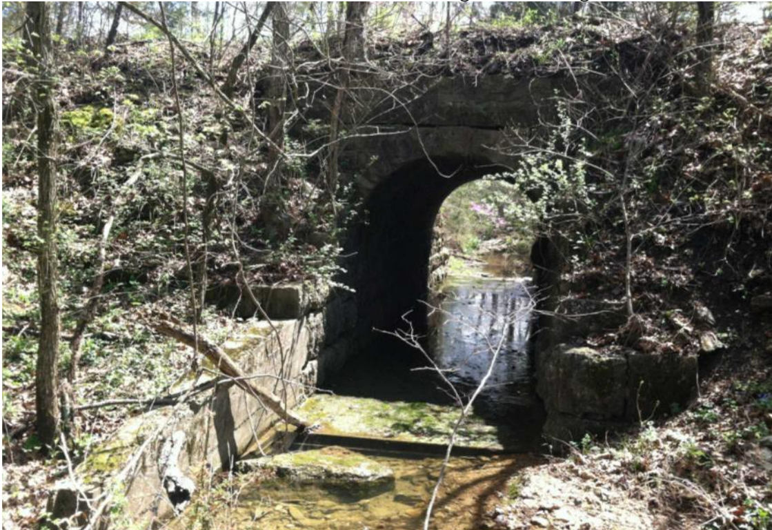
Photo 72: Culvert 148.31, Concrete Wing Wall, Facing Northeast
