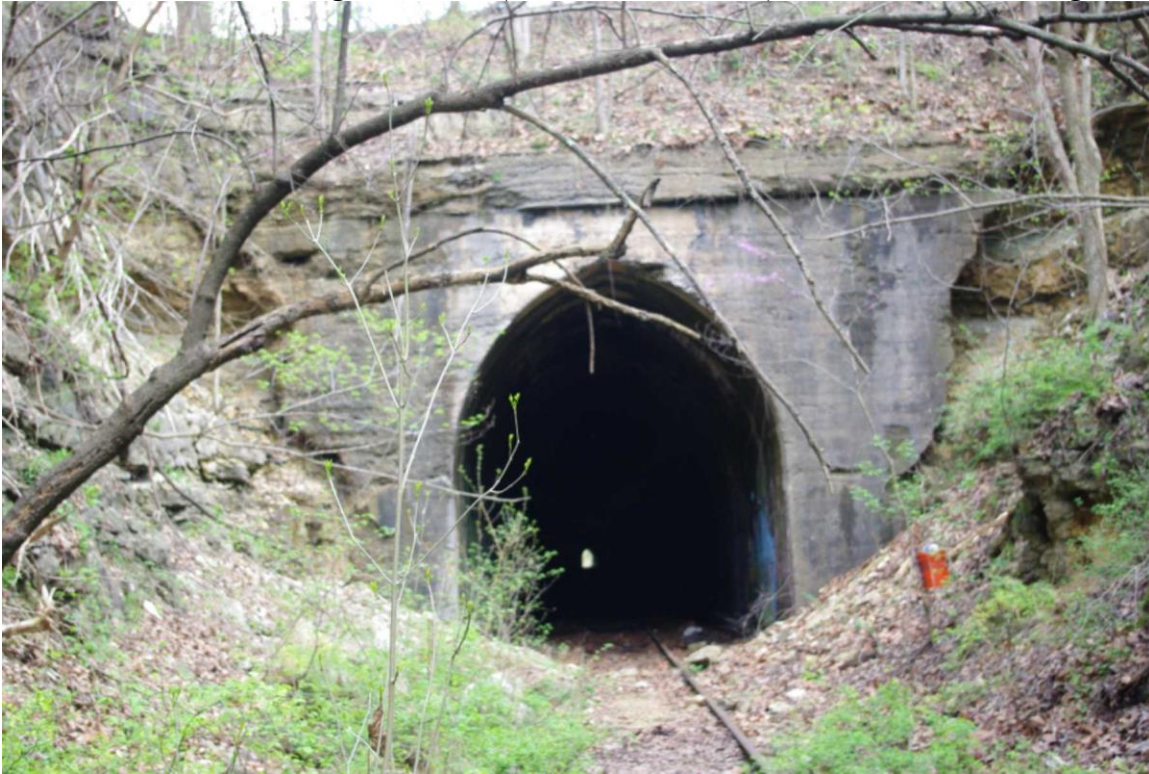
Photo 135: Tunnel 3, Eugene Tunnel (Mile Marker 148.81), West Entrance, Facing East
