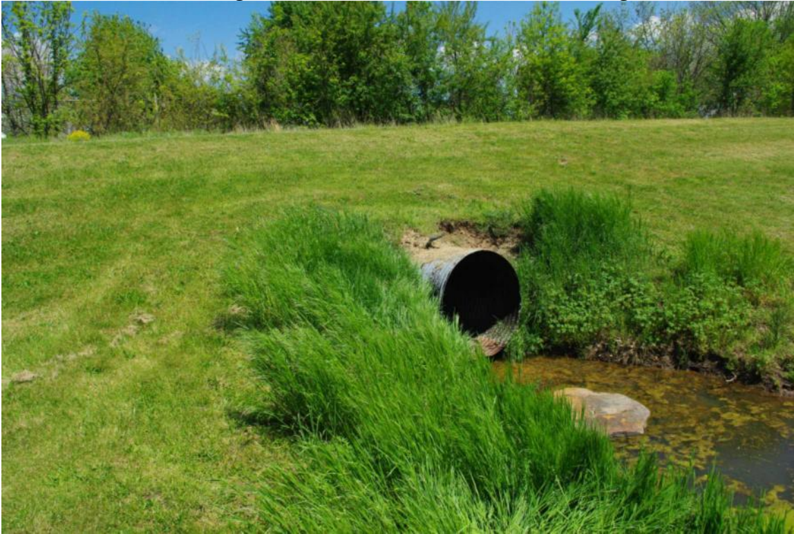
Photo 84: Drainage 105.05, Modern Galvanized Steel, Facing Northeast
