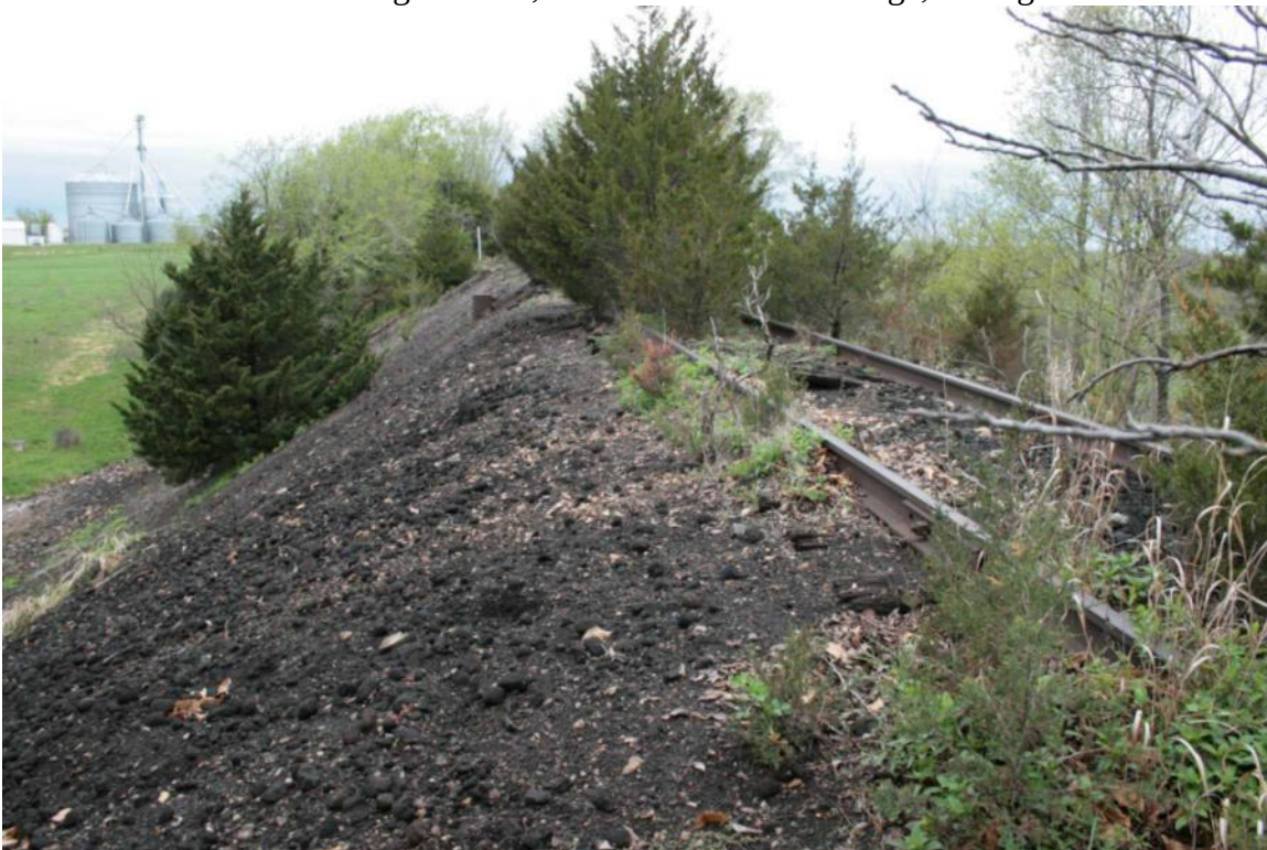
Photo 132: Bridge 198.40, Infilled Deck Plate Bridge, Facing West
