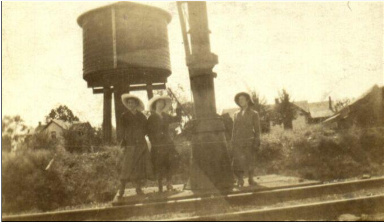
Figure 21: Former Water Tower at Belle (Osage Historical Society 2003)
