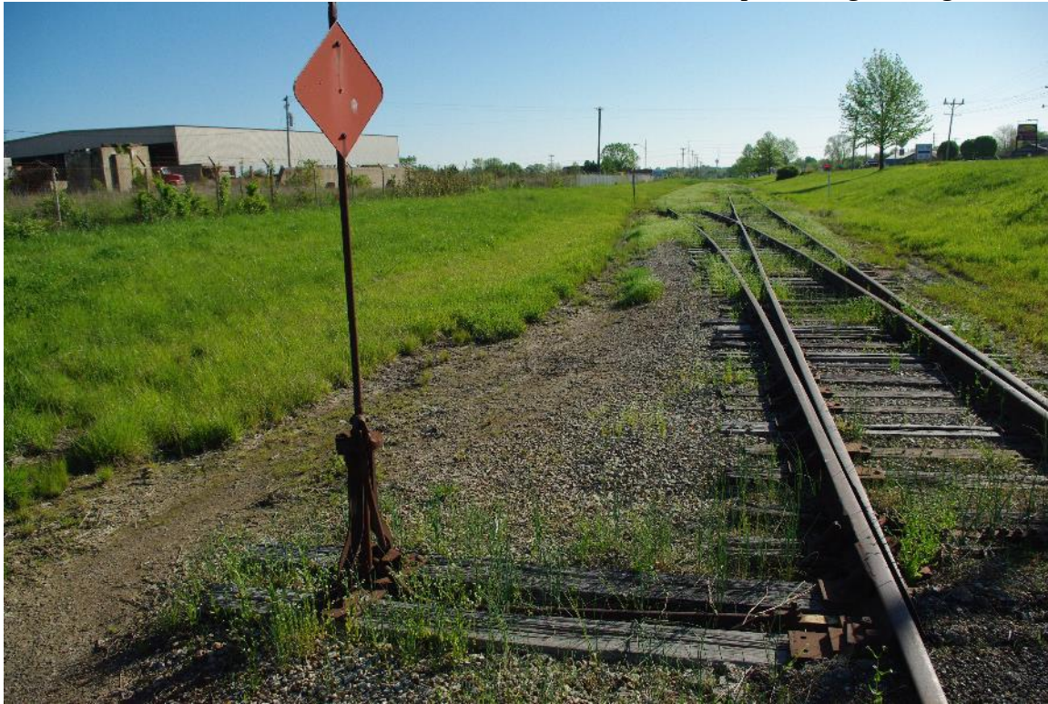
Photo 150: Switch 32: 91.50, South Switch for Owensville Depot Siding, Facing North
