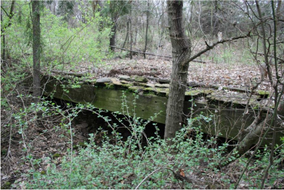
Photo 87: Bridge 137.70, Deck Beam Continuous Span Bridge, Facing Southwest
