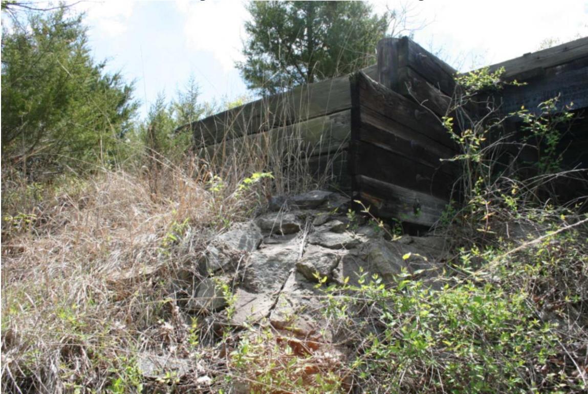
Photo 95: Bridge 78.60, Wood Abutment, Facing Northeast
