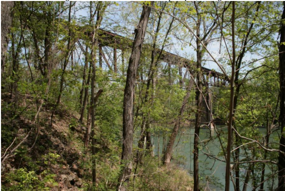
Photo 100: Bridge 114.70, Pratt Deck Truss Simple Span, Facing Northeast
