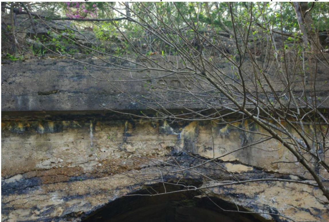
Photo 140: Tunnel 3, Eugene Tunnel, Closeup of “No 3” and “1903” Inscription, Facing West
