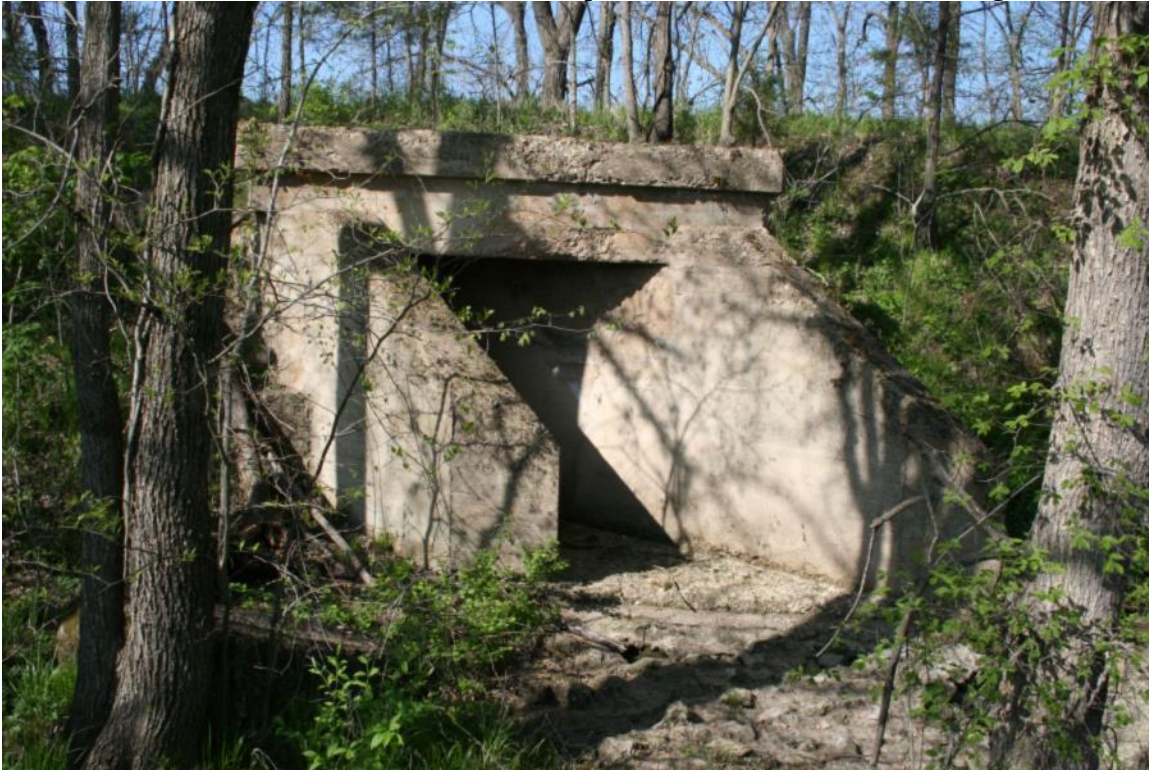
Photo 57: Culvert 126.50, Concrete Box Replacement on South Side, Facing Northeast
