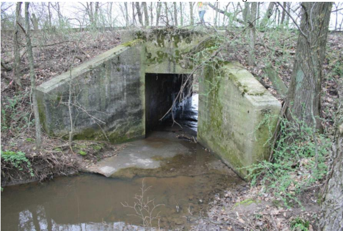
Photo 47: Culvert 213.35, Concrete Box, Facing Southeast
