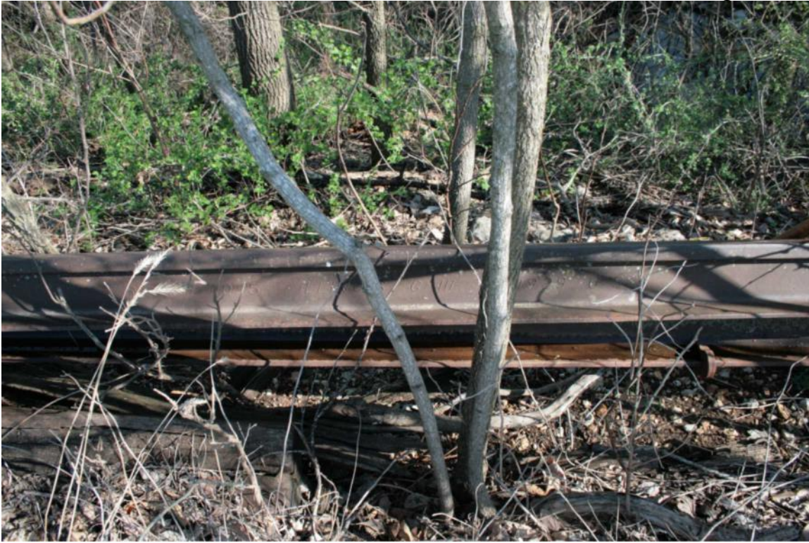
Photo 12: Embossed Track, between Mile Markers 180.00 and 181.00, Facing North
