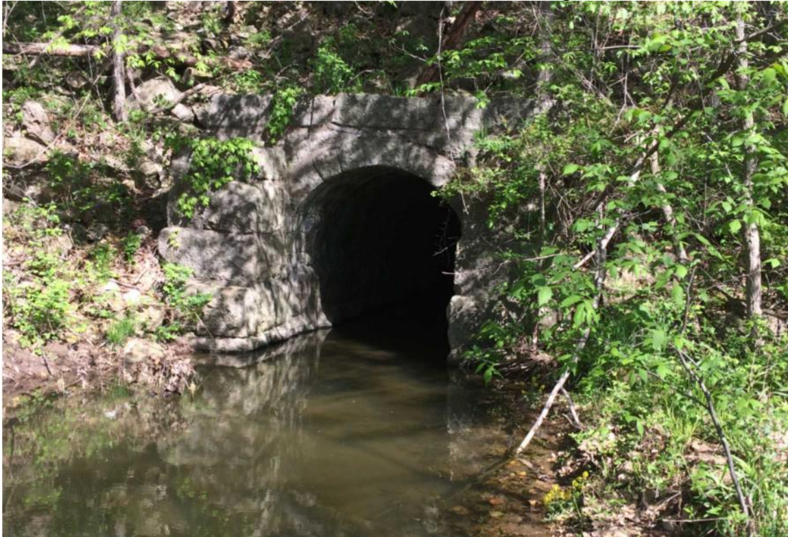
Photo 62: Culvert 117.65, Stone Arch, Facing North
