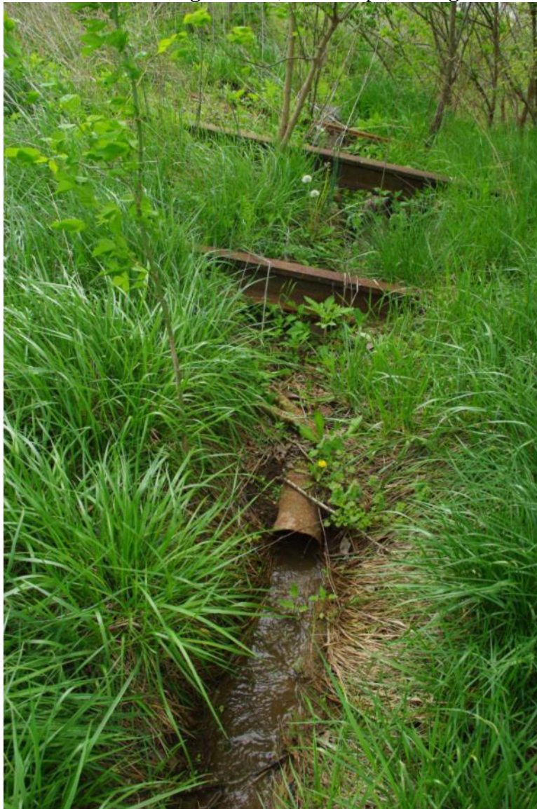
Photo 82: Drainage 144.72, Metal Pipe, Facing South
