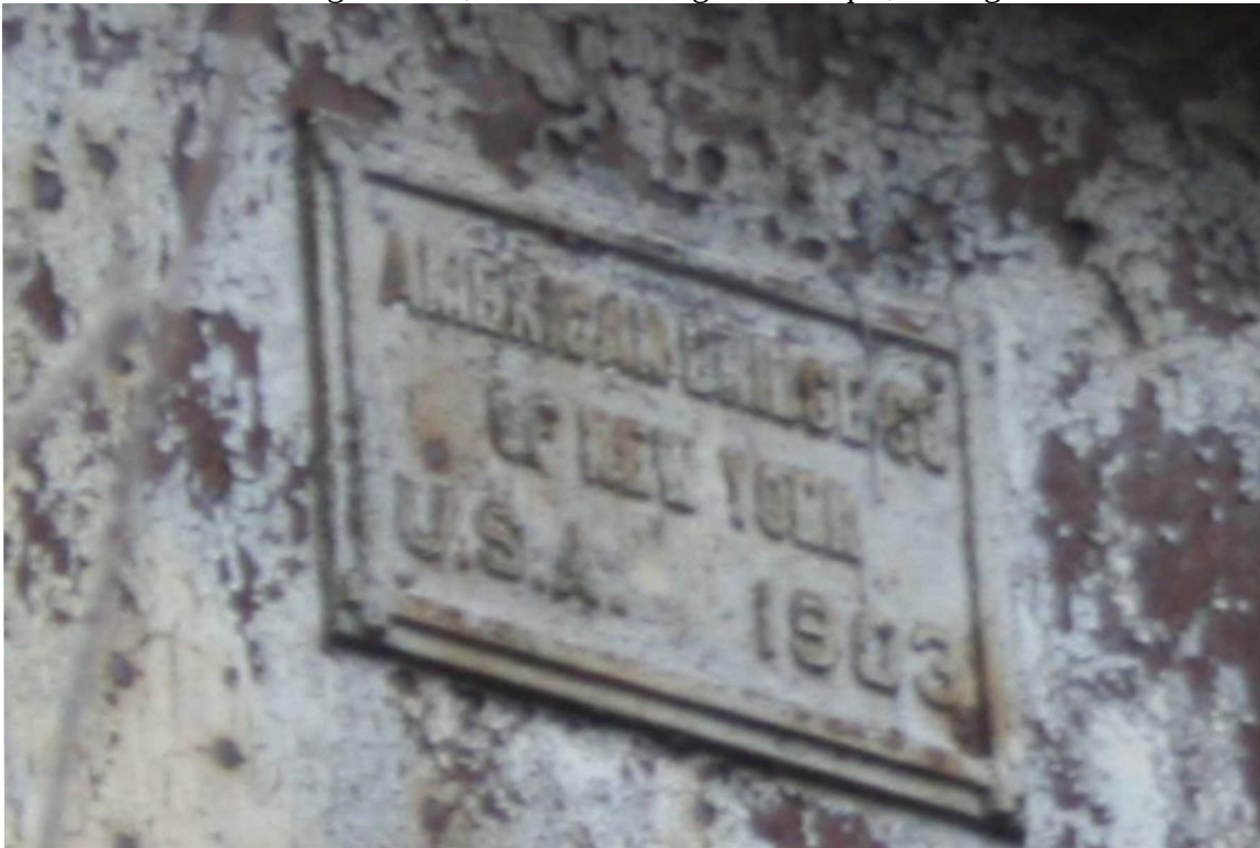
Photo 97: Bridge 215.30, American Bridge Co. Plaque, Facing Southwest
