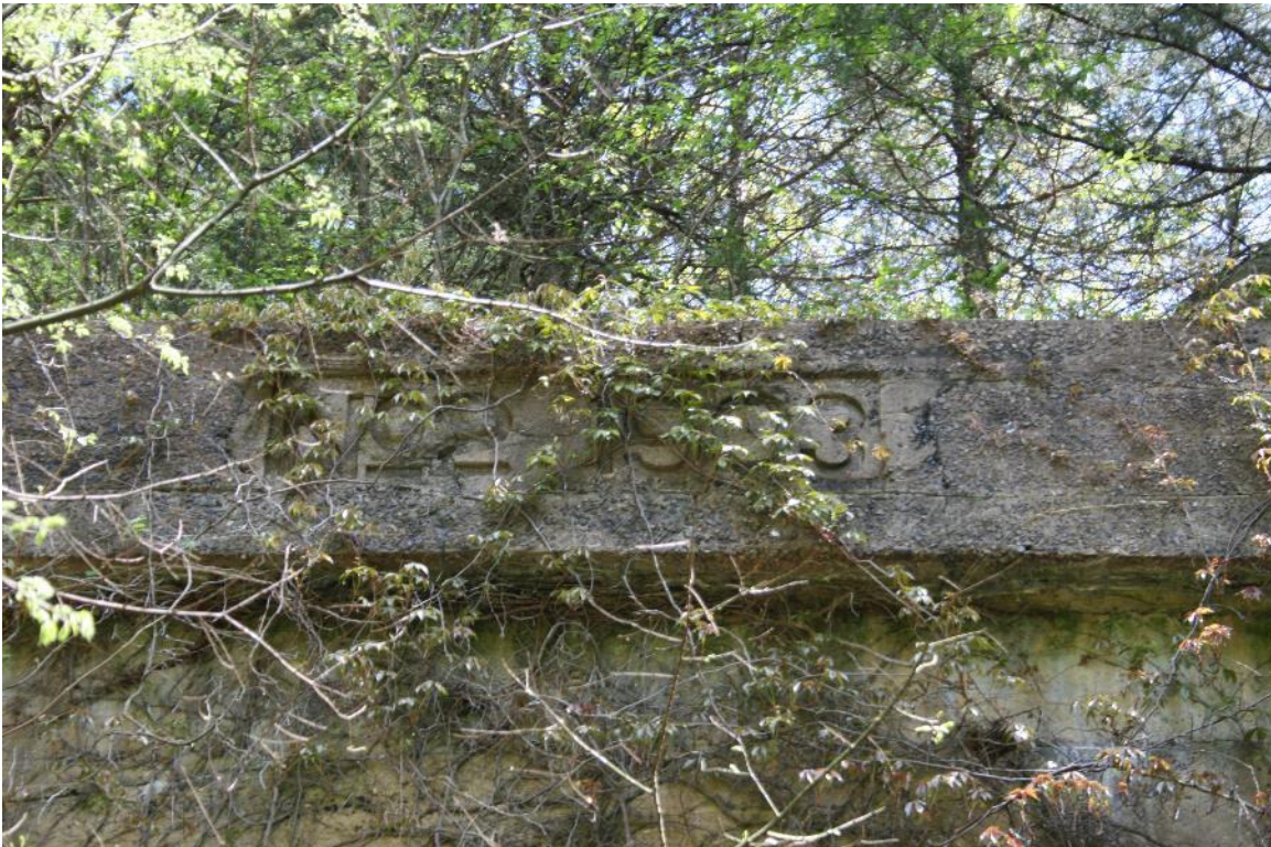
Photo 139: Tunnel 2, Meta Tunnel, Closeup of Inscription “No 2” and “1903”, Facing East
