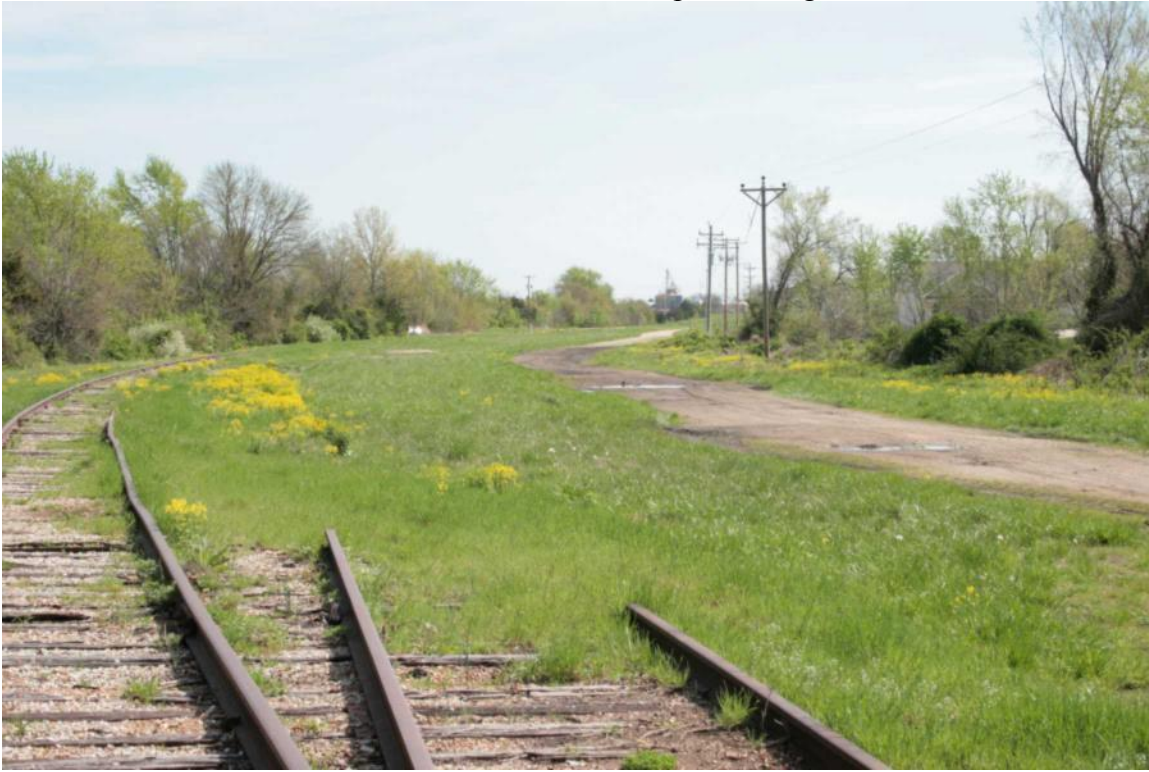
Photo 35: Location of Versailles Depot, Facing Northeast
