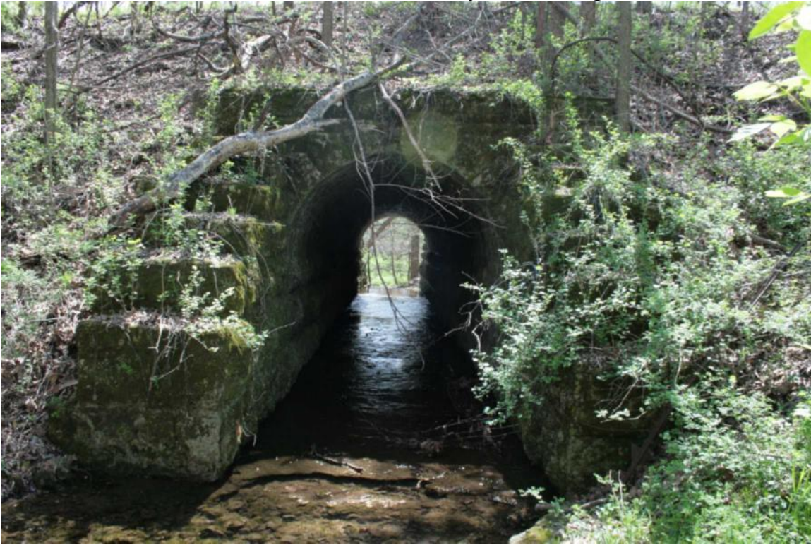
Photo 70: Culvert 146.68, Masonry Arch, Facing South
