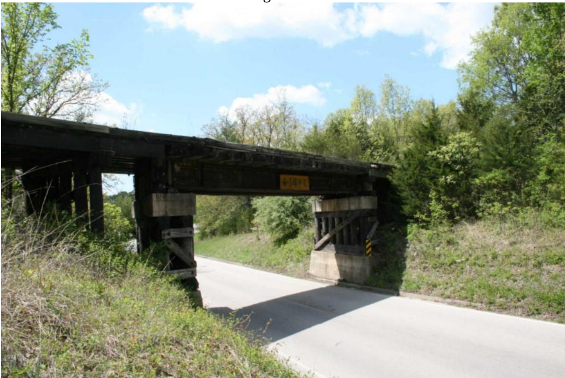
Photo 96: Bridge 78.60, Deck Plate with Transverse Bracing Wood and Concrete Piers, Facing Southwest
