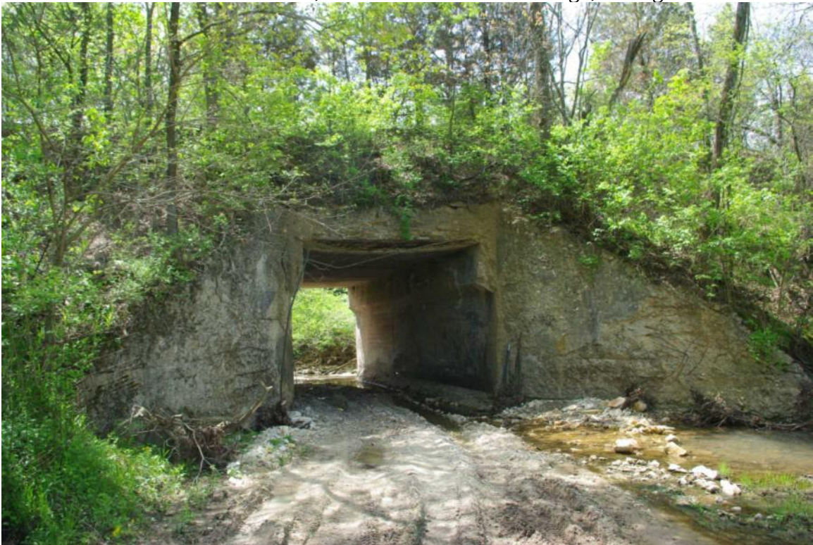
Photo 49: Culvert 88.92, Concrete Box Drive Through, Facing South
