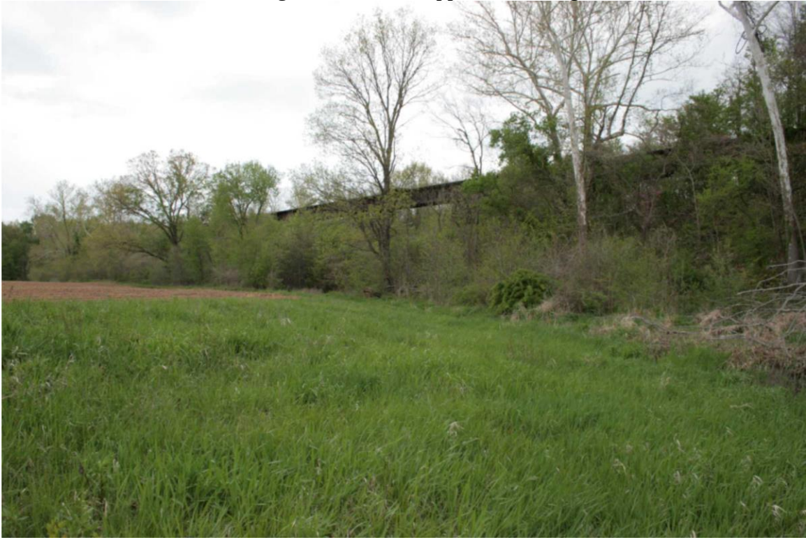
Photo 123: Bridge 143.33, East Approach, Facing Northwest
