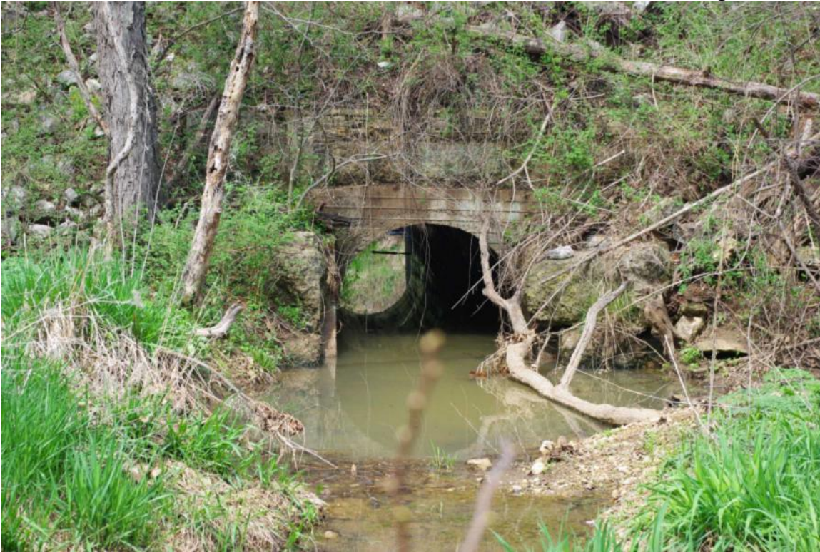
Photo 71: Culvert 174.85, Stone Arch with Inserted Concrete Arch, Facing North
