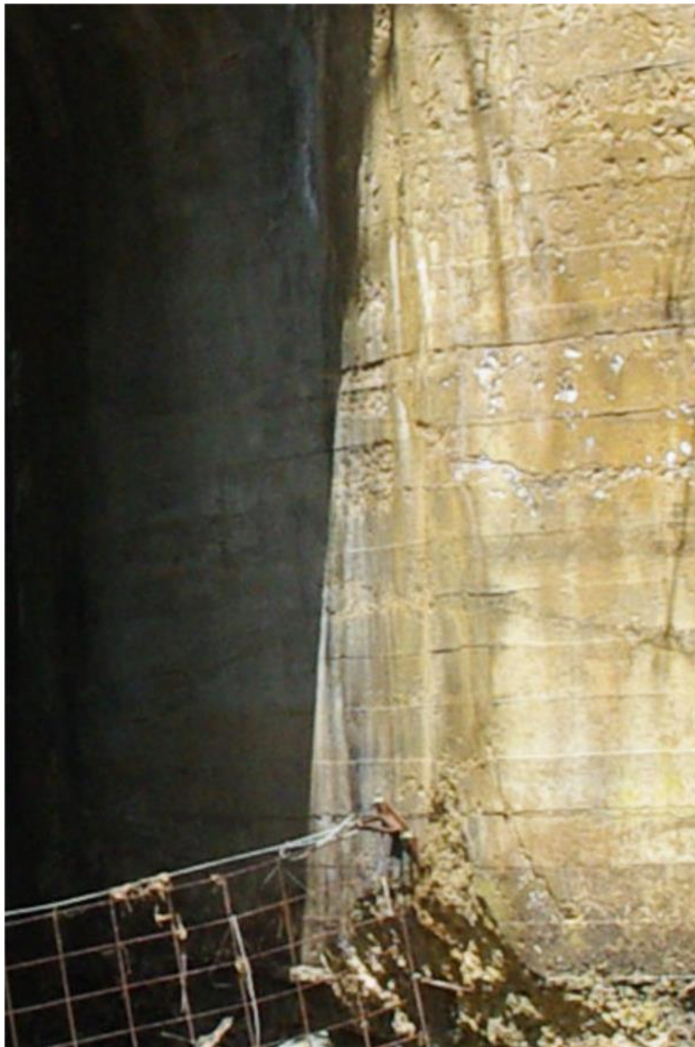
Photo 66: Culvert 88.20, Closeup of East Wall Showing Board Formed Concrete, Facing Northeast
