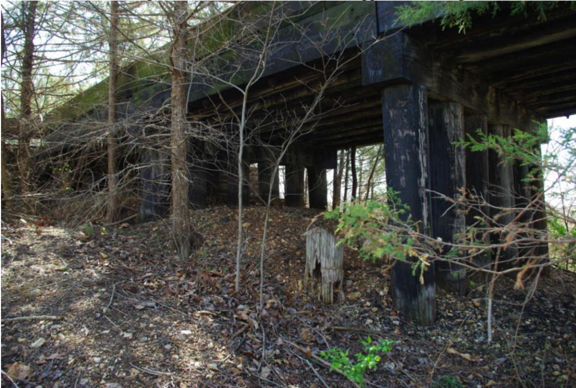
Photo 93: Bridge 183.50, Wood Piers for East Approach, Facing Southeast
