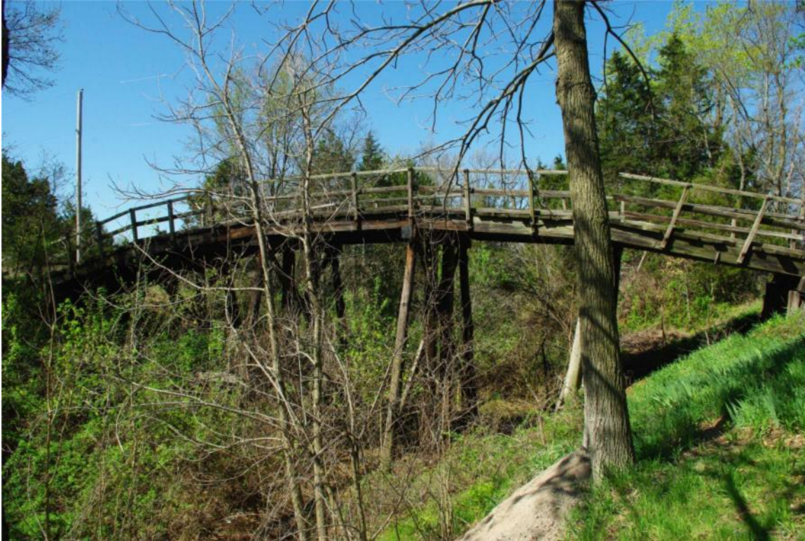
Photo 110: Bridge 184.47, Deck Arch Beam Bridge, Facing West
