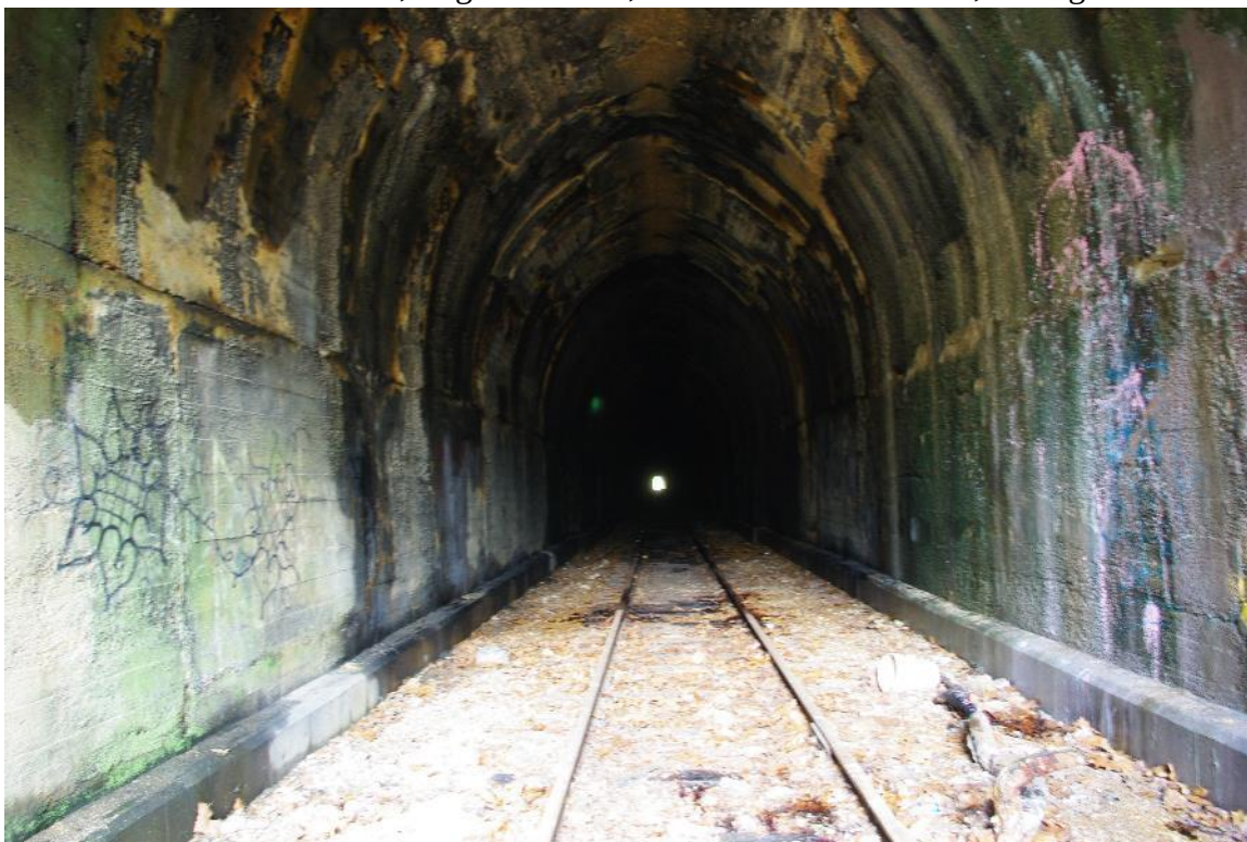
Photo 141: Tunnel 3, Eugene Tunnel, Interior Concrete Walls, Facing East
