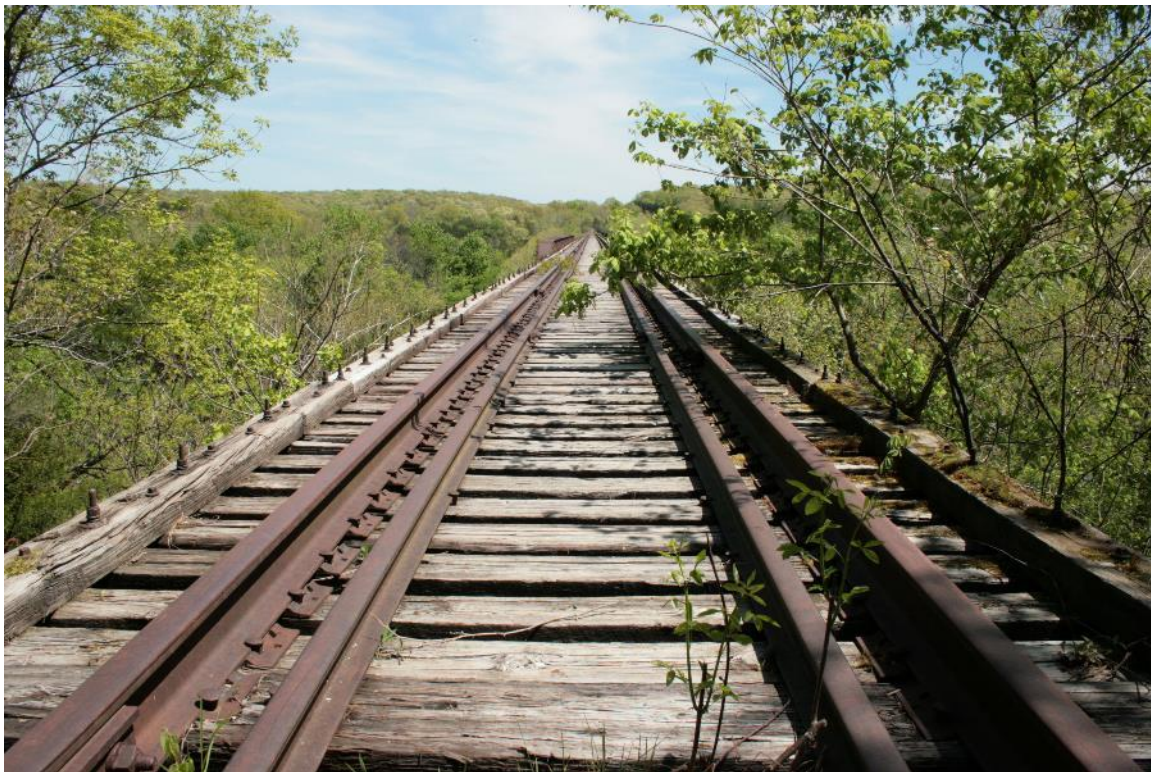
Photo 103: Bridge 114.70, Deck, Facing East
