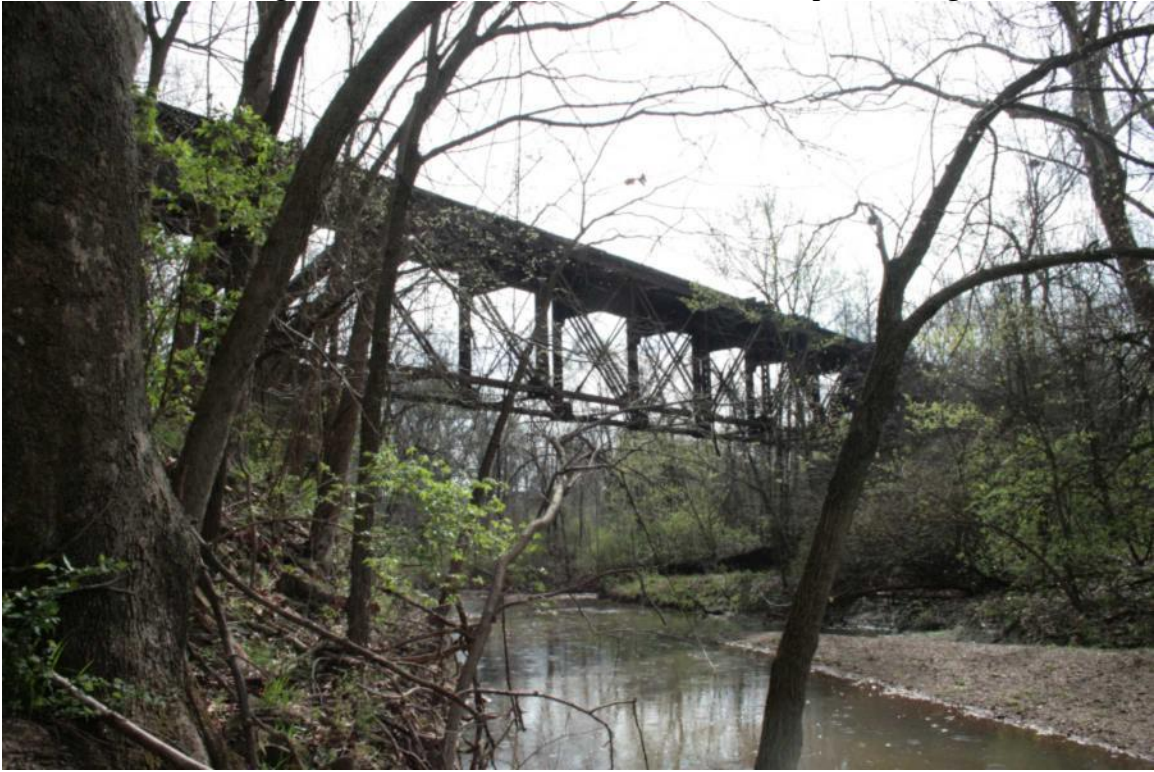
Photo 105: Bridge 189.75, Pratt Deck Truss Continuous Span, Facing Northeast
