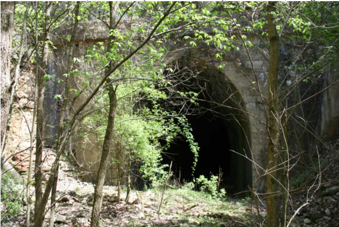
Photo 134: Tunnel 2, Meta Tunnel (Mile Marker 128.67), West Entrance, Facing East
