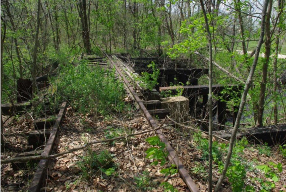
Photo 111: Bridge 144.90, Deck Beam Bridge and Wood Piers of Absent Bridge, Facing West
