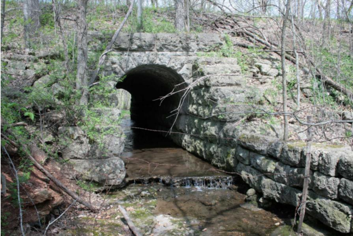
Photo 69: Culvert 146.68, Masonry Arch, Facing North
