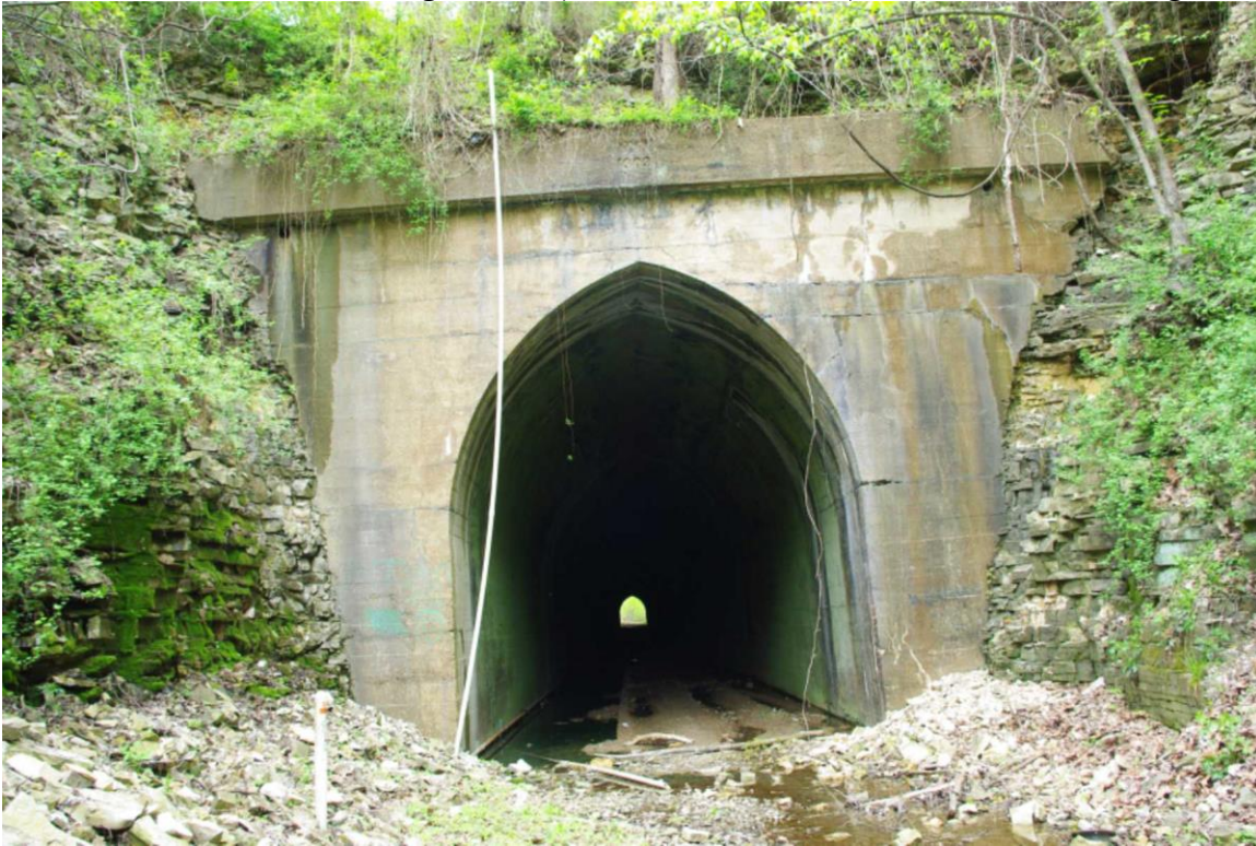
Photo 133: Tunnel 1, Freeburg Tunnel (Mile Marker 118.41), East Entrance, Facing West
