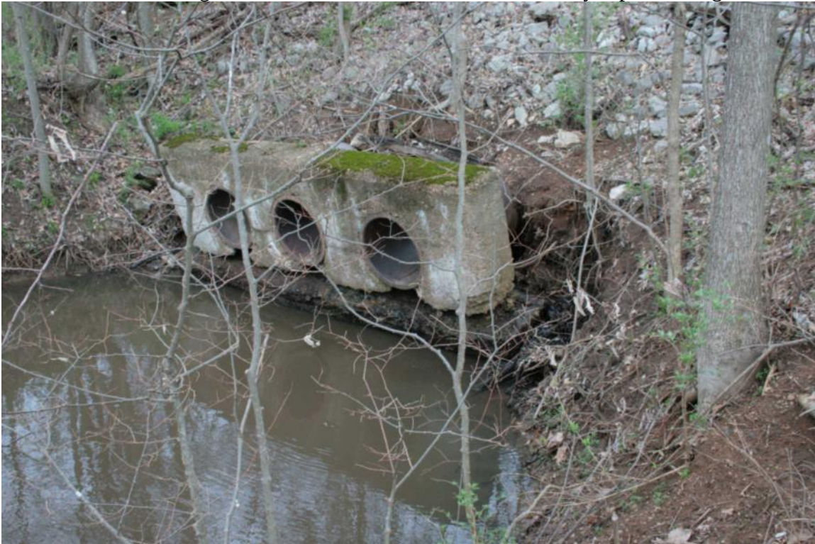
Photo 80: Drainage 163.30, Concrete Block with Three Clay Pipes, Facing South
