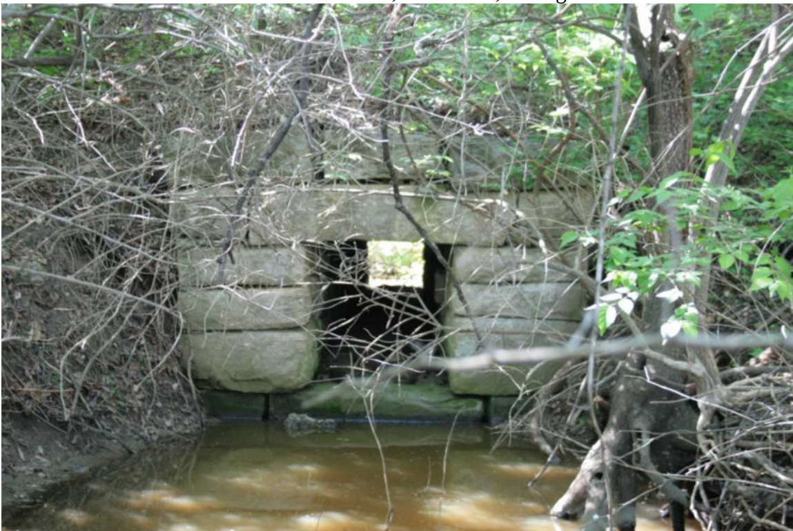
Photo 43: Culvert 94.12, Stone Box, Facing South
