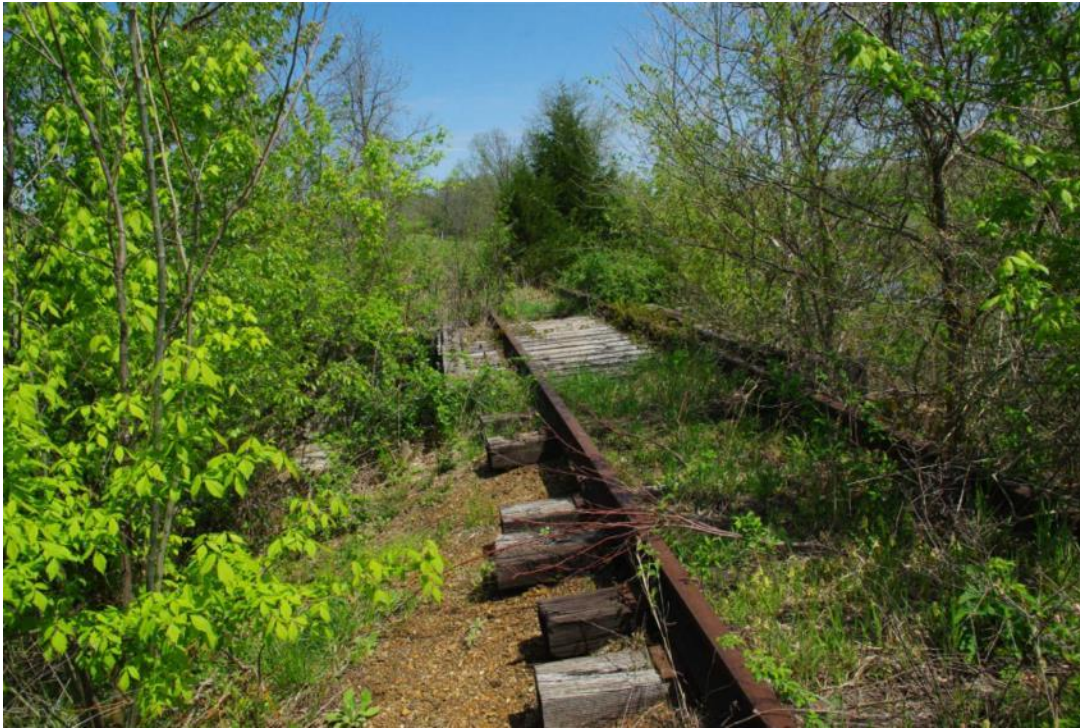
Photo 90: Bridge 123.20, Deck, Facing North
