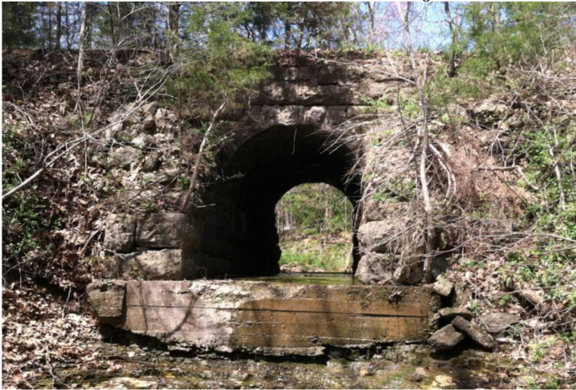
Photo 73: Culvert 148.31, Concrete Floor, Facing South
