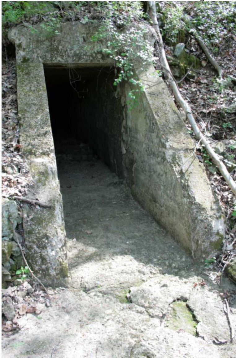
Photo 45: Culvert 112.65, Concrete Box, Facing North
