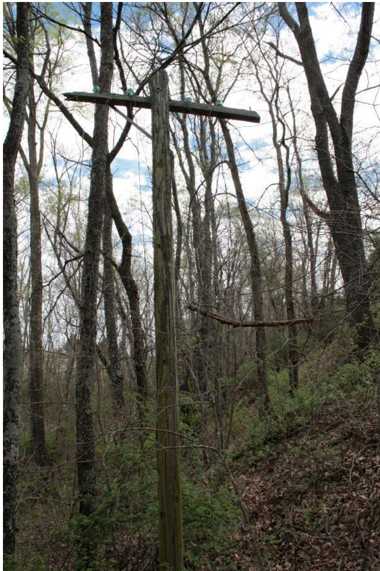
Photo 152: 190.00-Cedar Telegraph/Telephone Pole, With Insulators and Metal Wiring Intact, Facing East
