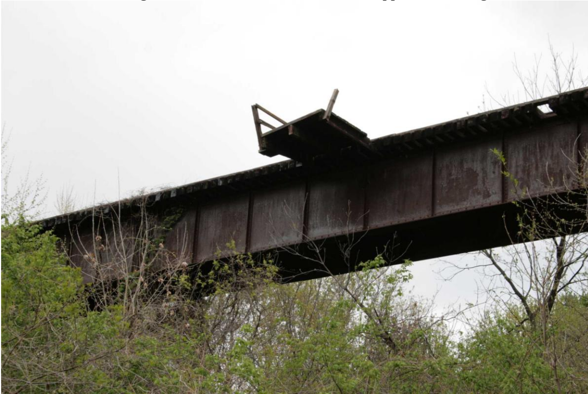
Photo 126: Bridge 143.33, Wood Platform on East Approach, Facing Northwest
