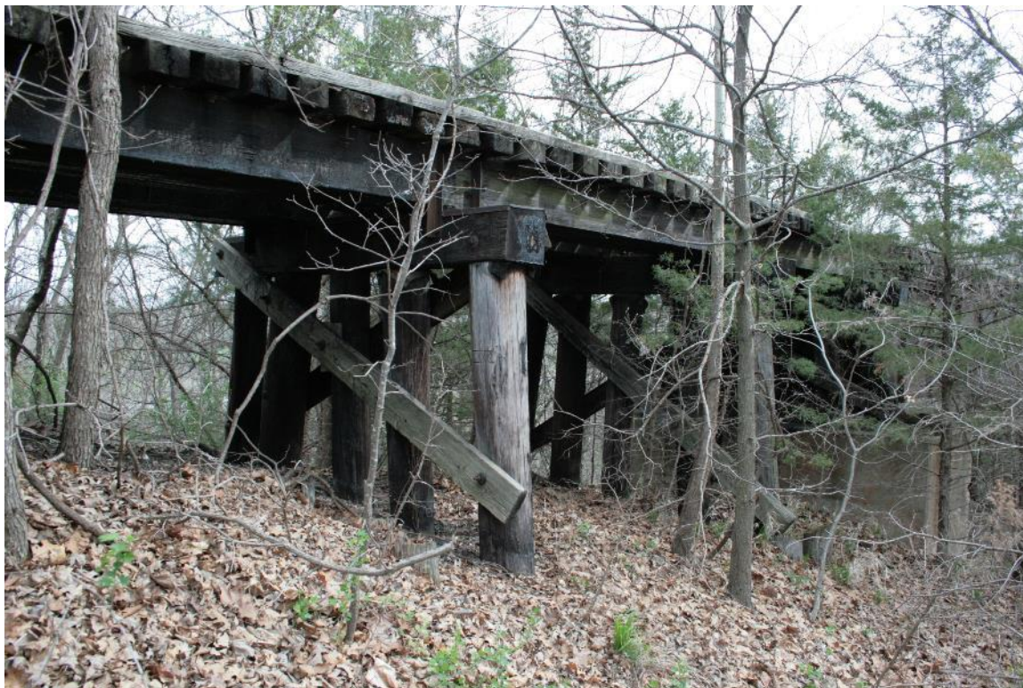
Photo 107: Bridge 189.75, Wood Piers under West Approach, Facing Northeast
