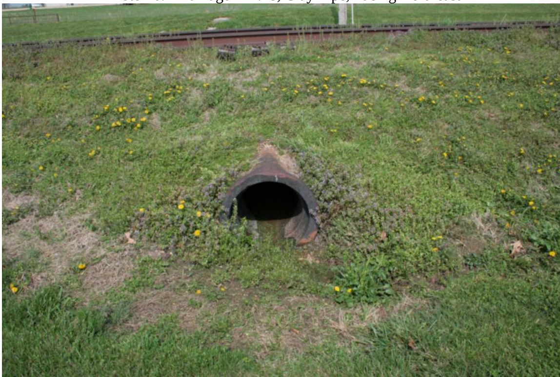
Photo 76: Drainage 171.28, Clay Pipe, Facing Northeast
