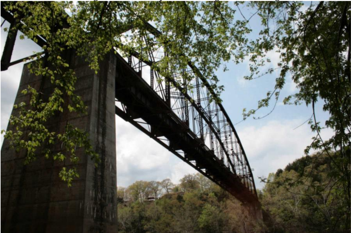
Photo 122: Bridge 143.33, Pennsylvania Through Truss, Facing Southwest
