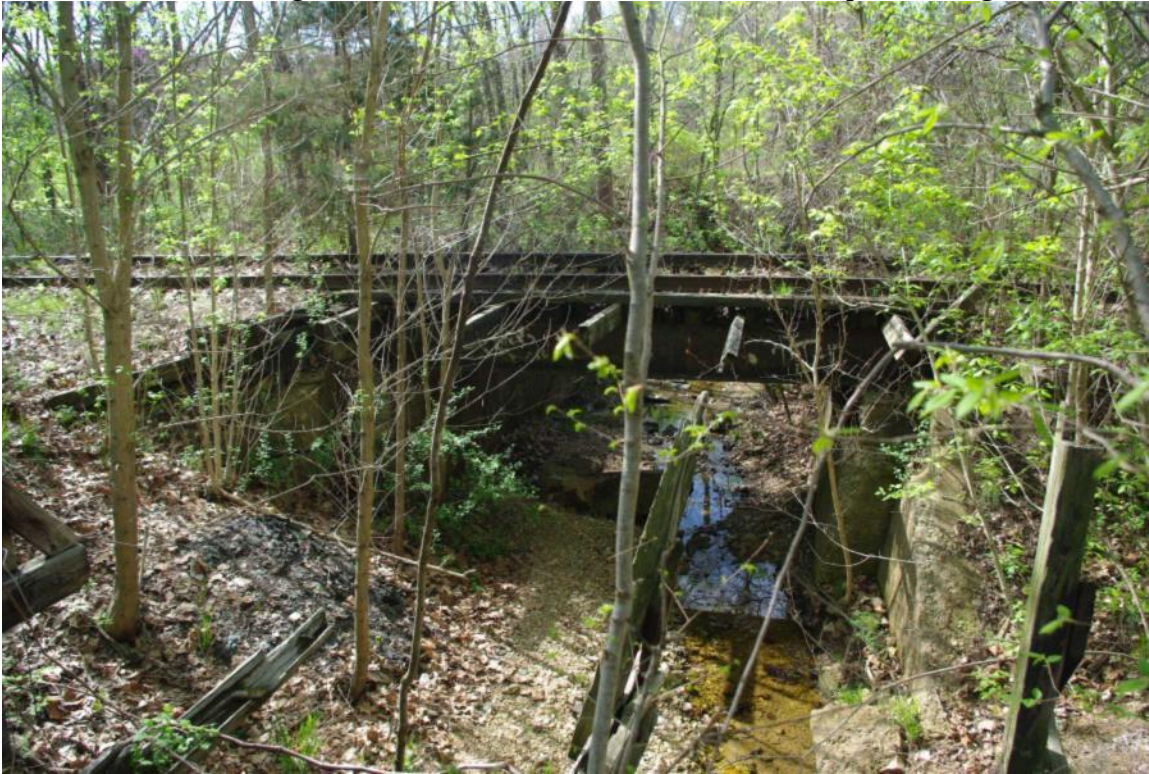
Photo 113: Bridge 149.40, Metal Deck Beam Continuous Span, Facing South
