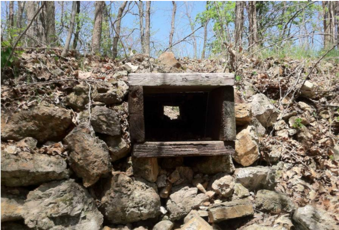
Photo 53: Culvert 132.10, Close-Up of South Side of Wood Box Culvert, Facing North
