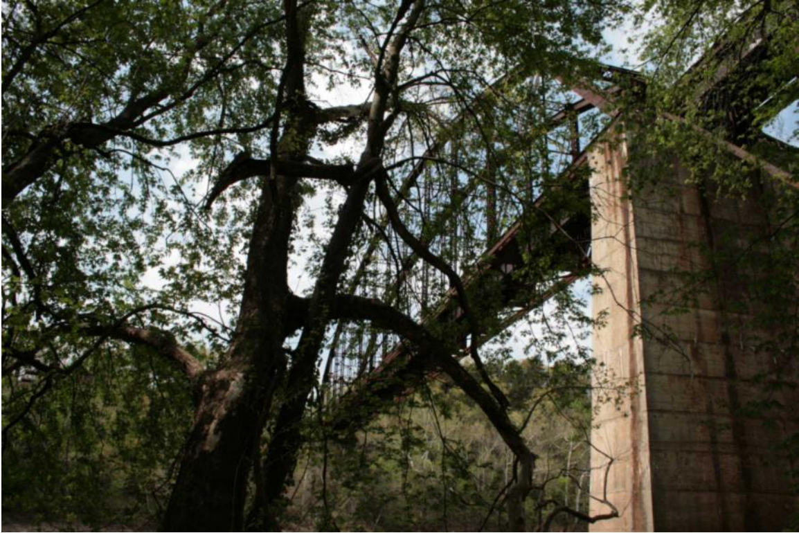
Photo 121: Bridge 143.33, Pennsylvania Through Truss, Facing Northwest
