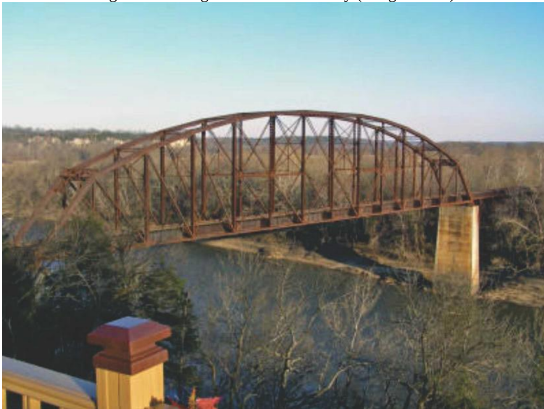
Figure 46: Bridge 143.33 from Henley (Baughn 2014)
