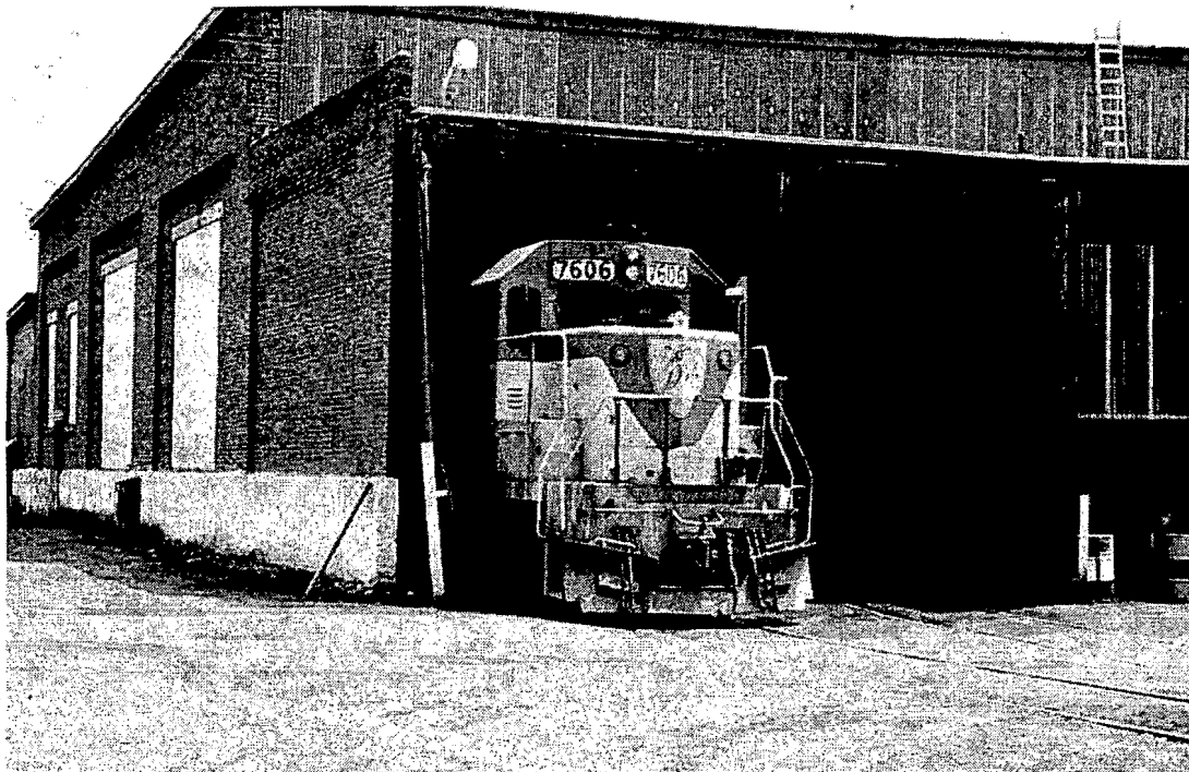
D&H engine terminal, 1970s, before demolition. Source: RailroadForums.com
