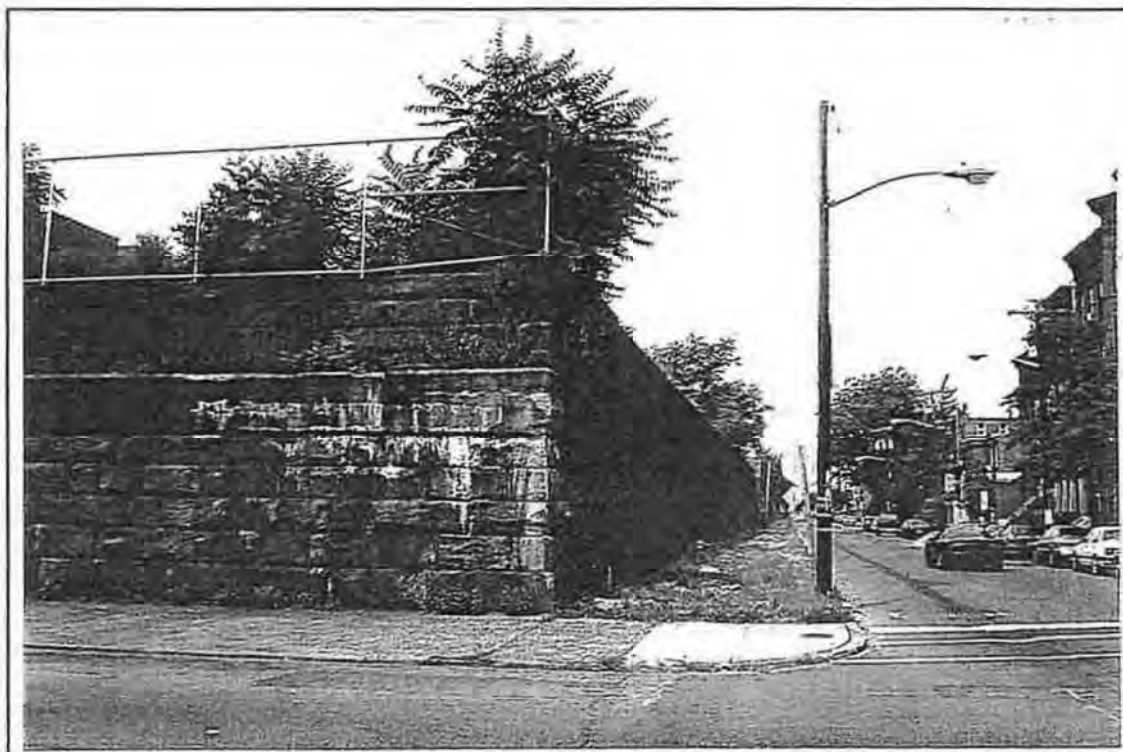
PLATE 2: View of Embankment at Manila and Sixth Streets, Looking West
