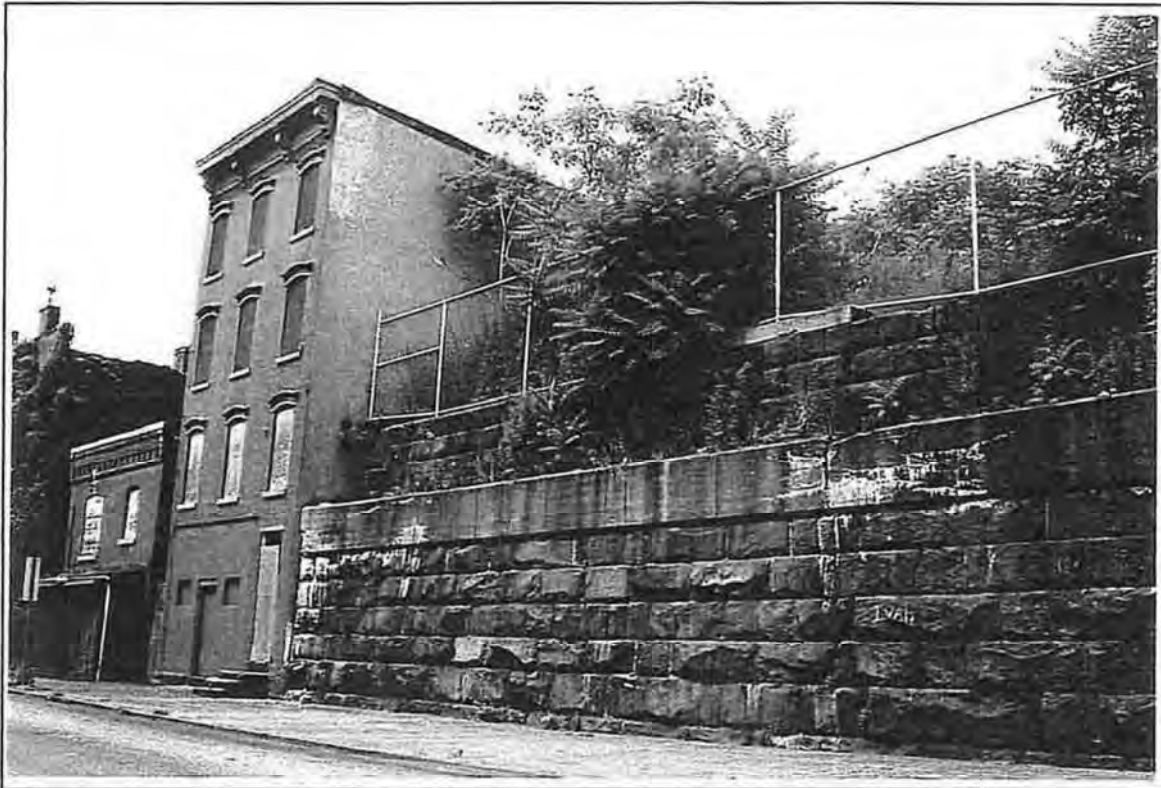
PLATE 10: Abandoned Buildings in Harsimus Cove Historic District, Looking West from Sixth and Erie Streets
