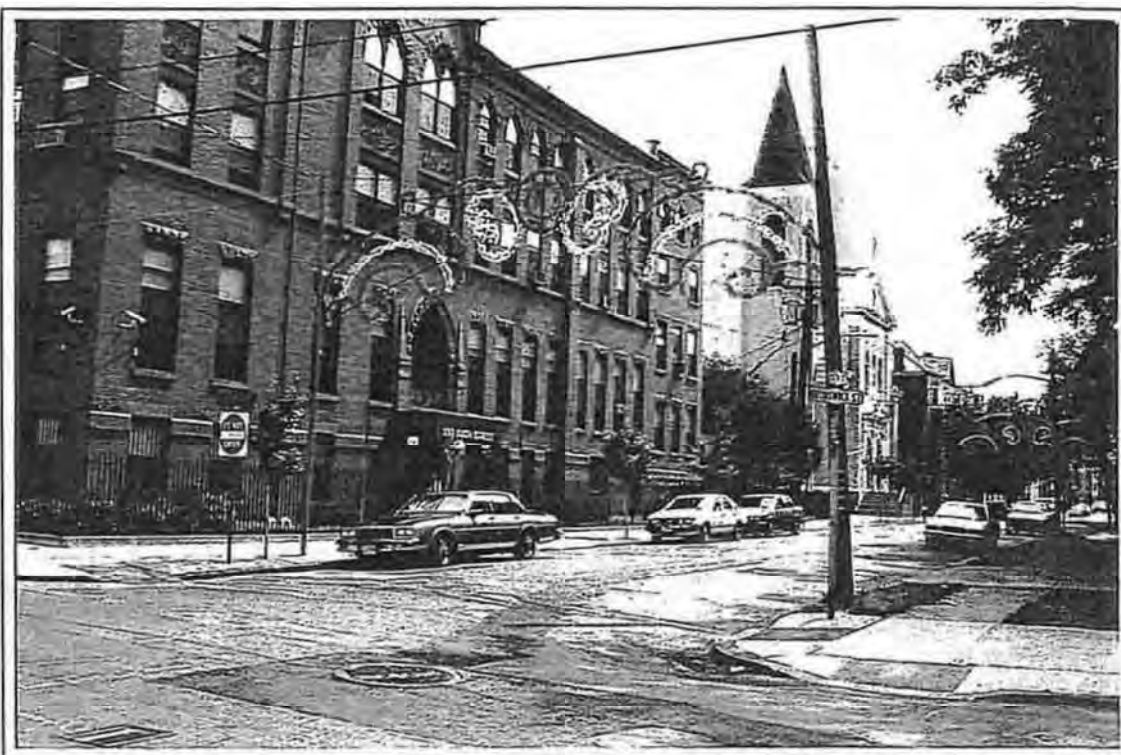
PLATE 9: Historic Church-related Buildings on Sixth Street, Looking East from Brunswick Street
